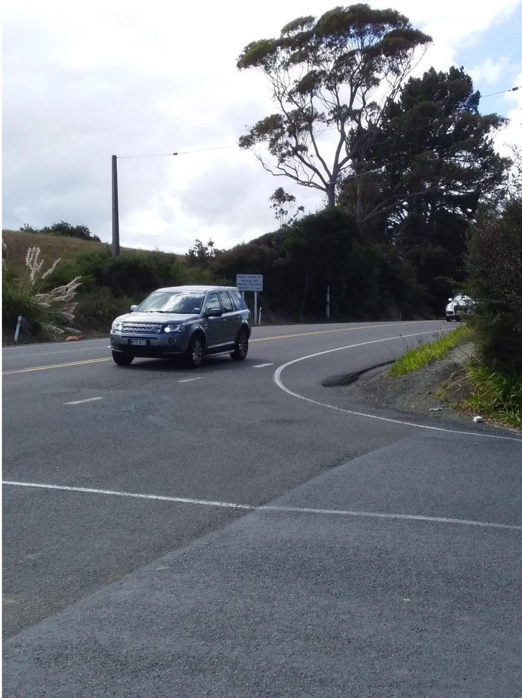
KcKinney /SH1 Lack of left turn lane, no footpath of kerbing and a substantial hole at the apex of the corner
