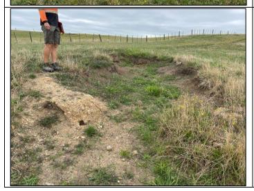
Photograph 2.7: Overland flowpath (as shown on Geomaps) up to 1m deep in NW paddock, originating from central part of paddock — landowner has advised novaflo drains from large Flats area discharge here, creating the scouring shown.
