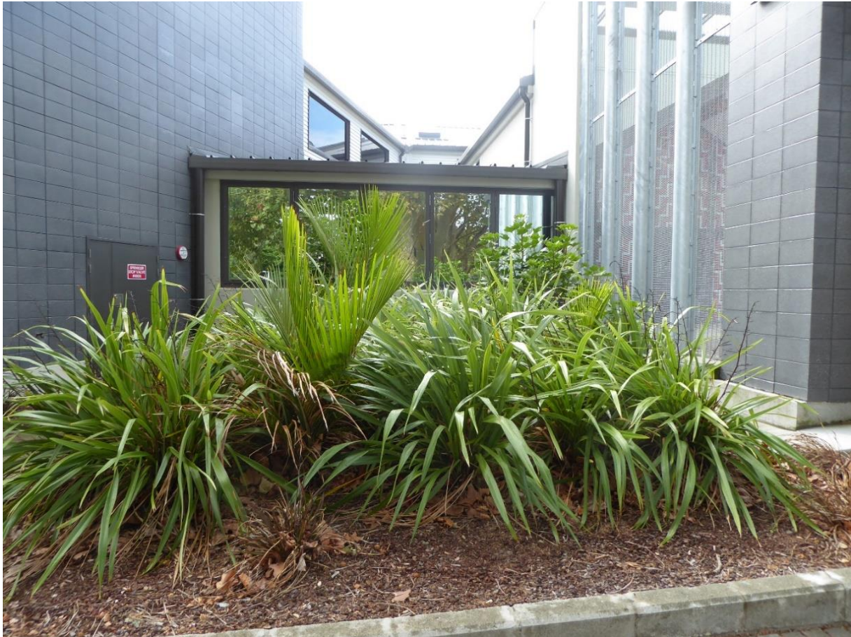
Figure M: East facing view of planting around the new Te Aka (T2) building on the southern side of the entry driveway
