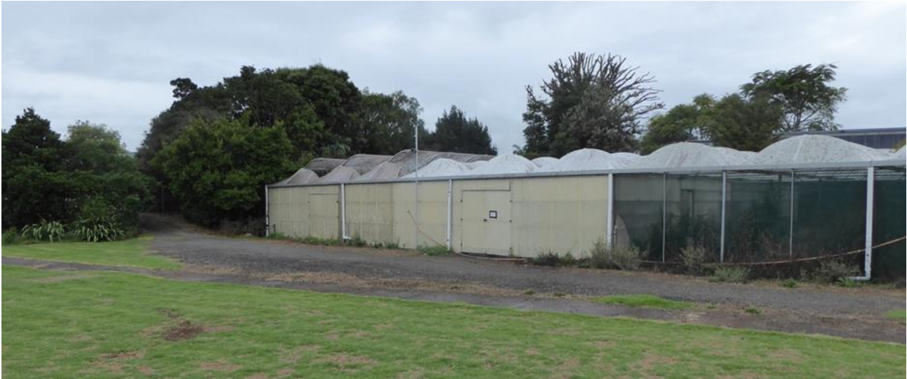
Figure P: Northeast facing view of the tunnel house complex on the Southern Site
