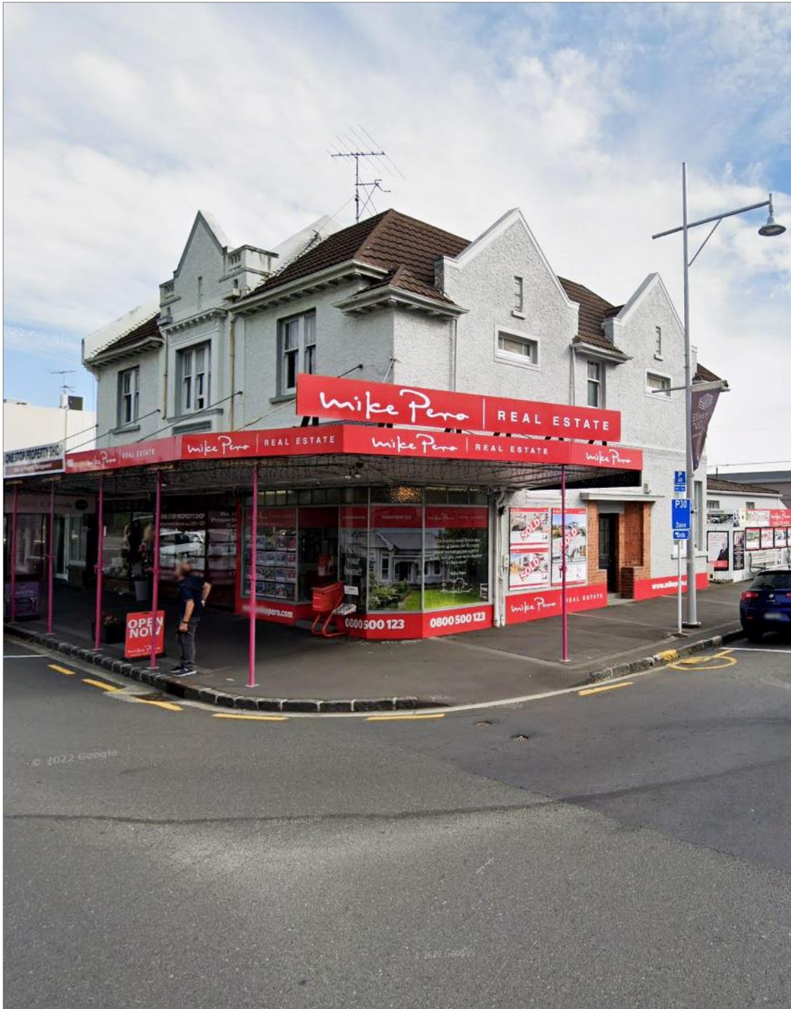
Figure 1: Mackenzie's Buildings. Google Maps, February 2021.
