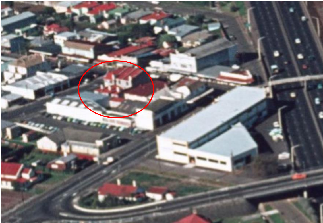
Figure 16: Mackenzie's Buildings in 1974. Shows what was likely the original corrugated iron roof. Auckland Council Libraries. Southern Motorway at Ellerslie, 1974. https://kura.aucklandlibraries.govt.nz/digital/collection/photos/id/89093
