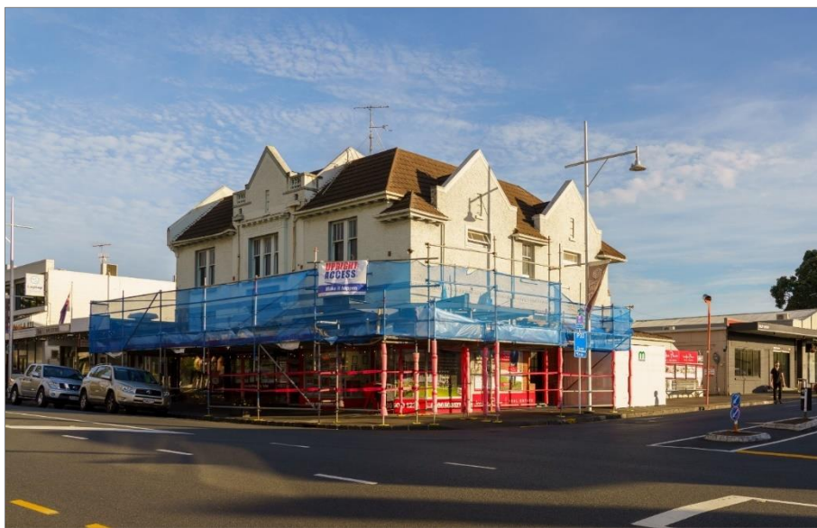
Figure 21 (top): The rear elevation of the building. Figure 22 (middle): East elevation of the building. Figure 23 (bottom): The corner elevation - the south and east elevations of the building. Blair Hastings, March 2022.
