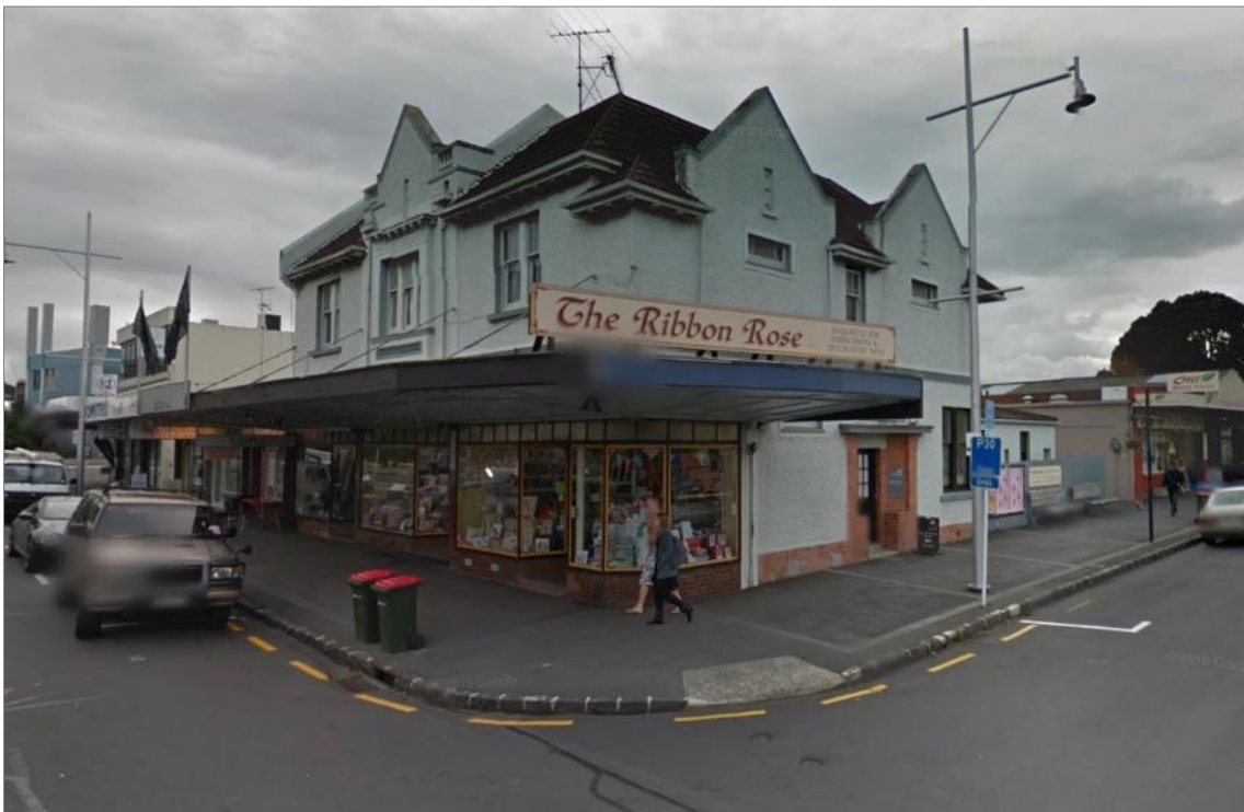
Figure 17: The buildings in May 2012. Included as it shows a better view of the ground floor elevations than can currently be seen due to the current construction works. Google Maps' Street View timeline feature. https://www.google.co.nz/maps
