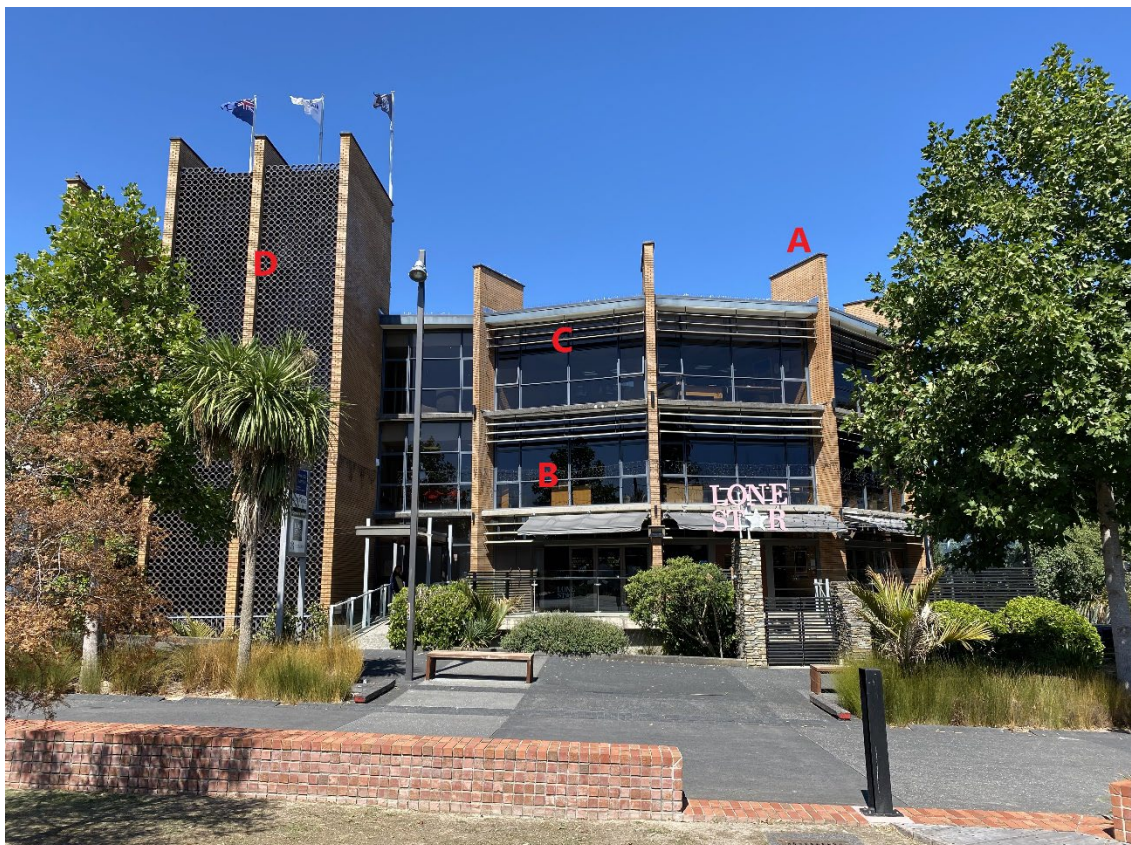
Figure 14. Annotated image showing the key features of the building: brick fins (A), glazed bays between fins (B), solar screens over the windows (C), and the stair/lift well with ceramic pipes (D). (David Bade, Auckland Council, 18/3/2020)
