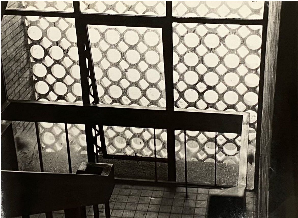
Figure 18. Interior of the building showing the ceramic screen and the carborundum floor tiles on the stairs (all products of the company). 75
