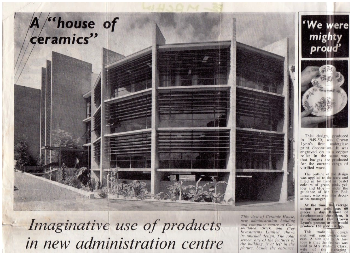
Figure 5. Newspaper clipping showing the completed building. 30
