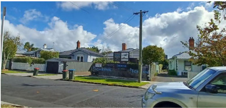
Figure 6: Chimneys in the Findlay Street streetscape (Auckland Council, March 2022)
