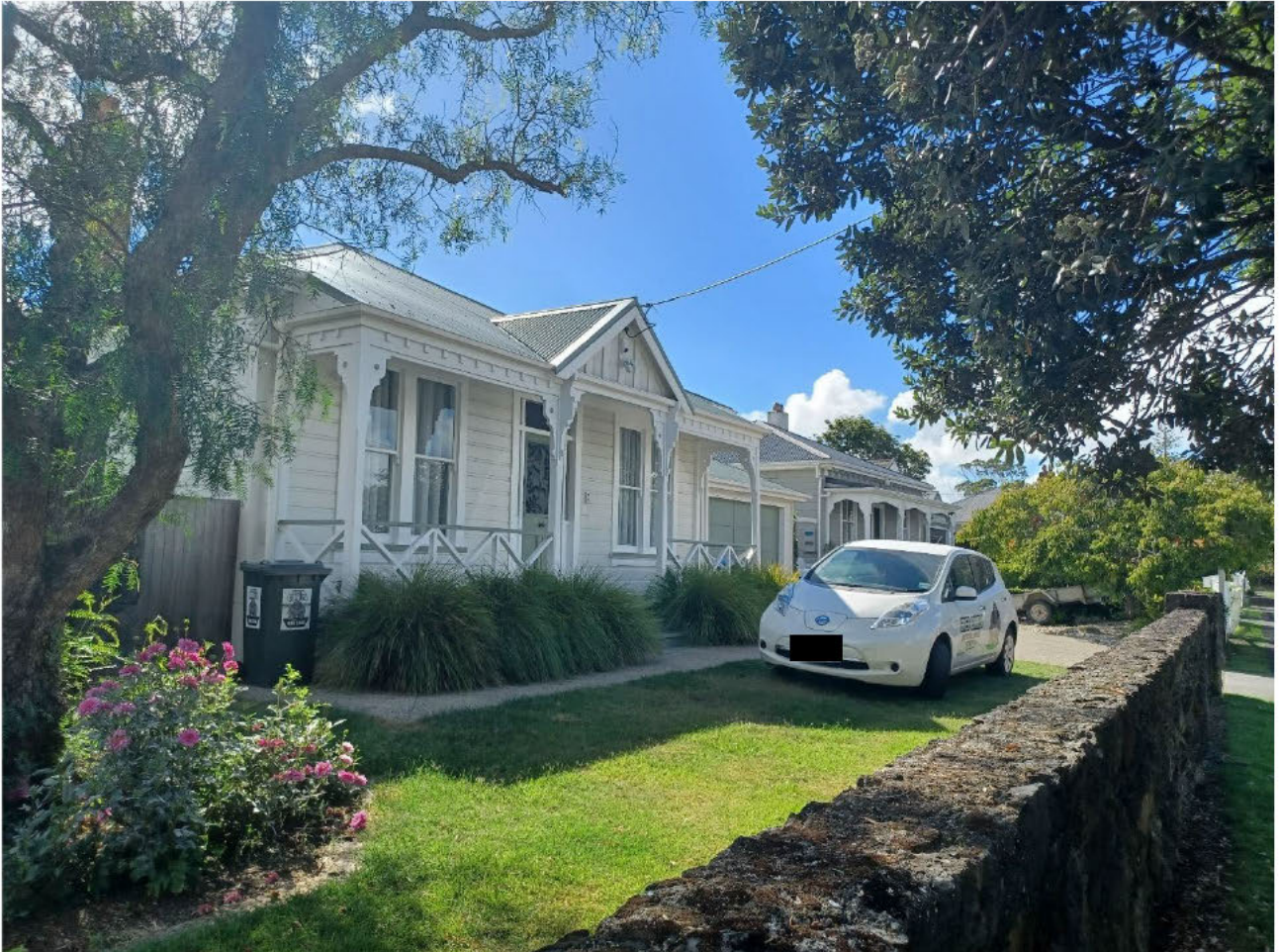
Figure 1: 11 and 9 Hewson Street, Ellerslie. (Auckland Council, March 2022)
