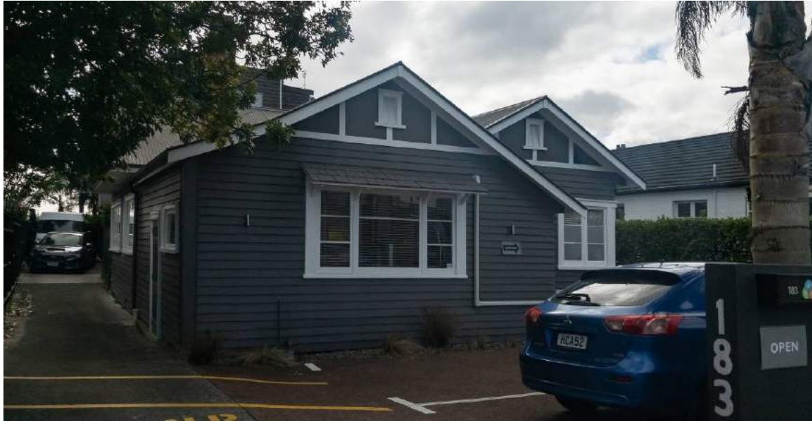
Figure 38: Showing the house at 183 Jervis Road. Source: Burgess Treep Knight 2019
