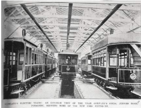
Figure 5: Showing the interior of Auckland Electric Tramways Company's sheds in Jervois Road 1902. Source: Auckland Libraries Heritage Collections AWNS-19020918-3-1
