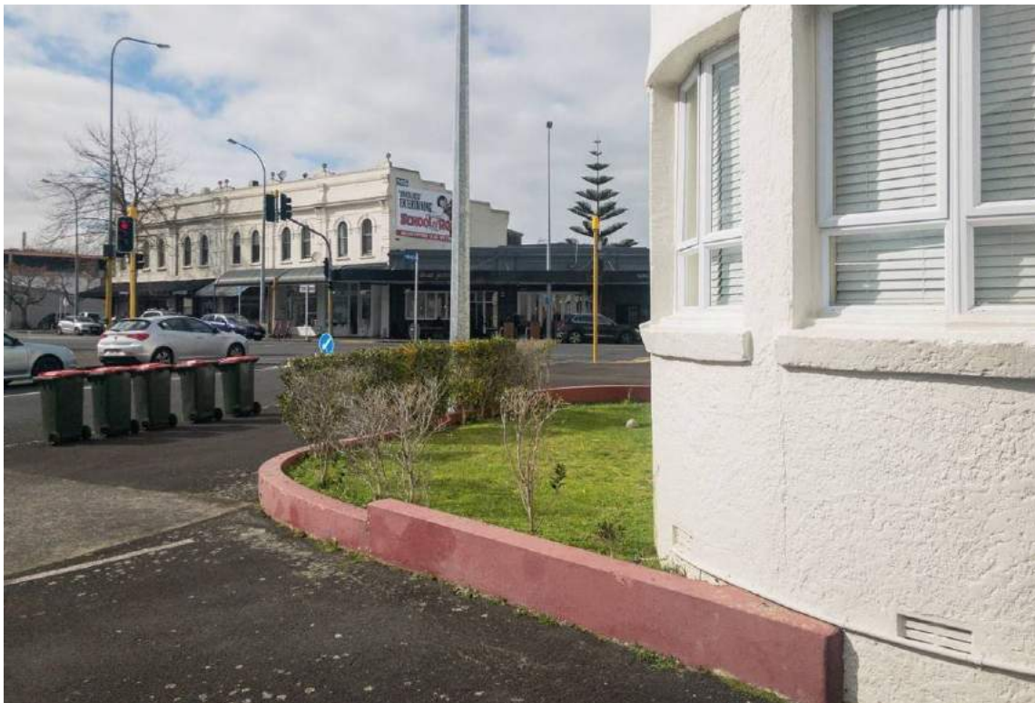
Figure 32: Looking south-east from the Raycourt driveway with the R & W Hellaby Building on the background. Source: Burgess Treep & Knight, 2019.
