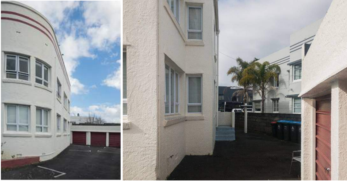
Figure 13: Rounded north eastern corner and garage at rear. Figure 14: Western side yard. Source: Burgess Treep & Knight, 2019.
