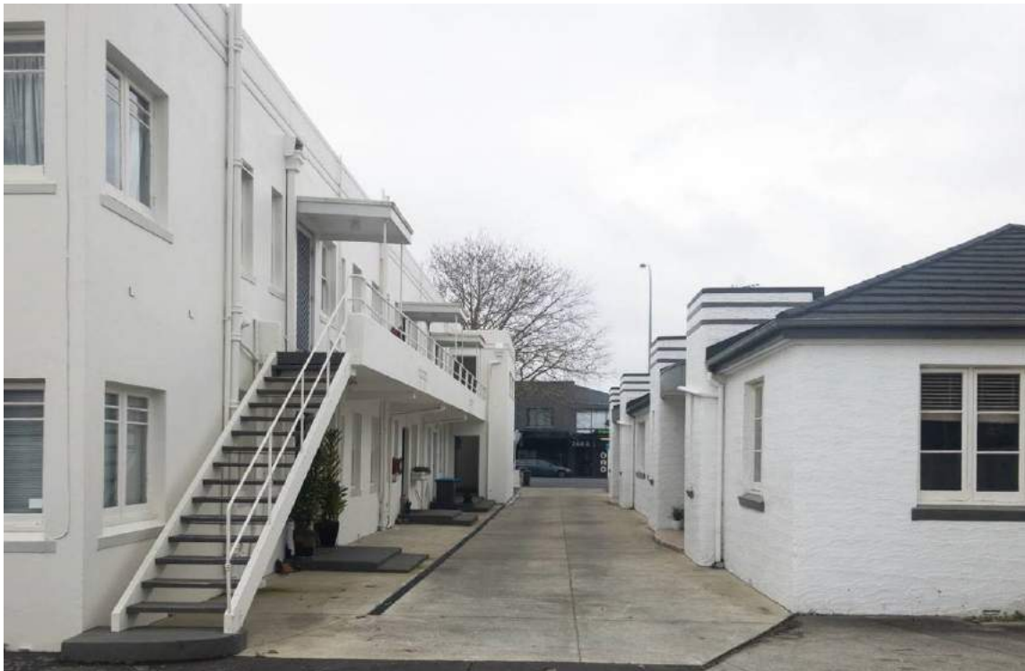
Figure 27: Looking south-east from the driveway in-between Kelmarna and Jervois Flats on the left and right respectively. Source: Burgess Treep & Knight, 2019
