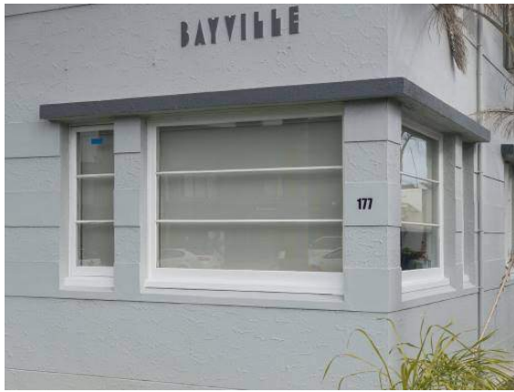
Figure 23: Original timber joinery. Figure 24: Bayville north-west corner (rear) elevation. Source: Burgess Treep & Knight, 2019.
