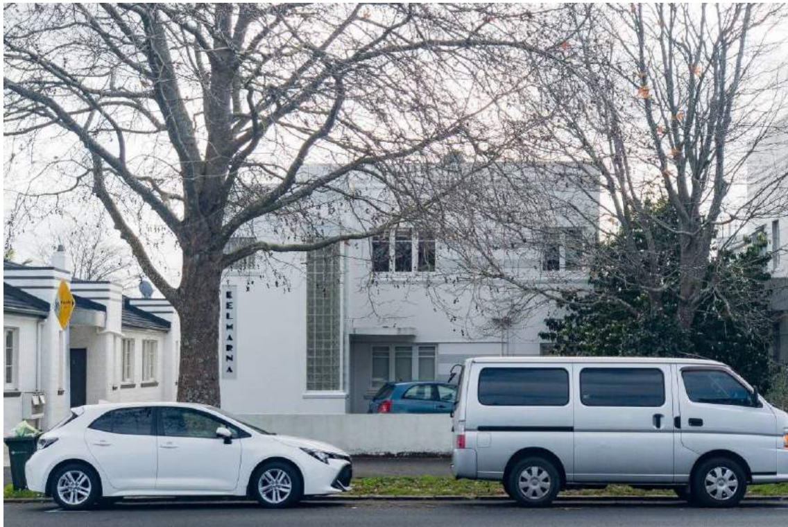
Figure 27: Kelmarna Flats, South (Jervois Road) Elevation
