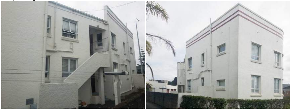
Figure 15: West (rear) elevation. Figure 16: south western corner. Source: Burgess Treep & Knight, 2019.
