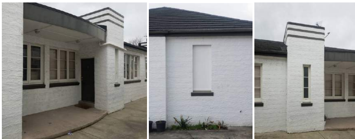
Figure 35: Jervois Flats north-east elevation showing windows and doors to apartments. Figure 36: Jervois Flats blocked-in window on the north-west (rear) elevation. Figure 37: Jervois Flats, vertical Streamline Moderne element with banded parapet. Source: Burgess Treep & Knight, 2019.
