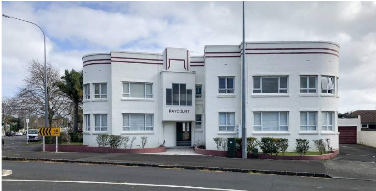
Figure 12: Raycourt Wallace St frontage. Source: Burgess Treep & Knight, 2019.
