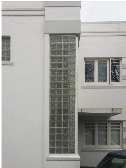
Figure 28: Vertical stack of glass bricks. Figure 29: glass bricks and plaster band detailing. Source: Burgess Treep & Knight, 2019.
