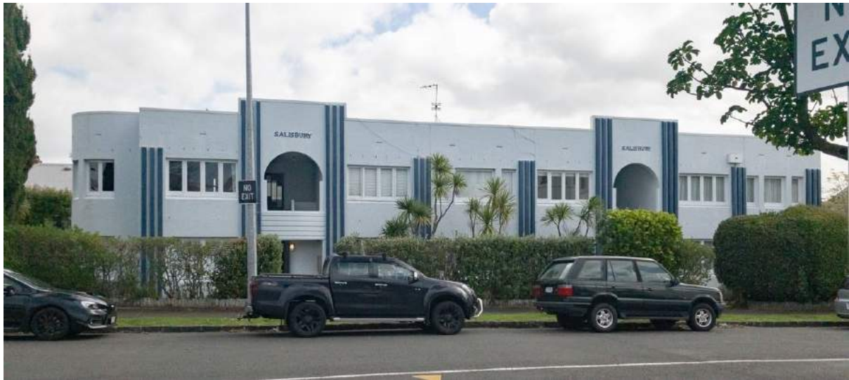
Figure 48: Salisbury St frontage. Source: Burgess Treep & Knight, 2019.
