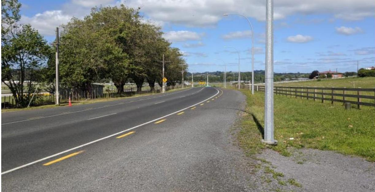
The available sight distance is over 230m in both directions and therefore exceeds the Austroads requirements.
