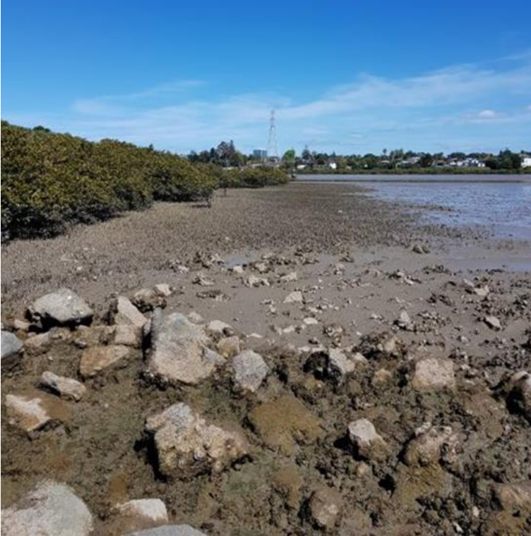
Figure 6: Slope and condition along the bank of Tamaki River estuary
