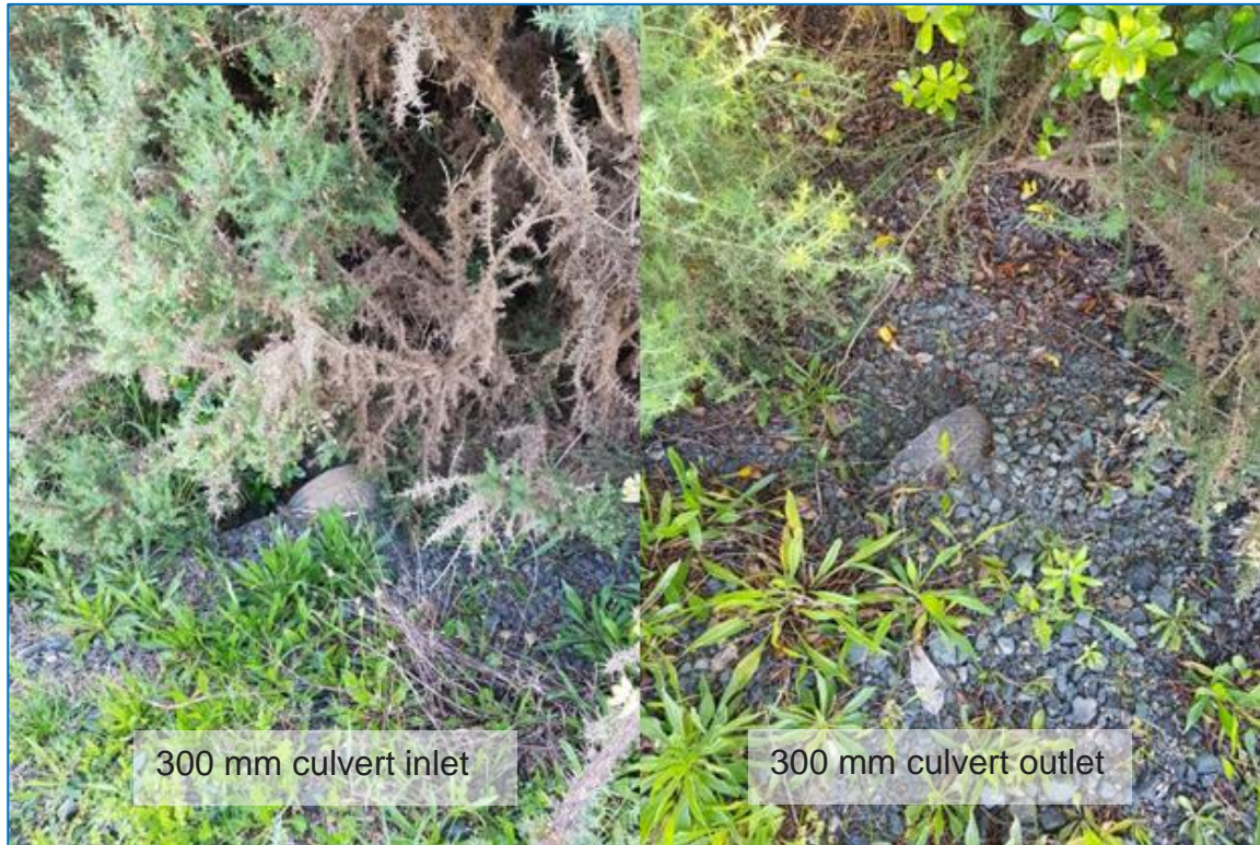
Figure 8: 300mm culvert across the internal gravel road
