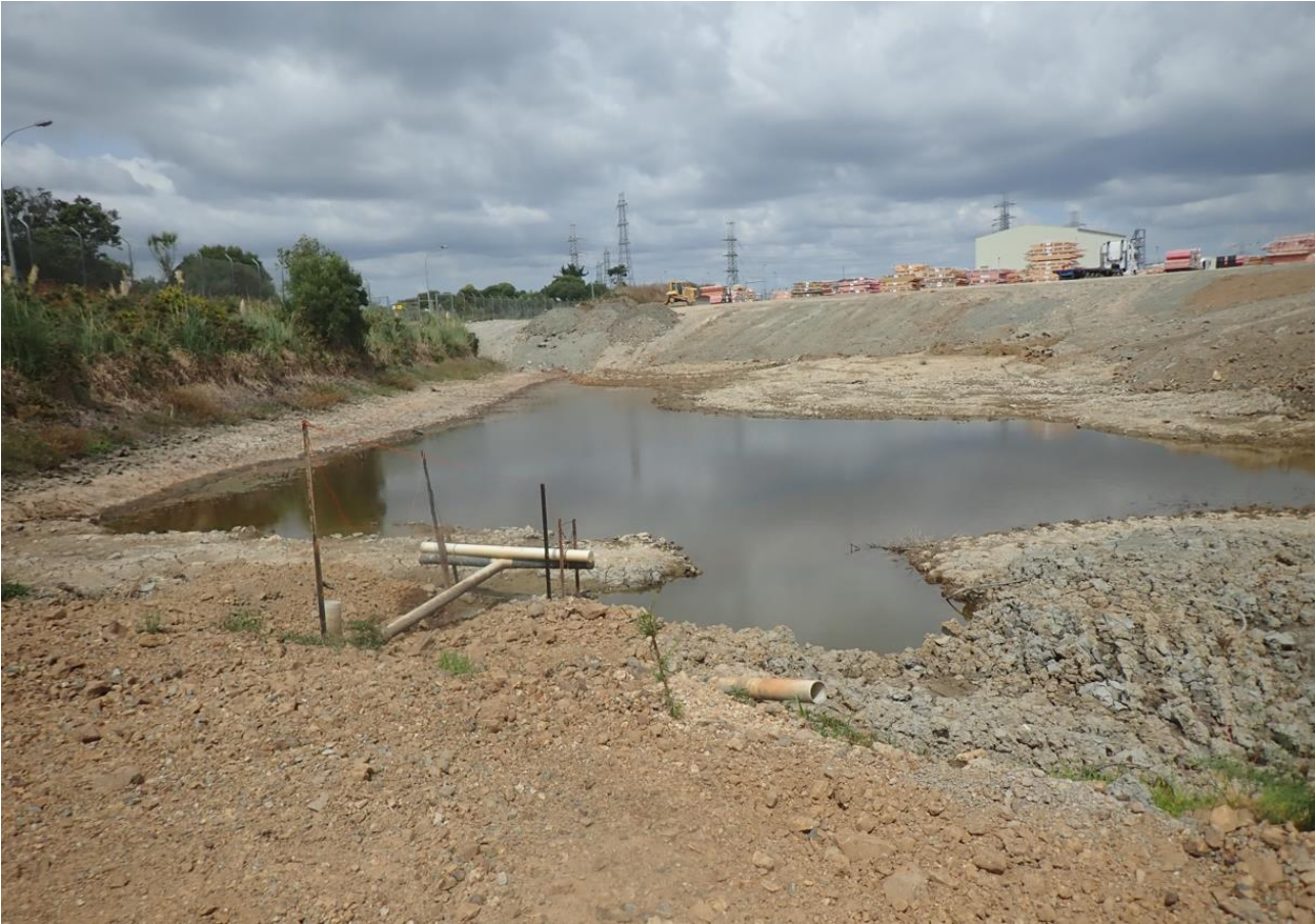
Figure 4: Remainder of the water cooling pond being used as a sediment control pond
