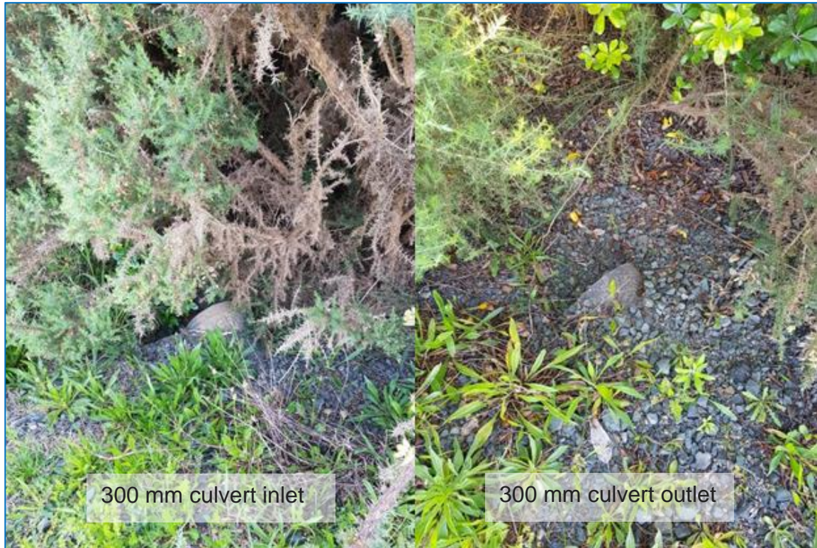
Figure 8: 300mm culvert across the internal gravel road
