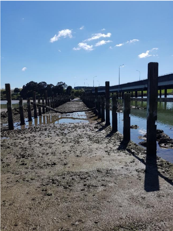
Figure 3: Existing Weir across Ōtara Creek
