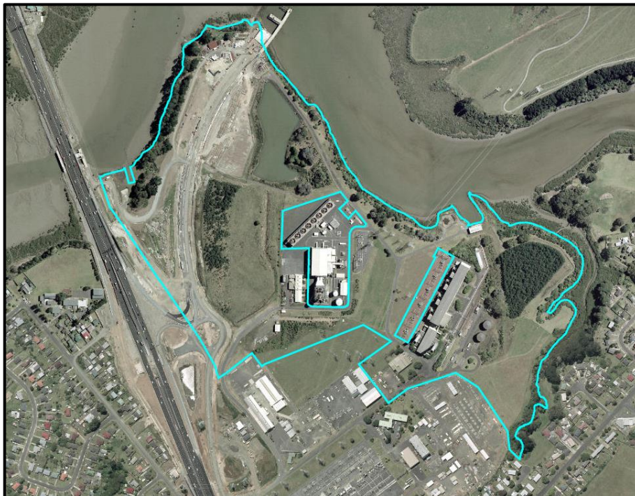
Figure 3-4: Construction of Highbrook Drive (Source: Auckland Council Geomaps Aerial Photography 2006)
