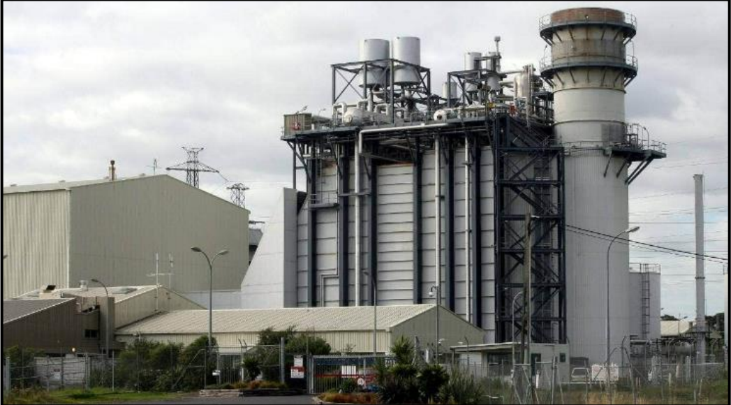
Figure 3-3: Photos of Ōtāhuhu Power Station
