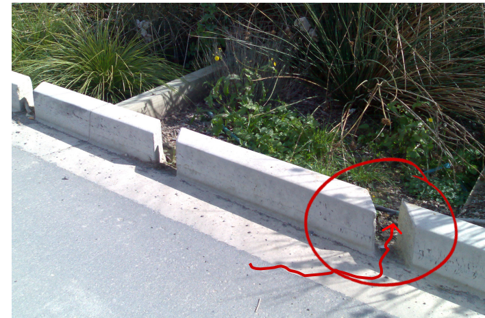
Incorporate on-site landscaping with storm water management. This example captures run-off from parking areas, channelling it to a rain garden via kerb cuts to filters before discharging to the piped system.
