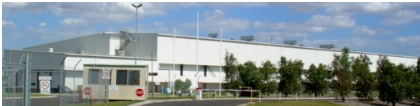
This large factory handles volatile materials and requires a climate controlled production floor (hence only very few windows and a plain 'shed' type design). It demonstrates an obvious security-controlled entry and the use of basic landscaping to screen the building's length.
