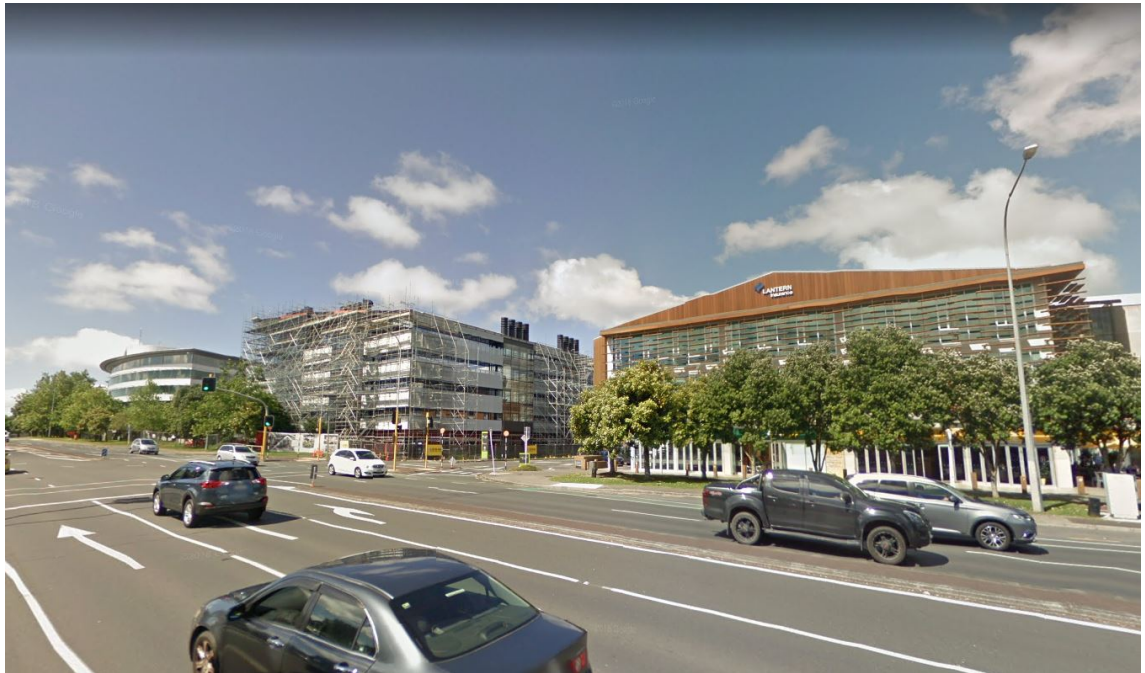
Figure 6: The scale of buildings along Taharoto Road has been gradually evolving over time from suburban residential to a more urban street corridor defined by medium rise buildings up to six storeys in height (Source: Google Street view).
