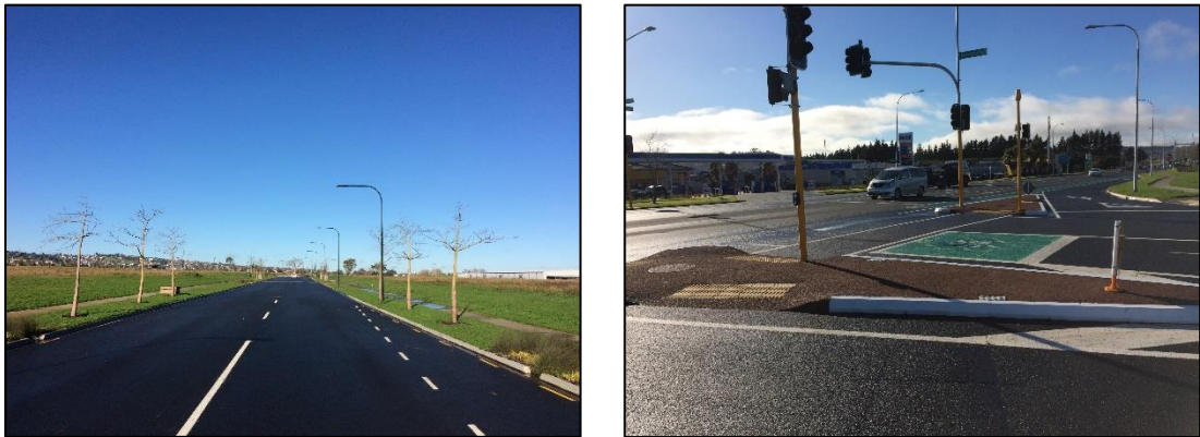
Figure 11 – Consented Development Infrastructure
