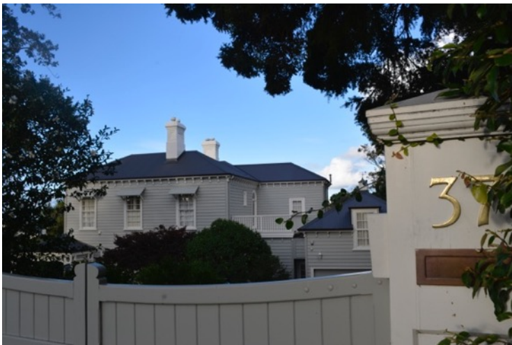
Figure 5: The west elevation and part south (rear) elevation of Glenholm, showing its central-gutter roof with prominent chimneys and first-floor double-hung sash windows (THS, 2018).
