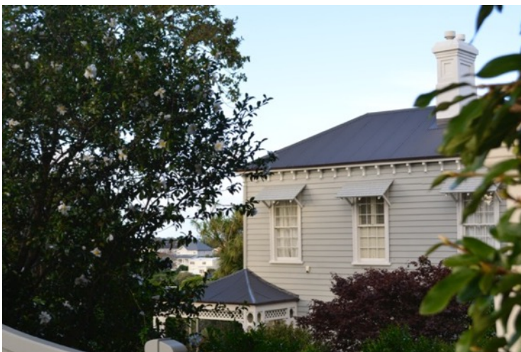
Figure 6: Part of the west elevation showing the first-floor double-hung sash windows and a portion of the wraparound verandah (THS, 2018).
