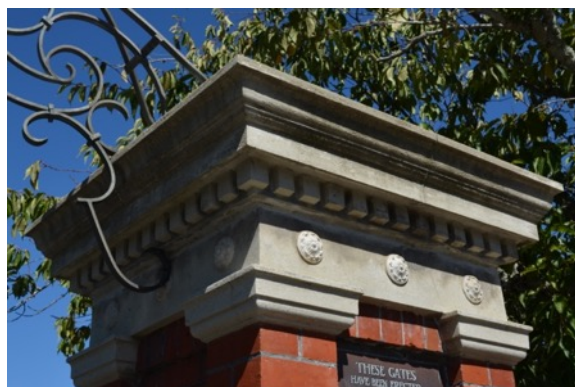
Figure 7: The decorative stonework on one of the principal pillars, comprising profiled cornice, dentil frieze and row of rosettes.
