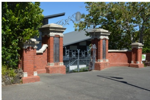
Figure 4: The War Memorial Gates viewed from Dromorne Road, comprising iron gates, brick pillars and walls decorated with Oamaru stone. Each principal pillar is inlaid with a dedication tablet.
