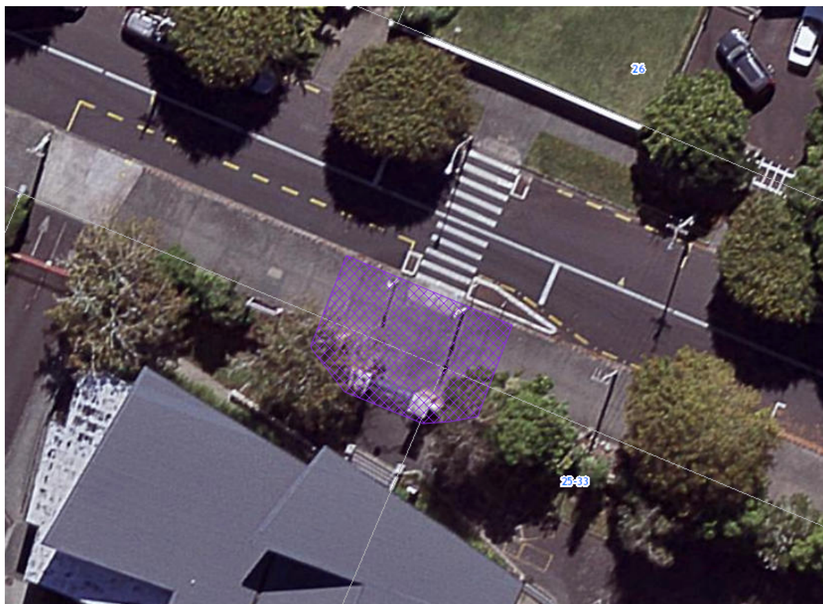
Figure 8: The extent of place of the War Memorial Gates is shown (purple hatch) and incorporates the structure itself and a portion of the Dromorne Road footpath directly in front of it. Given that portions of the memorial are not visible on the aerial, the extent has been drawn as closely as possible to the edge structure (Auckland Council GeoMaps).
