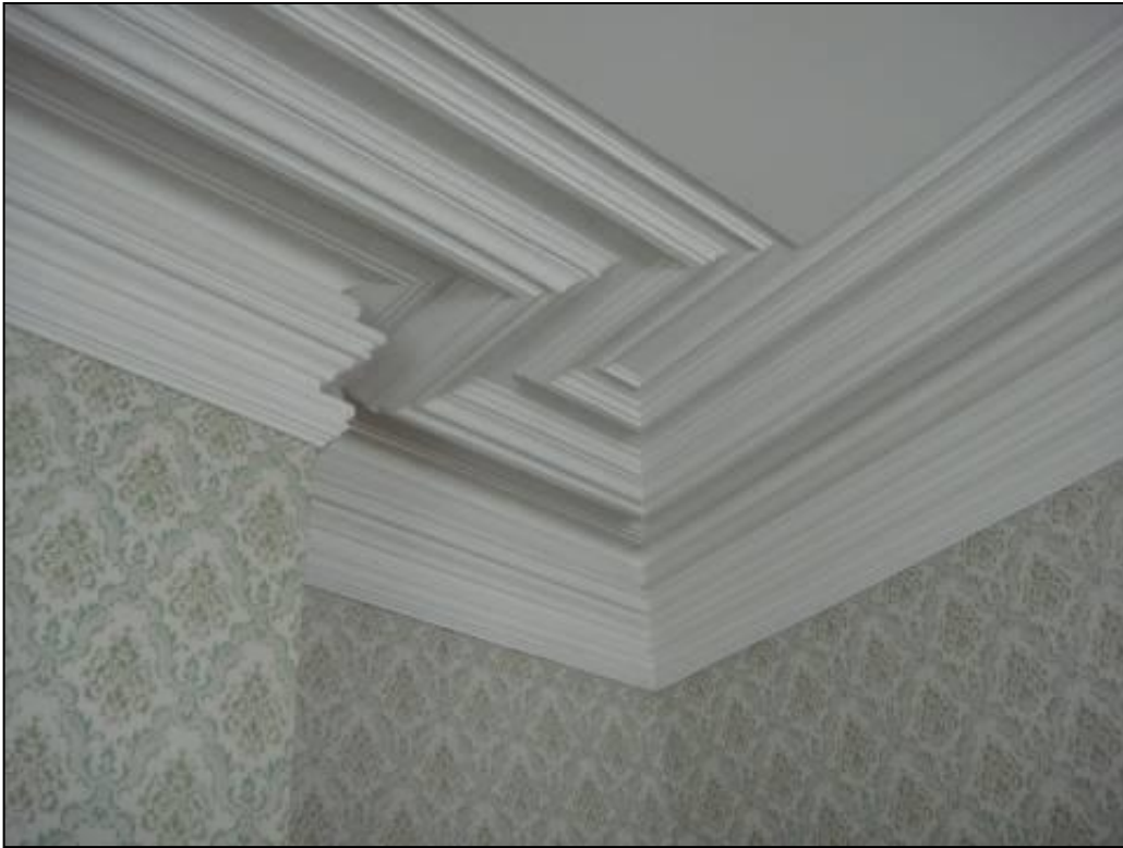
Figure 38. Cornice in west front room.
