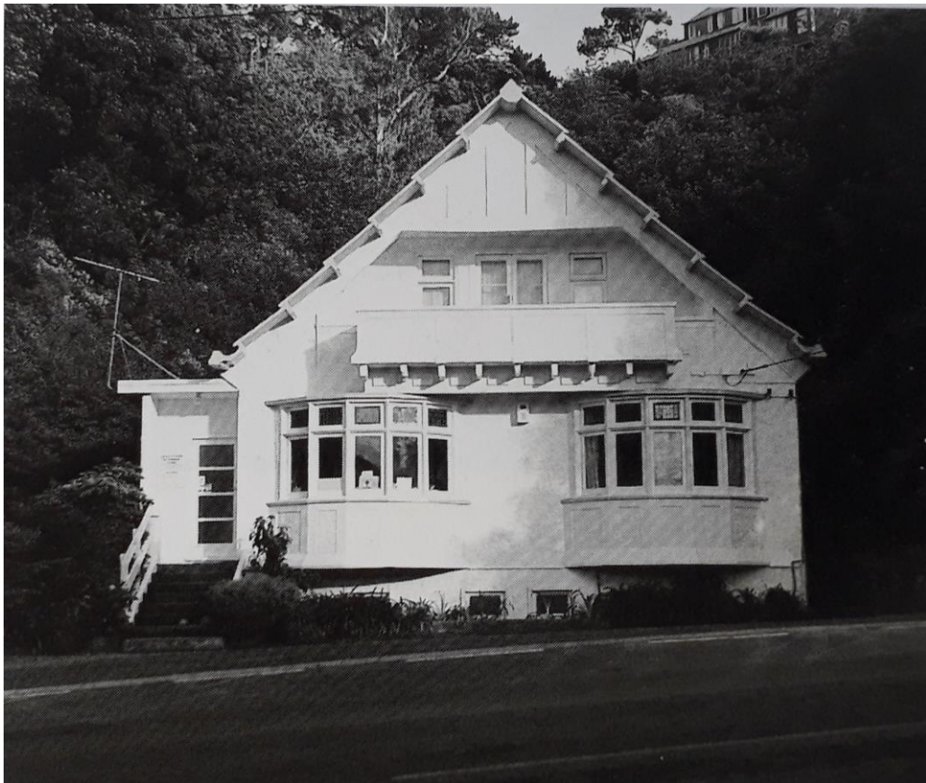
Figure 26. The English Cottage style all concrete house designed in 1918 by R W de Montalk. (Thornton).
