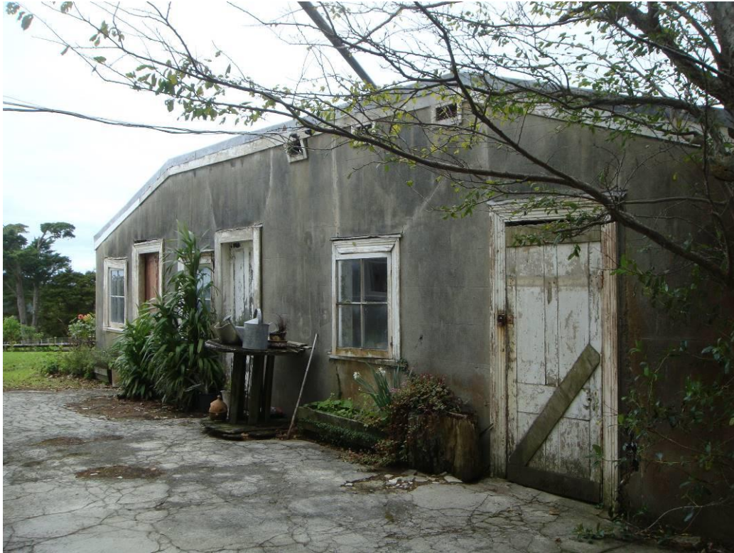
Figure 15. Ancillary building directly behind the house. (DPA Architects 2012).
