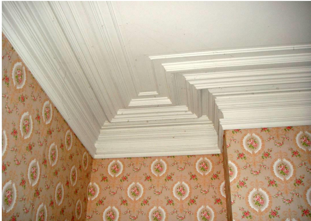
Figure 16. Plaster cornice on the interior in one of the ground floor front rooms (DPA Architects, 2012).
