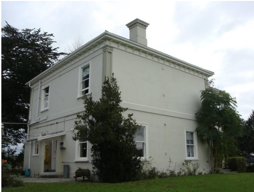
Figure 13. The eastern and southern elevations to the house (DPA Architects, 2012).
