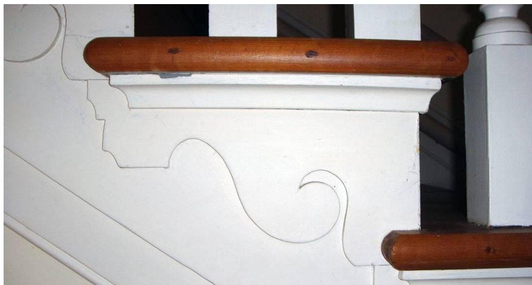
Figure 17. Elaborate carved detail along stringer of staircase (DPA Architects, 2012).
