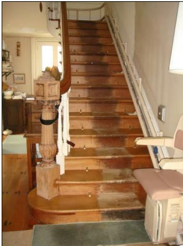
Figure 31. Staircase and elaborate newel post.
