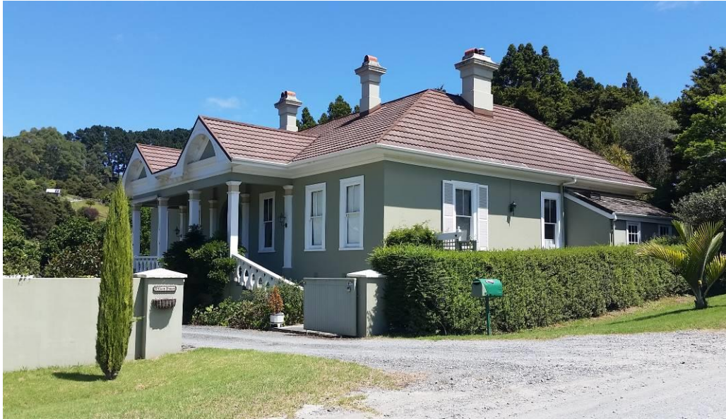
Figure 19 The former Managers House, which has been restored more recently. (Auckland Council, February 2019).
