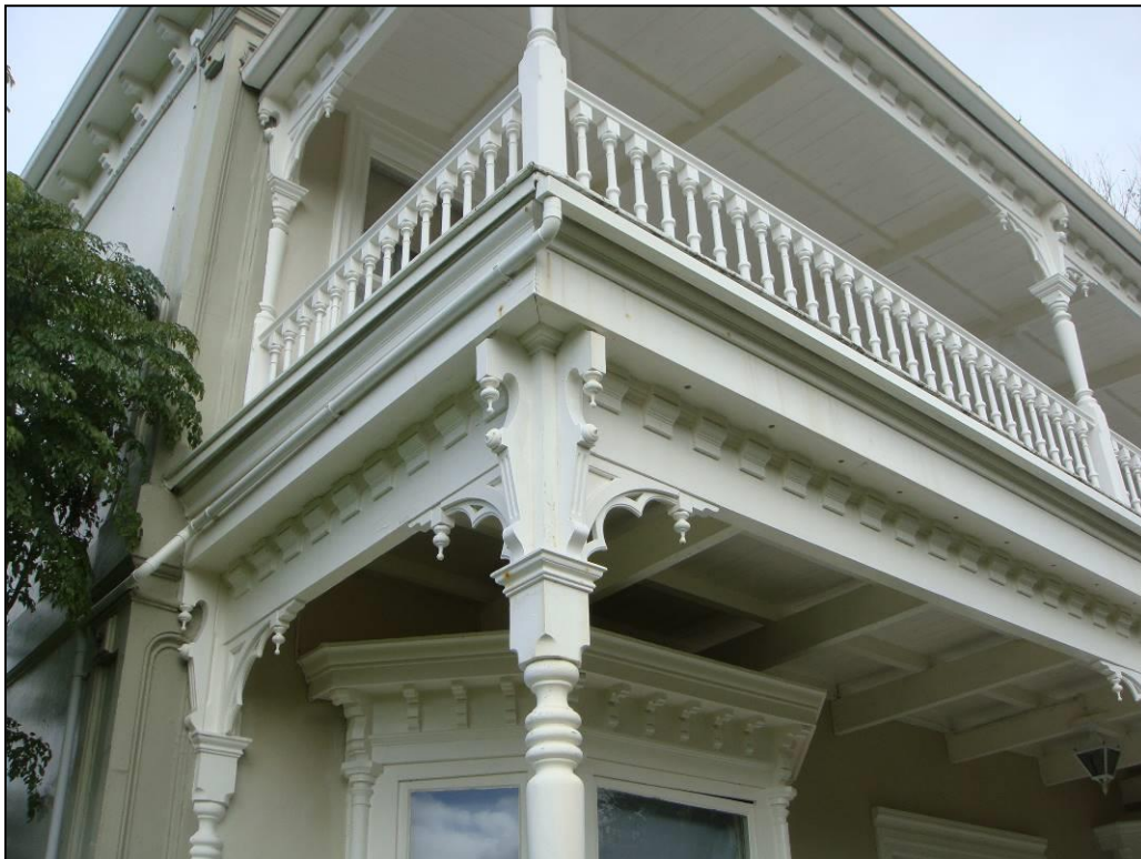
Figure 29. Details of verandah.
