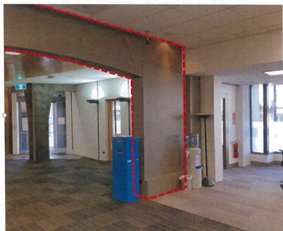
Photo 3 – Internalised external walls, looking east
