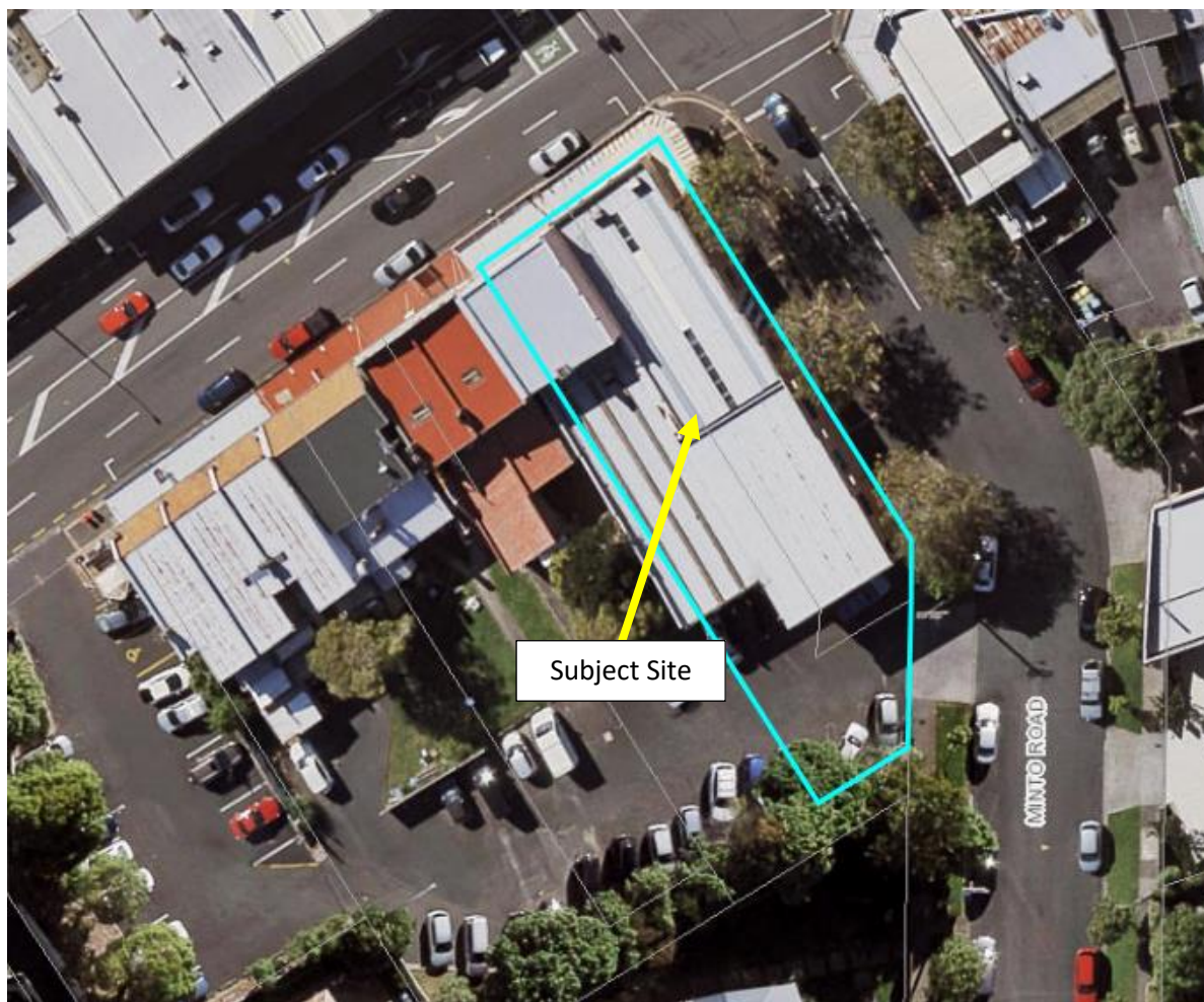
Figure 2: Aerial view of the subject site at 561 Remuera Road (Source: Auckland Council GeoMaps) (Note: The site boundaries shown on GeoMaps are not accurate relative to the positioning of the building and reference should be made to the CT).
