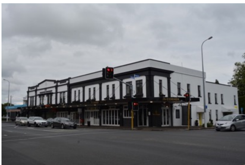
Figure 77: Looking northwest from the centre of Upland Village, showing the same group of two-storey buildings on the corner of Remuera and Upland roads.
