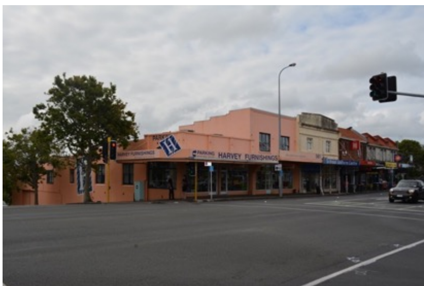
Figure 78: Looking southwest from the centre of Upland Village, showing the terrace of shop buildings on the corner of Remuera and Minto roads.
