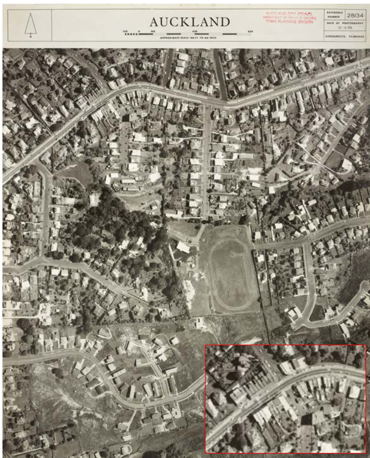
Figure 49: Aerial photograph of part of Remuera showing the Upland Village (top left, and close-up inset) in 1968. By this time, all but one of the buildings currently standing in the shopping centre were built (Sir George Grey Special Collections, Auckland Libraries, NZ Map 6960).
