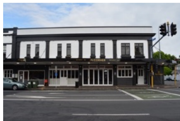
Brown Burcher & Letts Building, now The Corner
