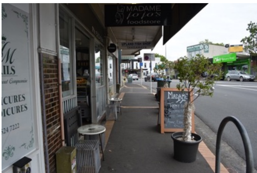
Figure 90: Looking roughly west along the footpath adjacent to 571-585 Remuera Road. Whilst shop fronts have been altered, some aspects of their configuration and features remain. Note the traditional glazed tiles to the left.
