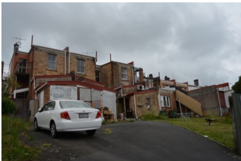
Figure 94: Largely unchanged rear elevations of the terrace of shops at 541-561 Remuera Road. A number of modest single-storey additions are visible.
