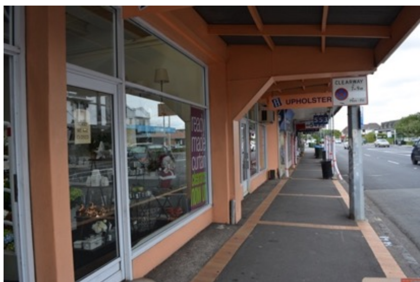
Figure 92: Looking roughly west along the footpath adjacent to the 541-561 Remuera Road.
