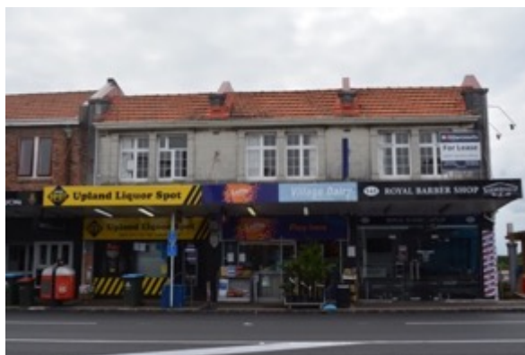
Figure 58: Hints of the Spanish Mission style is evident in the clay tile roof edged by gabled parapets. Detailing includes a series of pilasters that frame the first-floor windows.
