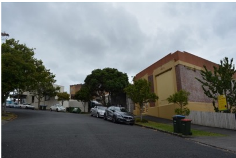
Figure 82: Looking roughly north along Minto Road as it rises to Remuera Road, showing the AEPB Remuera substation. Note the street trees along Minto Road.
