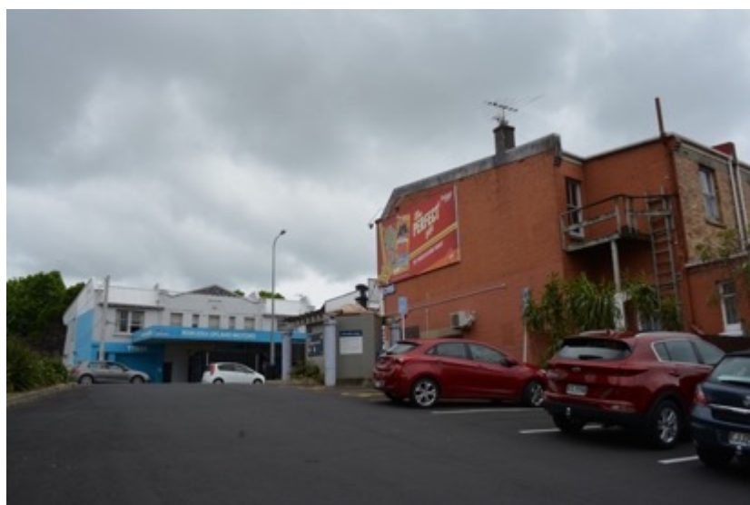
Figure 93: View looking north from the public carpark at 539 Remuera Road on the edge of the HHA, showing 541-545 Remuera Road (right), the public toilets (centre) and the garage at 586-592 Remuera Road (left).
