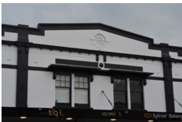
Figure 55: Showing the vertical and horizontal modulation of the building at 594-600 Remuera Road, emphasised by Stripped classical detailing such as a profiled parapet, cornices, plain modillions and pilasters. Other details include bracketed sun-hoods and plaster motifs.
