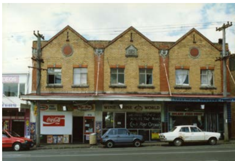
Figure 16: The 'Rayner 2' building at 579-565 Remuera Road in Upland Village during the 1980s. At this time the shops included a fish shop, liquor store and dairy (Shops, Remuera Road, Haresnape, William Raymond McDonald, 1921-1991, photographer, 1980s, PH-ALB-477-5-p73-2, Auckland Museum (untraced rights holder)).
