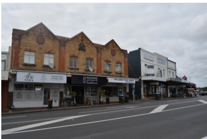
Figure 87: Two blocks of shops located in the southeastern portion of Remuera Village. The two-storey buildings, separated by an accessway, were constructed between 1923 and 1925.
