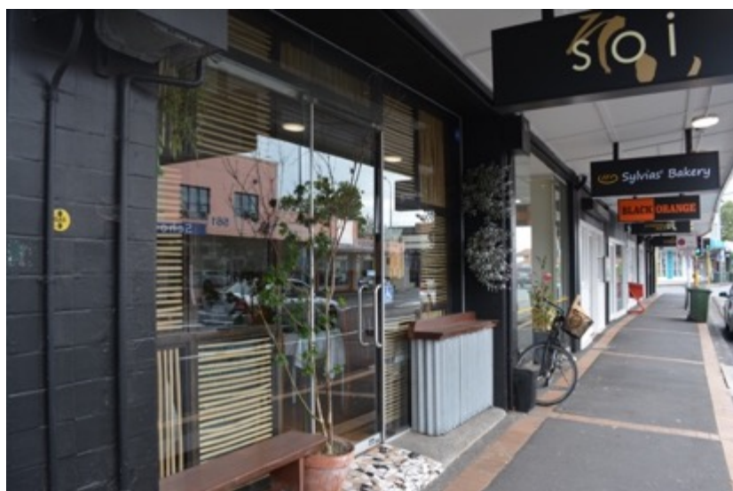
Figure 91: Looking roughly east along the footpath adjacent to 594-608 Remuera Road. Whilst the shop fronts have been replaced, attempts have been made to apply consistent signage under the verandahs.
