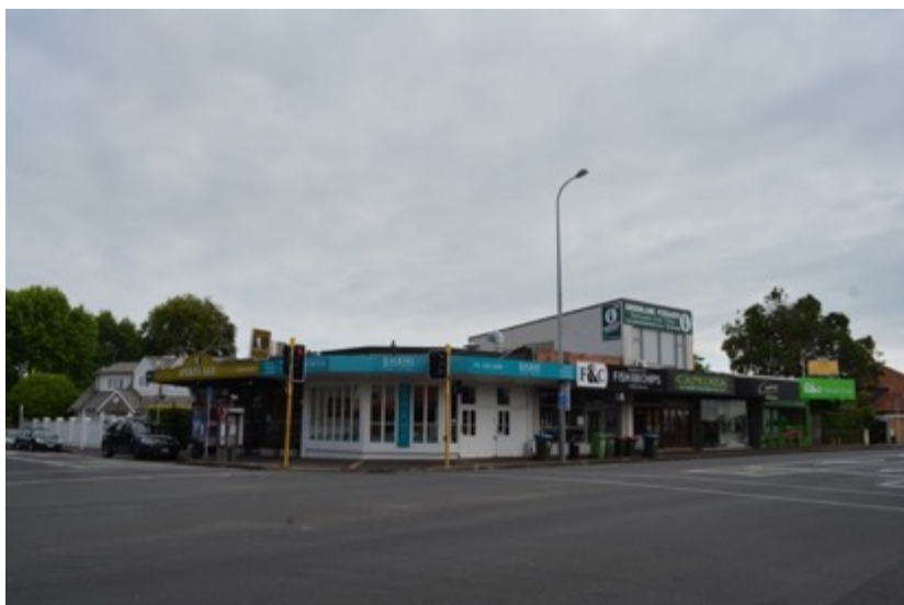
Figure 88: Looking northeast from the centre of Upland Village, showing the terrace of shop buildings on the corner of Remuera and Upland roads. These buildings were built between 1958 and 1961 and are situated outside the HHA.
