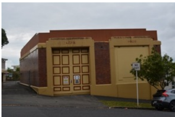
Figure 59: Although highly modified, the Art Deco/streamline moderne styling of the Remuera substation building is still apparent in its defined outlines, curvilinear and geometric detailing.
