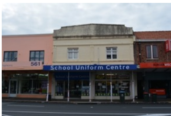
Figure 56: Stripped classical detailing on the building at 551-553 Remuera Road includes a profiled parapet, pilasters, cornice and decorative plaster discs.
