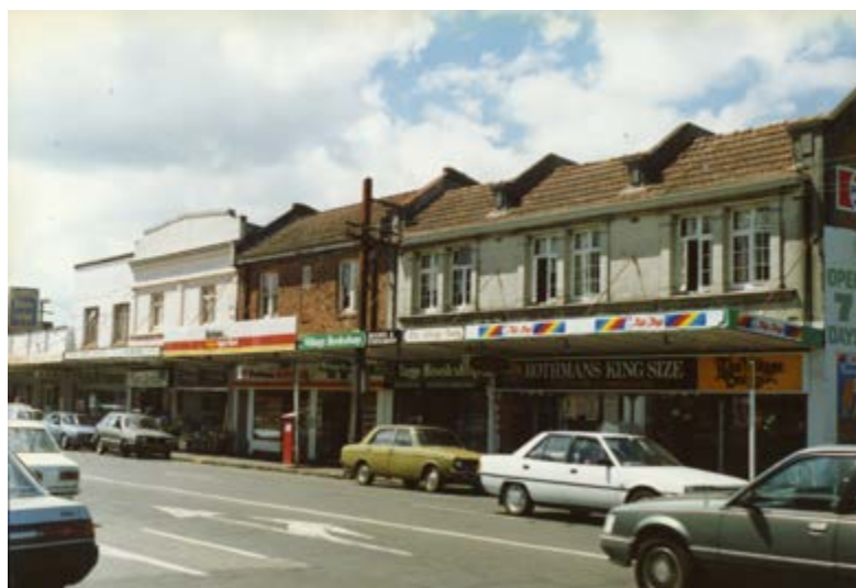
Figure 14: View of the southwestern group of shops (545-561 Remuera Road) in Upland Village during the 1980s. At this time the shops included Beltons United Realty World, Village Bookshop and the Village Diary (Shops, Remuera Road, Haresnape, William Raymond McDonald, 1921-1991, photographer, 1980s, PH-ALB-477-5-p74-3, Auckland Museum (untraced rights holder)).
