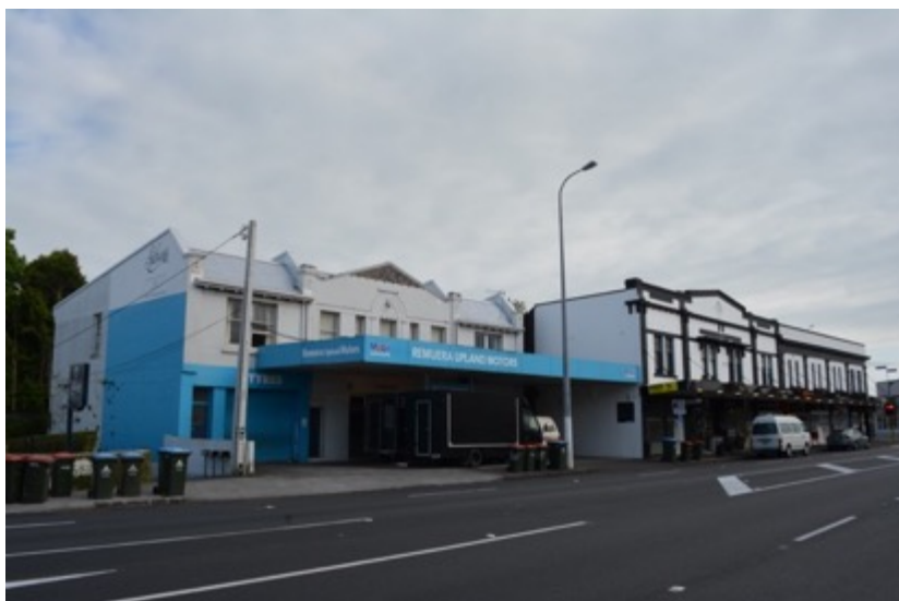
Figure 76: Looking northeast from the western edge of Upland Village, showing the distinctive group of two-storey buildings. The two blocks of residential shops and former service station were built between 1923 and 1926.
