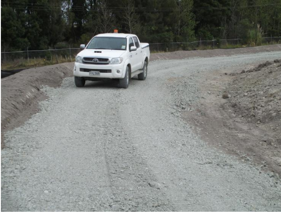
Figure: Stabilised haul route
