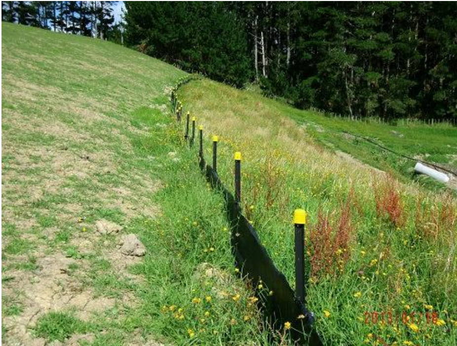
Figure: Silt fence
