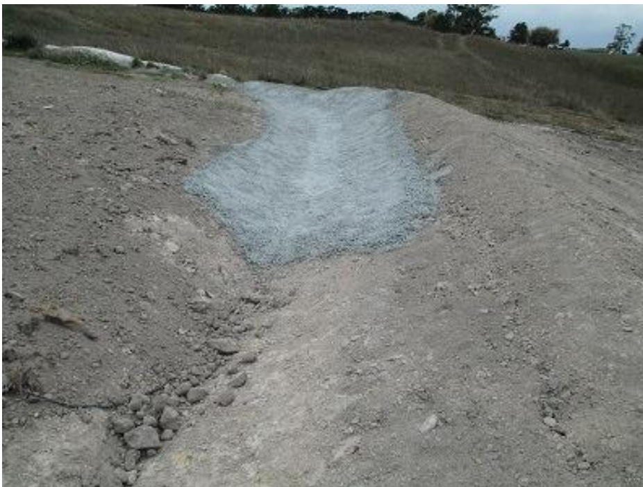
Figure: Lined dirty water diversion on intermediate cover
