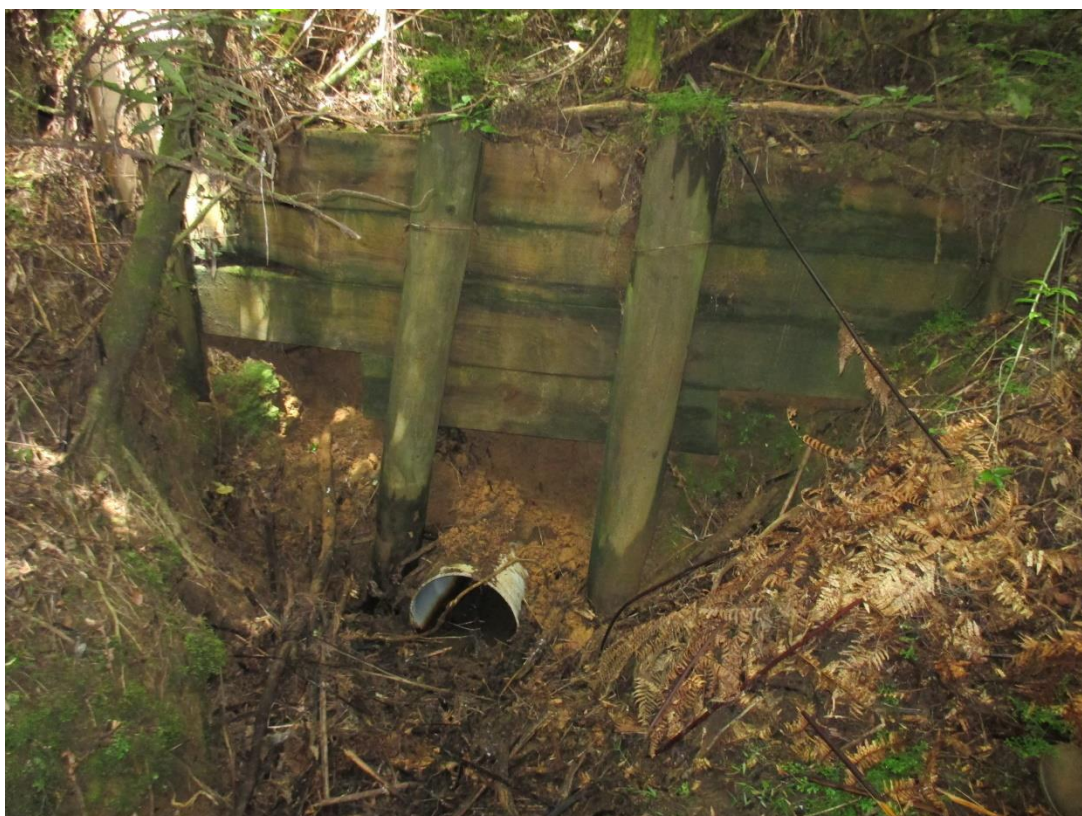
Figure 15.2: Existing stream crossing at proposed embankment location
