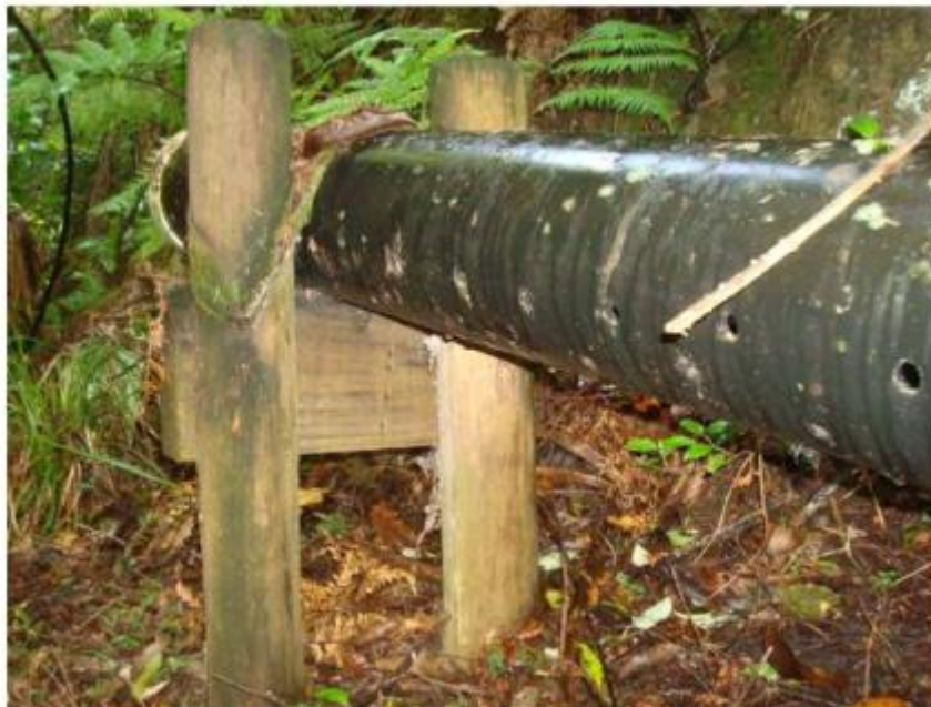
Figure 7: Dispersal Bar with Suitable Supporting Structure and Outlet Holes
