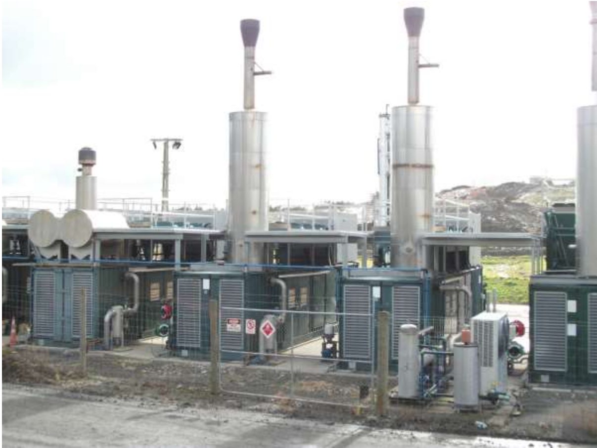
Photograph 3.2: Generators at Redvale Landfill
