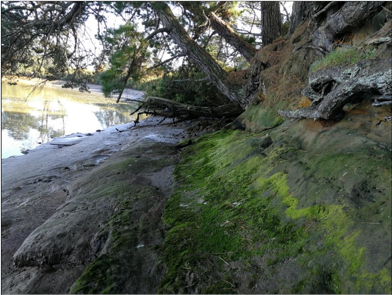
Figure 3: Waitemata Series toe material from the norther section of cliff at the subject site. (Source: Site visit)
