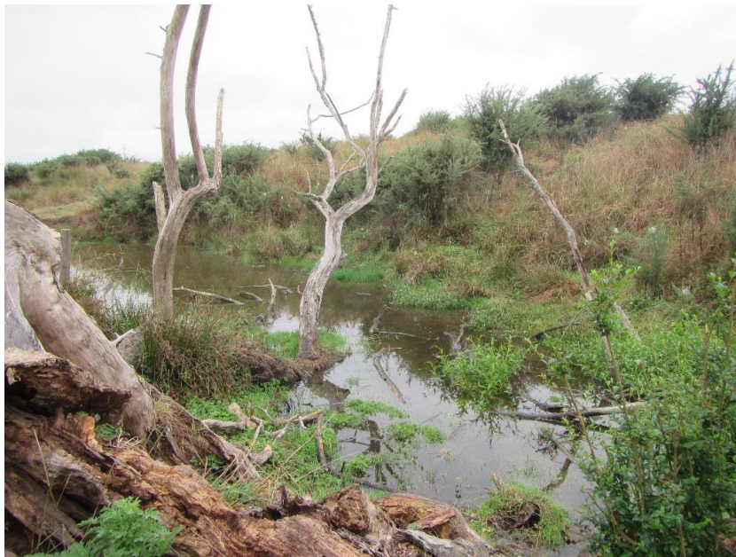
Plate 17: Pond at downstream end of watercourse, looking toward damaged crossing. 19 March 2019.
