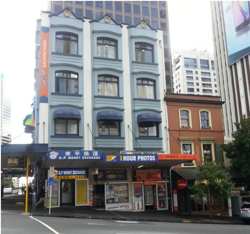
Figure 6. The north-east elevation fronting Victoria Street West (Auckland Council, 24/3/2015)
