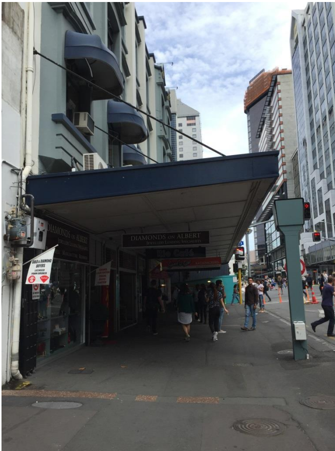
The veranda over the footpath on Albert Street.
