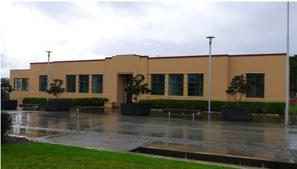
Figure 1: RNZAF Headquarters (5 July 2017; Auckland Council)
