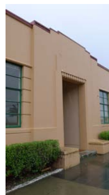
Figure 5: Stepped parapet (5 July 2017; Auckland Council)
