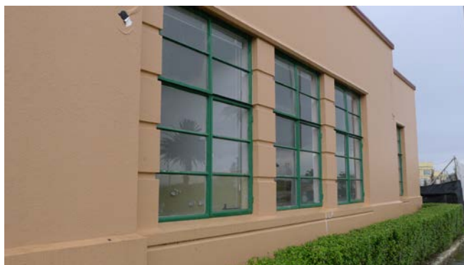
Figure 10: Windows front facade (5 July 2017; Auckland Council)
