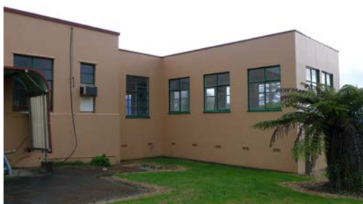
Figure 16: Southern elevation of the 1953 extension (5 July 2017, Auckland Council)
