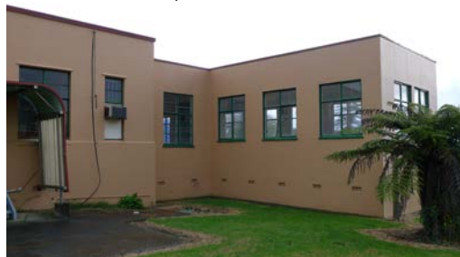
Figure 15: Eastern (rear) elevation showing the 1953 extension (5 July 2017; Auckland Council)
