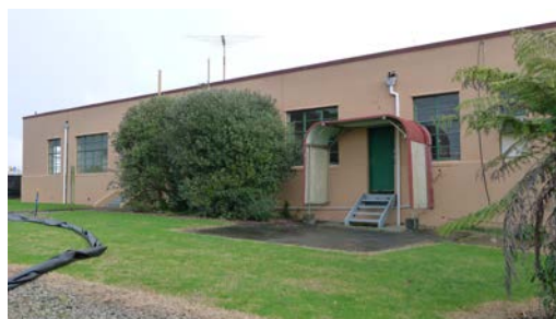
Figure 13: Eastern (rear) elevation (5 July 2017; Auckland Council)
