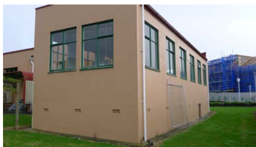
Figure 17: Eastern and northern elevations of the 1953 extension (5 July 2017; Auckland Council)
