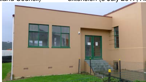
Figure 18: Western elevation of the 1953 extension (5 July 2017; Auckland Council)
