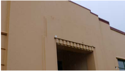
Figure 6: Plaster detailing around entry porch (5 July 2017); Auckland Council)
