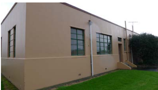
Figure 12: Eastern (rear) elevation (5 July 2017; Auckland Council)
