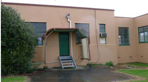
Figure 14: Eastern (rear) elevation (5 July 2017; Auckland Council)
