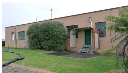
Figure 20: Bush and palm tree along the rear elevation (5 July 2017; Auckland Council)
