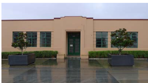
Figure 19: Hedge and magnolia trees along the front facade (5 July 2017; Auckland Council)
