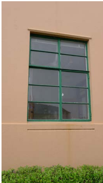
Figure 8: Stringcourse under windows (5 July 2017; Auckland Council)
