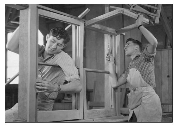
Figure 47: Standard window joinery for state houses made off site (Alexander Turnbull Library PAColl-4161-01-207-10).
