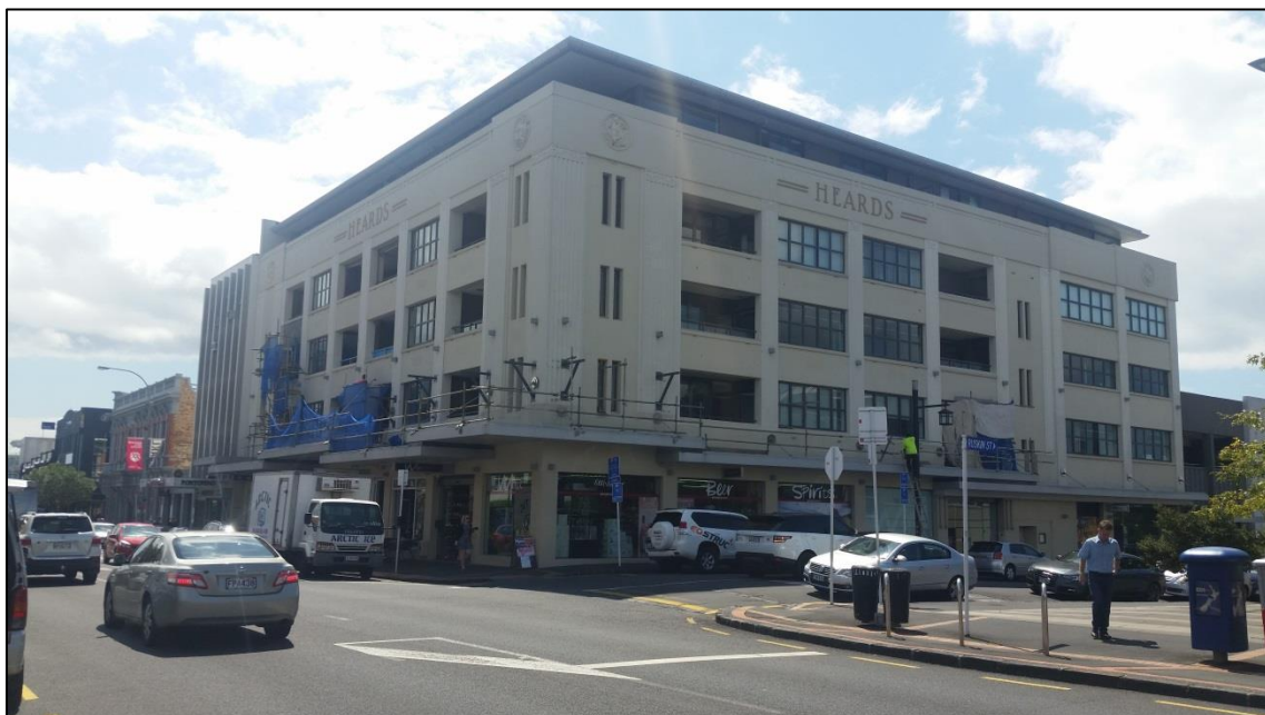
Figure 15: The former Heard's factory in Parnell Road as it is now. This building has been adaptively reused as apartments and offices above retail spaces. (Auckland Council February 2017).
