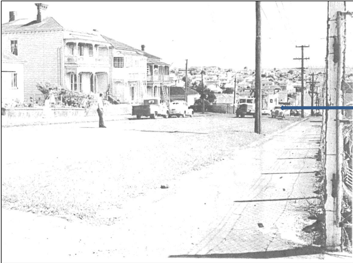
Image taken of Crummer Road taken from near Ponsonby Road in 1965. The arrow points to the Murray shoe factory which was still operating out of the building. (Auckland Council Property Files)
