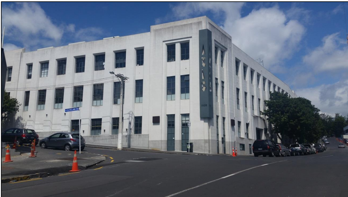
Figure13: The Axis Building (former Nestle Factory) in St Georges Bay Road. (Auckland Council, February 2017).
