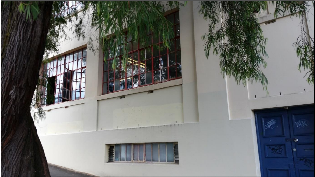
Crummer Road façade showing panelled window bays, an original entry door and how the south western side of the building is concealed by later development.
