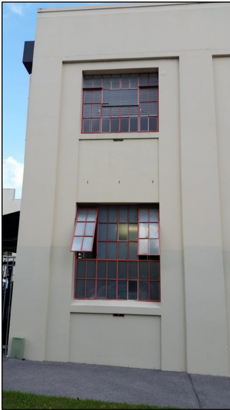
Original steel windows of building and decorative panelling effect of façade framing the window bays.
