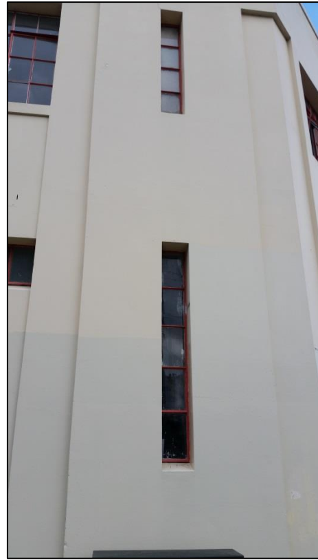
Original steel windows of building and decorative panelling effect of façade framing the window bays.
