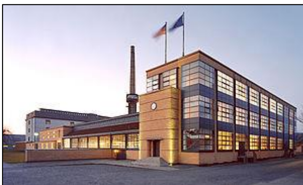
Figure 9: Fagus Shoe Last Factory in Germany, built between 1911 and 1913, https://en.wikipedia.org/wiki/Fagus_Factory accessed 1 November 2016).
