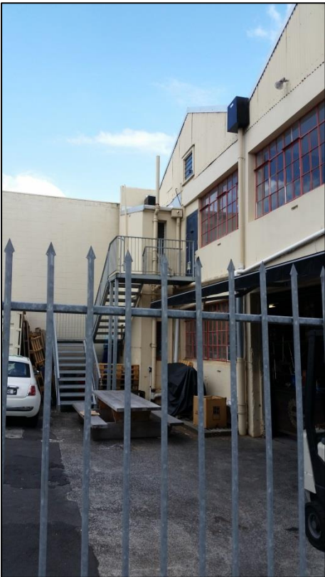
The rear of the building, shows many original features, including the twin gabled roof form and the steel framed windows. The staircase was added later.
