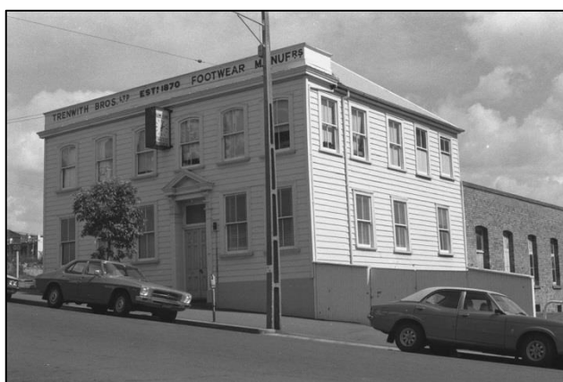
The Trenwith Brothers footwear factory in the 1970s. More window openings have been added to the side walls to let more light into the building. (Sir George Grey Special Collections, Auckland Libraries, 314-10-31).
