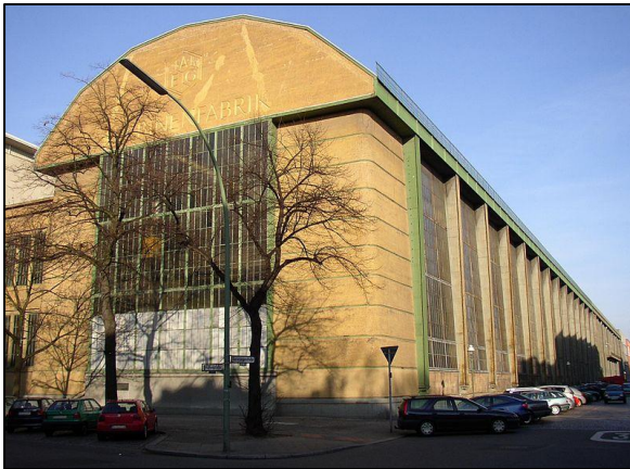
Figure 8: The AEG turbine factory completed in 1909 in Berlin demonstrating the large amount of glazing in a concrete and steel building. https://en.wikipedia.org/wiki/AEG_turbine_factory accessed 28 November 2016 (accessed 28 November 2016).
