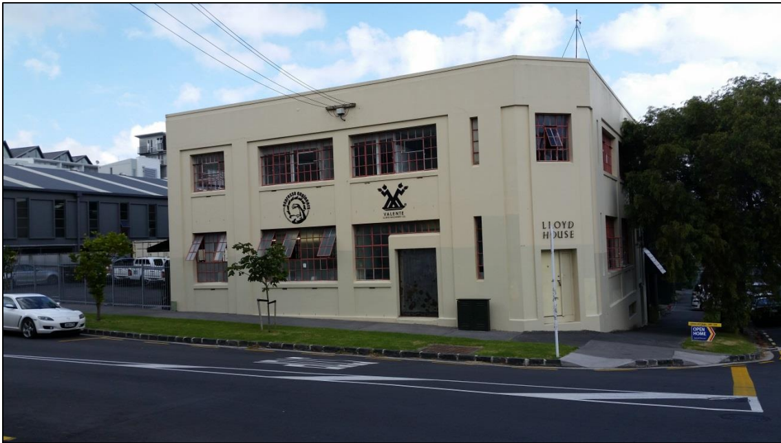
Mackelvie Street façade taken from north eastern corner of street.
