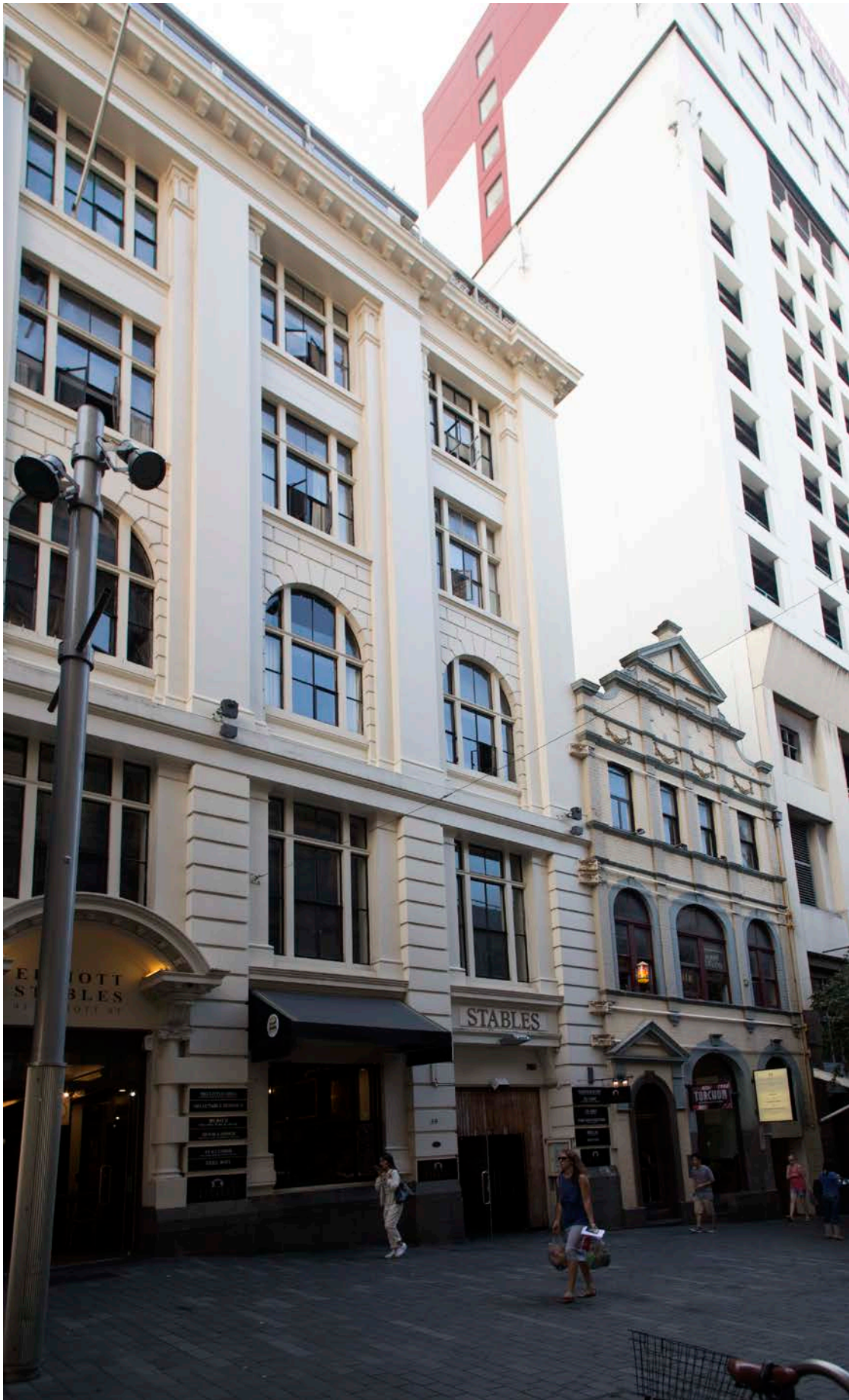
Figure 27: Elliott Street with Archibald Clark and Sons Warehouse, 39 Elliott Street and Atrium on Elliott. Rachel Ford 04/04/2017
