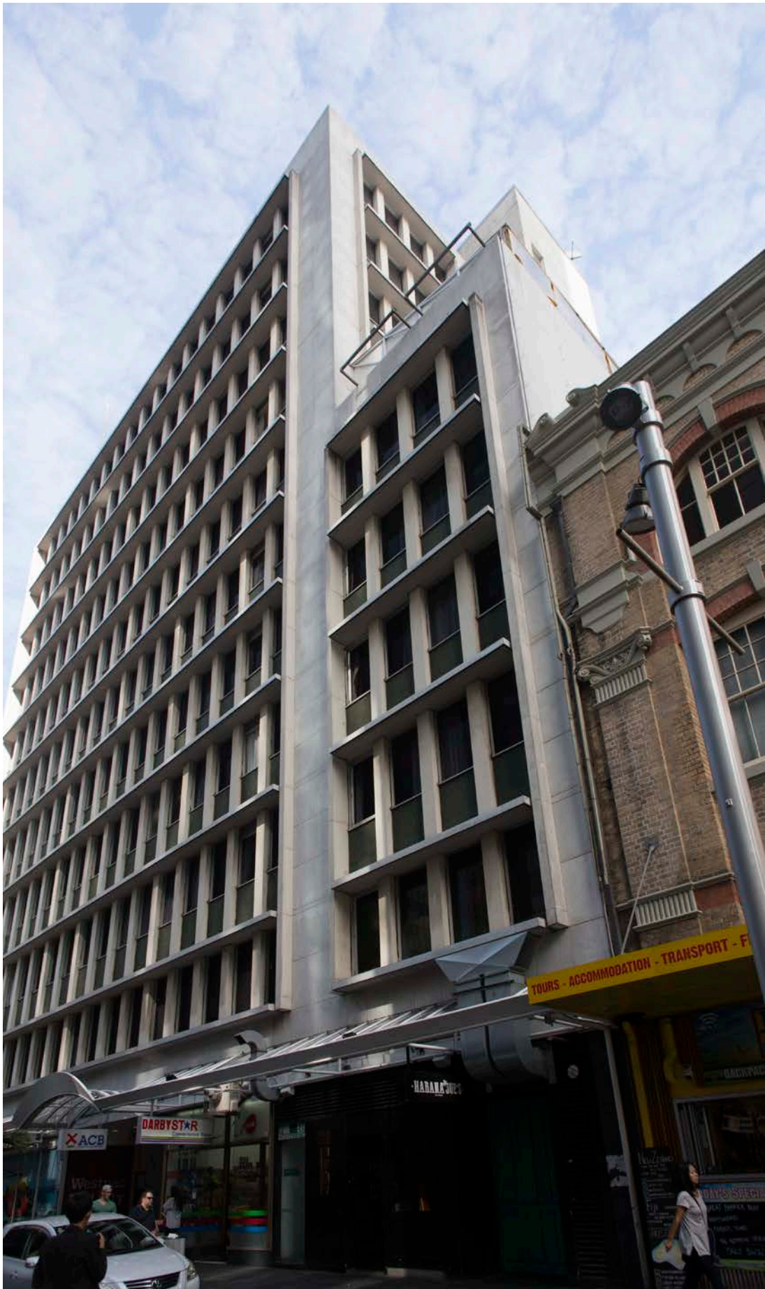
Figure 43: The junction between the Darby building and the neighbouring office building on Queen Street. Rachel Ford 04/04/2017
