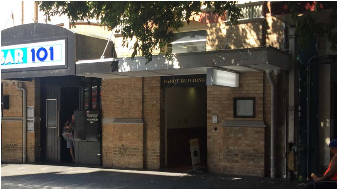
Figure 50: Darby Building sign above the main entrance. Anna Boyer 06/03/2017
