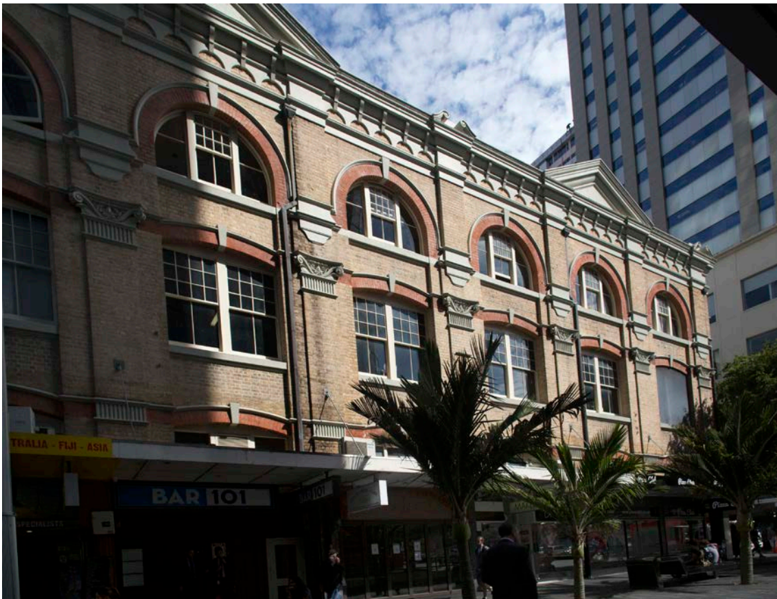
Figure 42: Darby Street facade looking towards Elliott Street. Rachel Ford 04/04/2017
