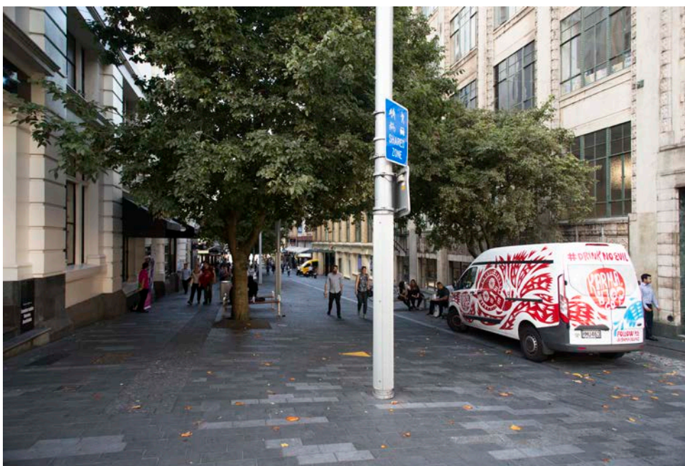
Figure 9: Wellesley Street entrance to Elliott Street. Archibald Clark and Sons Warehouse (left) and Smith & Caughey (right). Rachel Ford 04/04/2017
