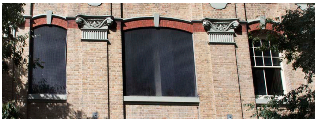
Figure 13: Detail of meshed out windows, first floor on Elliott Street. Rachel Ford 04/04/2017
