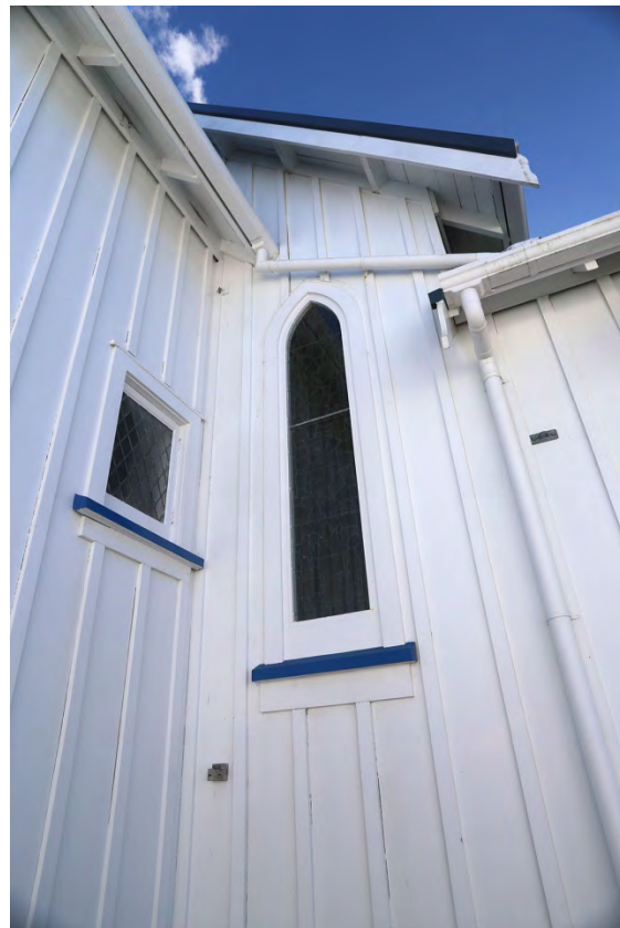
Figure 31: South elevation of vestry. The window on the right was shipped from London and installed in 1961
