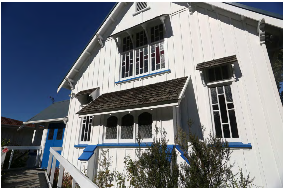
Figure 25: Northern elevation of Church showing window details and shingles. The additional doors and access ramp can be seen to the left.
