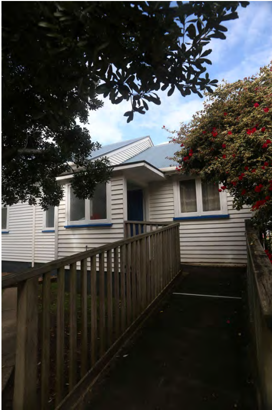
Figure 32: Western Entrance and porch to (northern elevation)
