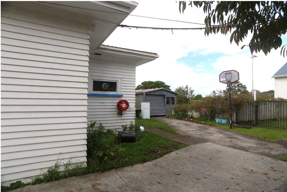
Figure 39: Back of Eastern elevation showing attached fire hose and garage.
