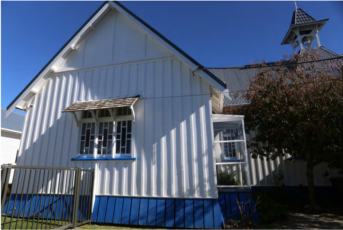
Figure 29: Vestry on eastern elevation. Addition of shelter to the north face can be seen and the stairs have been realigned.
