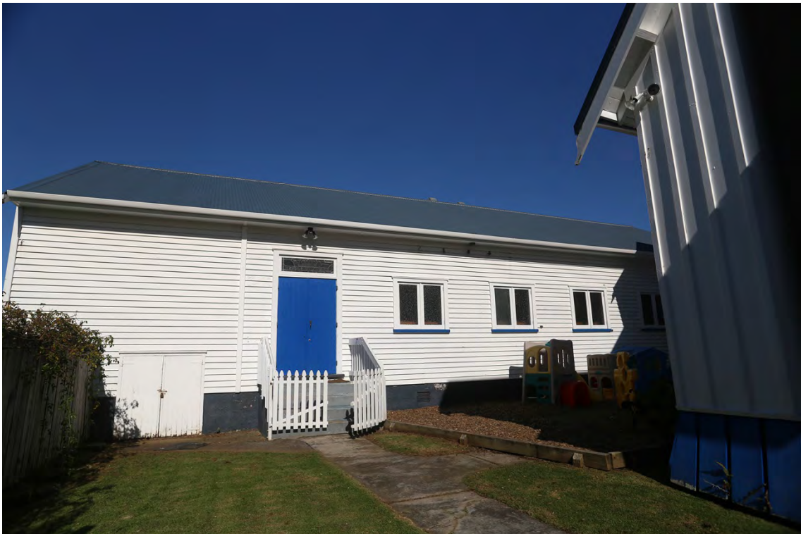
Figure 36: Northern elevation of Rattray Memorial Hall at the rear of the church (right)
