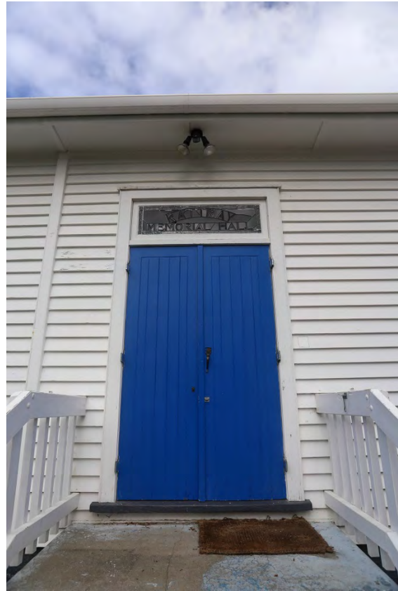
Figure 33: Main entrance to hall Hall (northern elevation)
