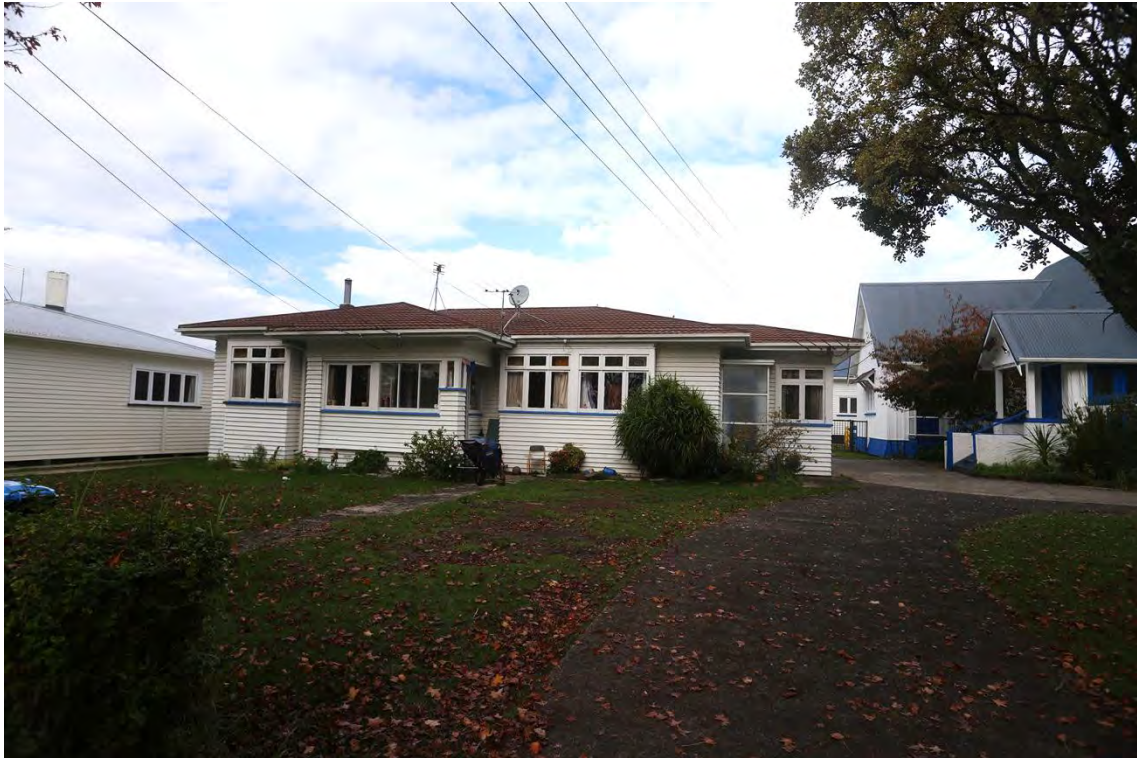
Figure 37: Vicarage from Dignan Street (northern elevation) showing extensions and the enclosing of the front porch.
