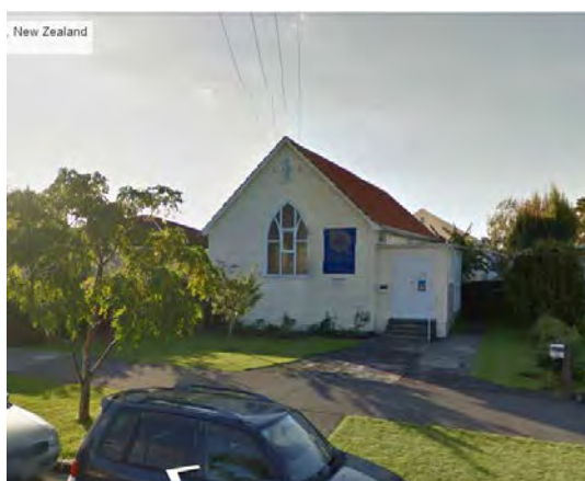
Figure 23: The former Baptist Church as seen from Formby Avenue (Google Street View 25 June 2014)
