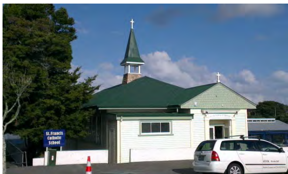
Figure 20: St Francis Catholic Church (May 2014)
