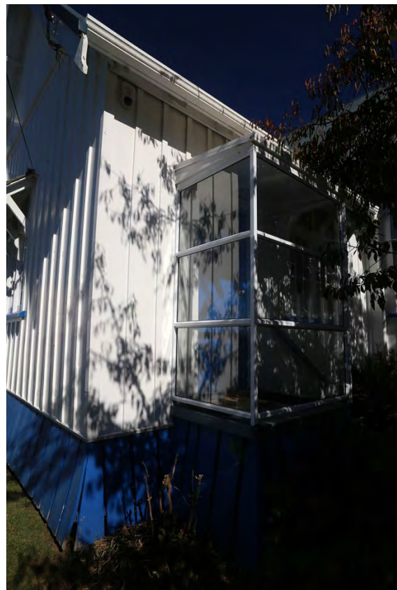
Figure 28: Addition to entrance of Vestry
