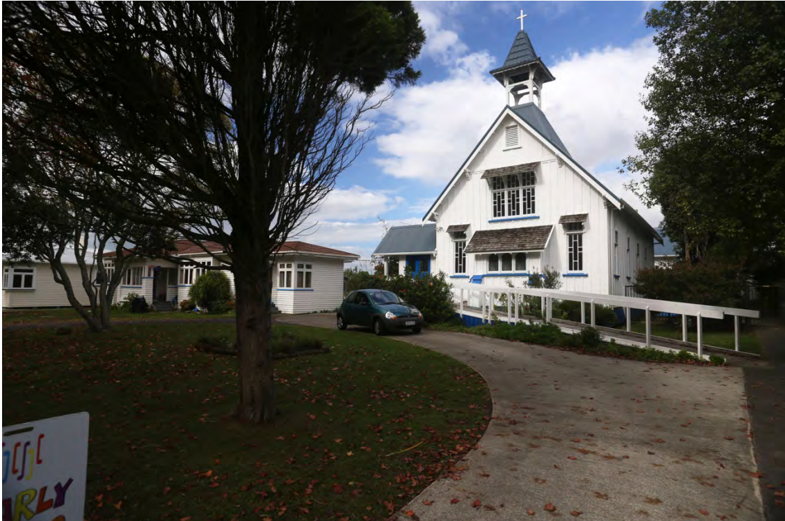
Figure 24: Church of the Ascension northern elevation showing access ramp to the church and the vicarage on the left.
