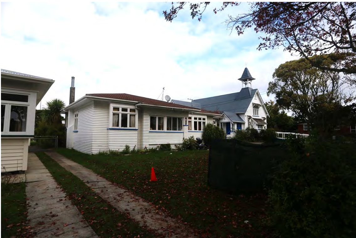
Figure 40: North and east elevations from Dignan street showing 1949 chimney
