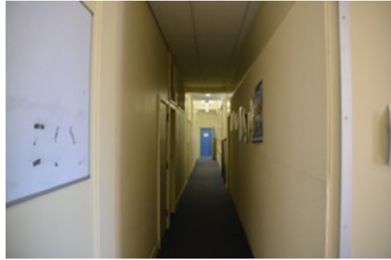
Figure 15: The main corridor that runs almost the full width of the building, with linoleum covered floor, painted plastered wall lining, and fibrous plaster ceiling tiles.
