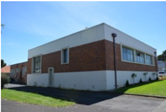
Figure 8: Part east and south (rear) elevations. The horizontal emphasis of the wall cladding is especially evident here.
