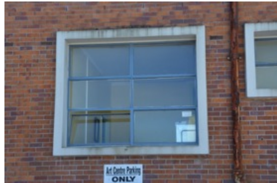
Figure 13: Showing one of multi-glazed metal windows, set within projecting concrete box frames, a distinctive feature of the buildings design.
