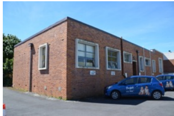
Figure 9: West and part south (rear) elevations of the western, more restrained, portion of the building.
