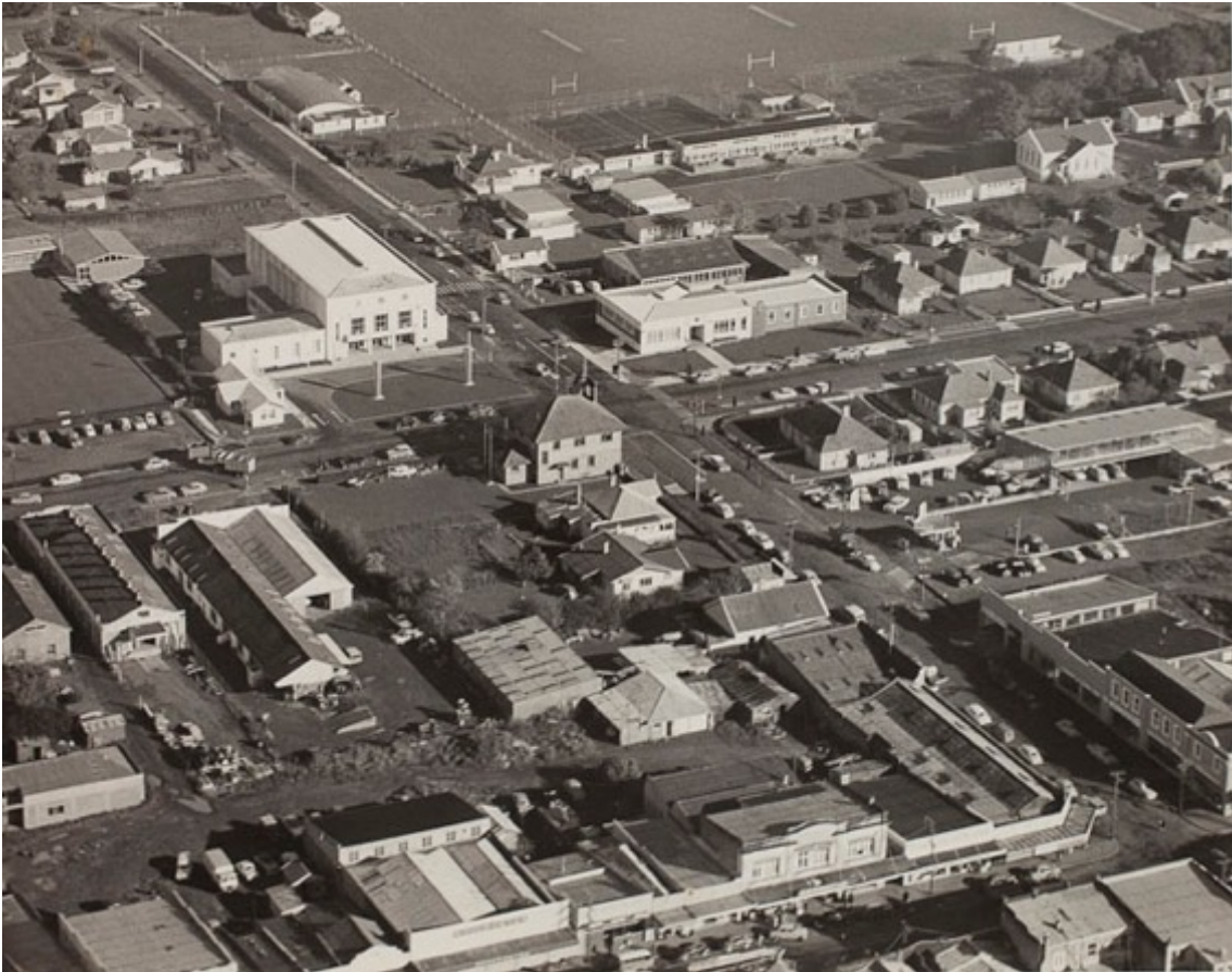
Figure 36: Aerial view of Pukekohe looking roughly southwest, 1961, the newly opened Municipal Chambers and Public Library (just above mid-centre). Refer to Figure 19, Appendix 1 for a close-up image (Auckland Libraries, South Auckland Research Centre, FRA: I, 5, Footprints 03147).
