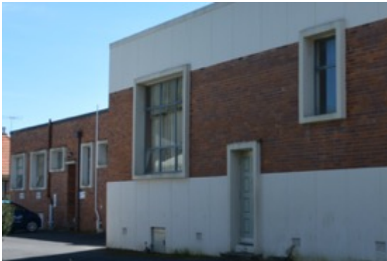
Figure 12: The collection of openings on the rear elevation.
