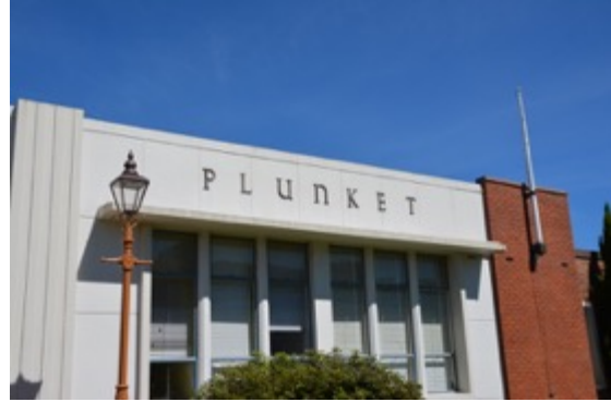
Figure 11: One of the main multi-glazed windows and 'Plunket' sign.
