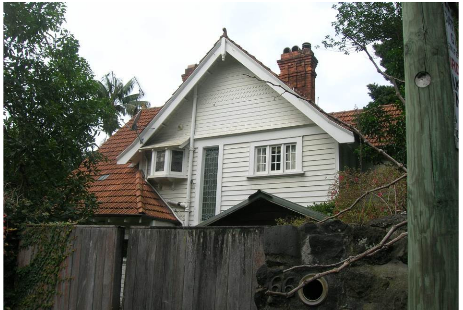
▲ 66-68 Gillies Avenue, showing gable and oriel window
