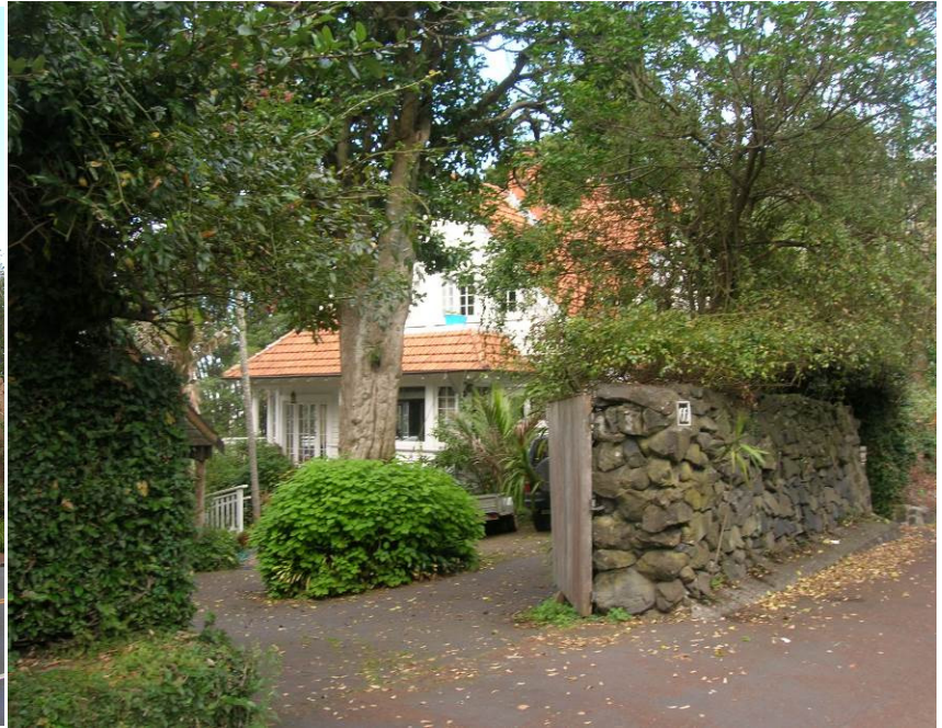
▲ figure 1: Two views of the property from Gillies Avenue – Salmond Reed Architects, May 2016
