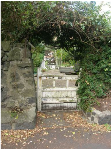
▲ 66-68 Gillies Avenue: Entry Gate
