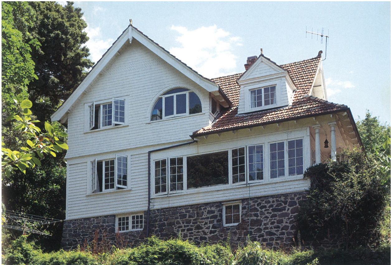
▲ 66-68 Gillies Avenue, Epsom, before the 2009 alterations at basement level
