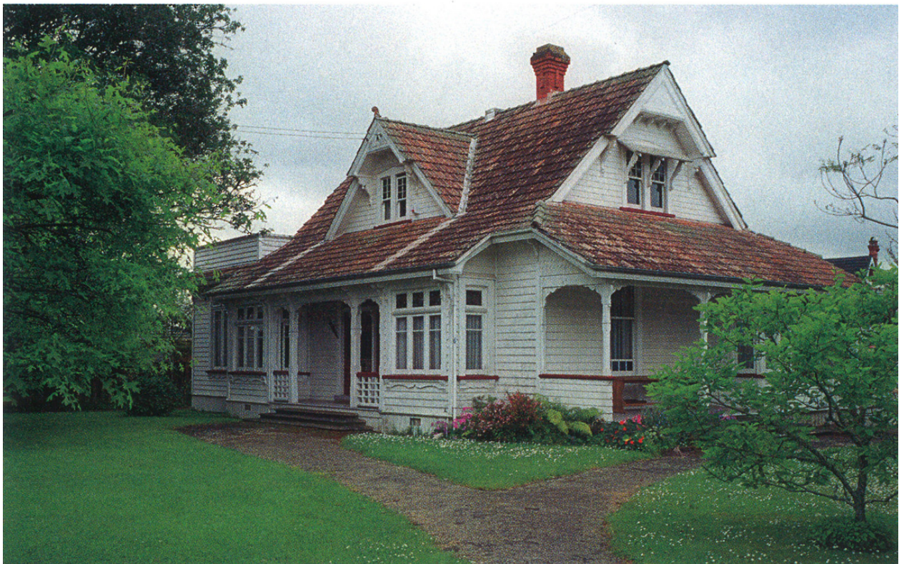
▲ 11 Kimberley Road, Epsom, recently demolished
