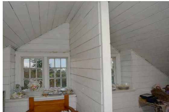
Figure 19: Showing the attic space (THS, 2016).
