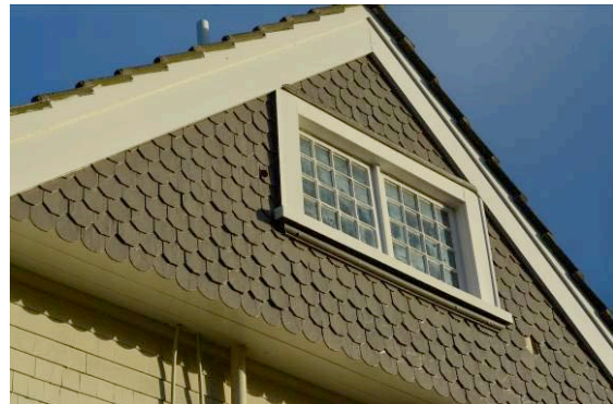
Figure 15: The north wing gable showing the use of both half-round and octagonal shingles and a multi-glazed attic window (THS, 2016).
