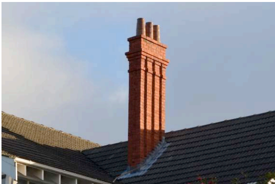
Figure 14: The corbelled and fluted brick chimney, located on the eastern roof slope (THS, 2016).
