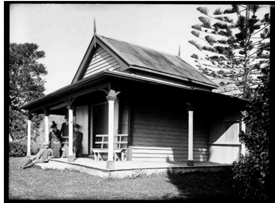
Figure 25: Showing a close up view of part of William Swainson’s former home, owned at the time by Mrs Street and used as a summerhouse, 1899. It was demolished in 1954. Sir George Grey Special Collections, Auckland Libraries, 1-W118
