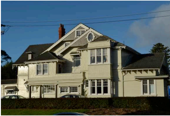
Figure 8: West (road-side) elevation, fronting Gladstone Road (THS, 2016)
