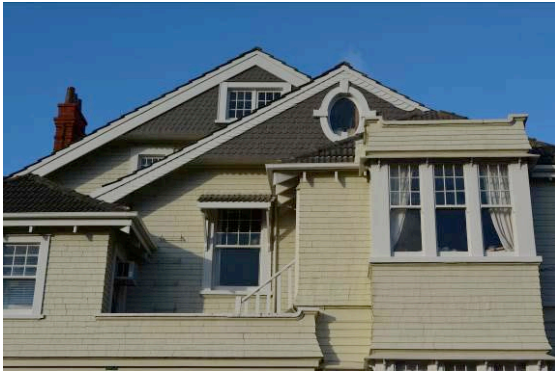
Figure 12: Showing the variety and layering of roof forms and windows visible on the west elevation (THS, 2016).
