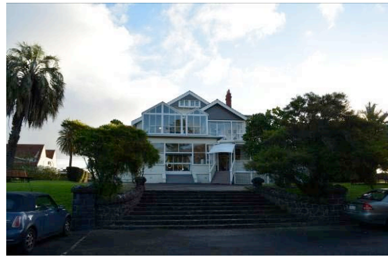
Figure 7: Showing the east (park-side) elevation of the building and rear stone steps, viewed from the car-park (THS, 2016).
