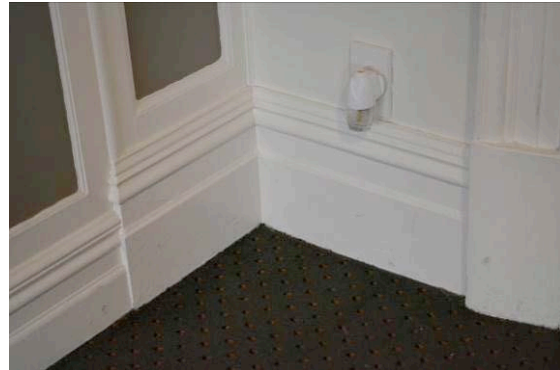
Figure 17: Profiled skirting boards (the varying heights possibly suggesting different dates), architraves and wall panelling (THS, 2016).
