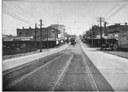
Figure 61. Dominion Road in Balmoral, 1920s
