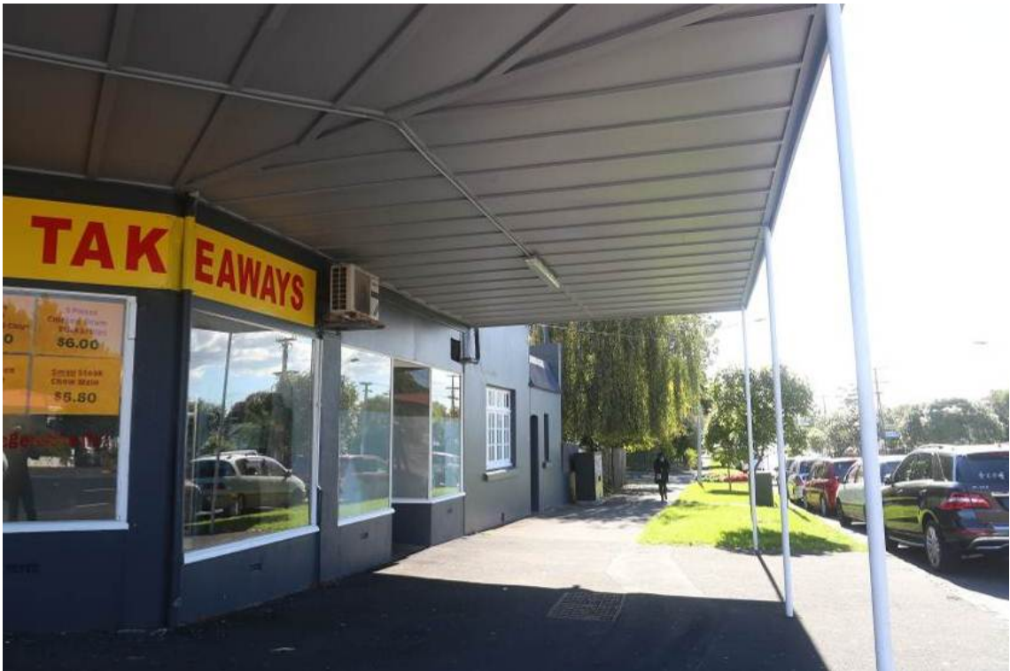
1041 Great North Road, detail of Premier Avenue storefronts (Rachel Ford, May 2014)
