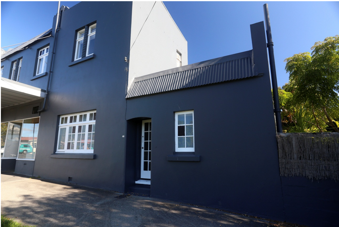
1041 Great North Road, detail of attached apartment at 2A Premier Avenue (Rachel Ford, May 2014)
