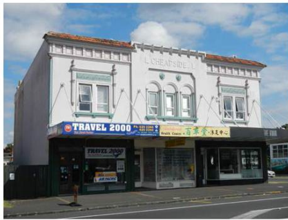
Cheapside Buildings, 727-731 Dominion Road
