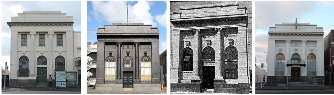
Figure 6: Patterson’s four monuments to thrift: 1928 Ponsonby, 1929 Symonds St (Khyber Pass), 1929 Dominion Road (demolished 1999), and 1931 Point Chevalier. Photos: David Reynolds.
