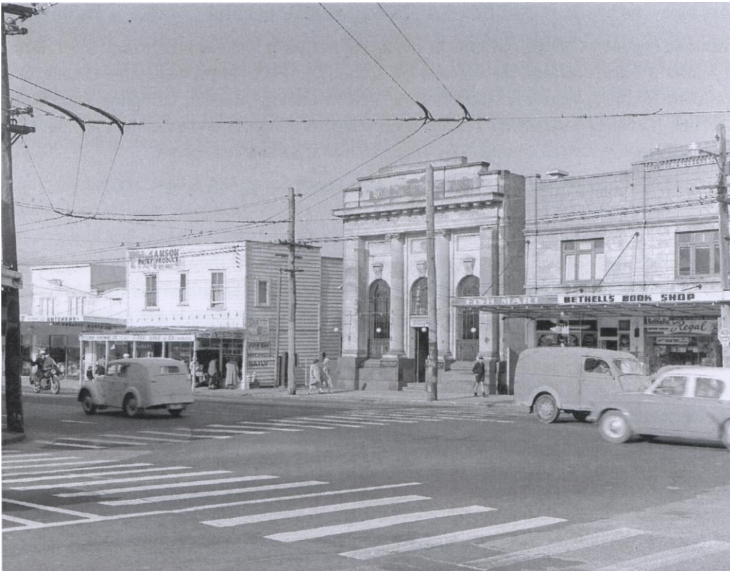
Figure 4: The Auckland Savings Bank building probably in the mid 1960s. The facade is unpainted and retains its original lighting. Photographer: Barry Mackay. Source: Point Chevalier memories, 1930's-1950's
