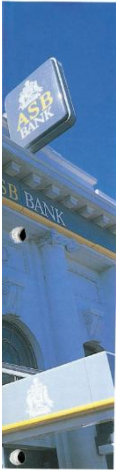
Above: Detail of the front facade of the Point Chevalier branch of the ASB, illustrating Patterson's use of displaced volute brackets to ornament the facade. (Photo: Bill McKay)
