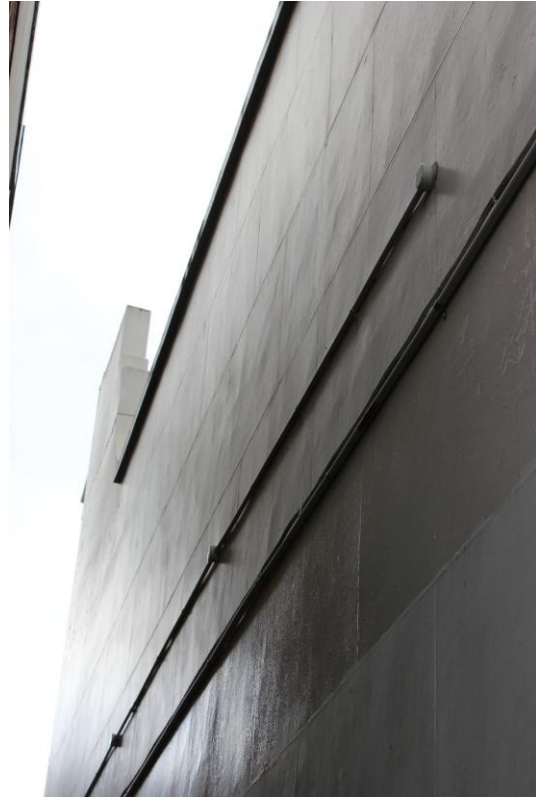
Figure 11: View along west wall from the side lane showing scribed lines in the cement render in imitation of ashlar. 13 May 2014 Photo: David Reynolds
