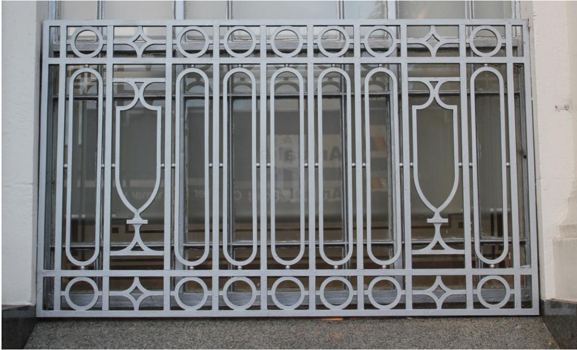
Figure 8: Security screens are fitted to both street windows. These have been painted in the new corporate livery but were once dark green. 29 March 2014. Photo: David Reynolds
