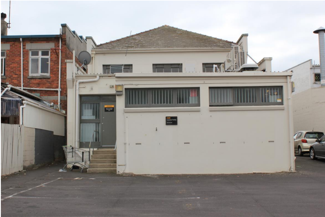
Figure 13: The south elevation with later additions beyond the original footprint of the 1930 plan. The building retains its original slate roof and terracotta ridging. 29 March 2014. Photo: David Reynolds
