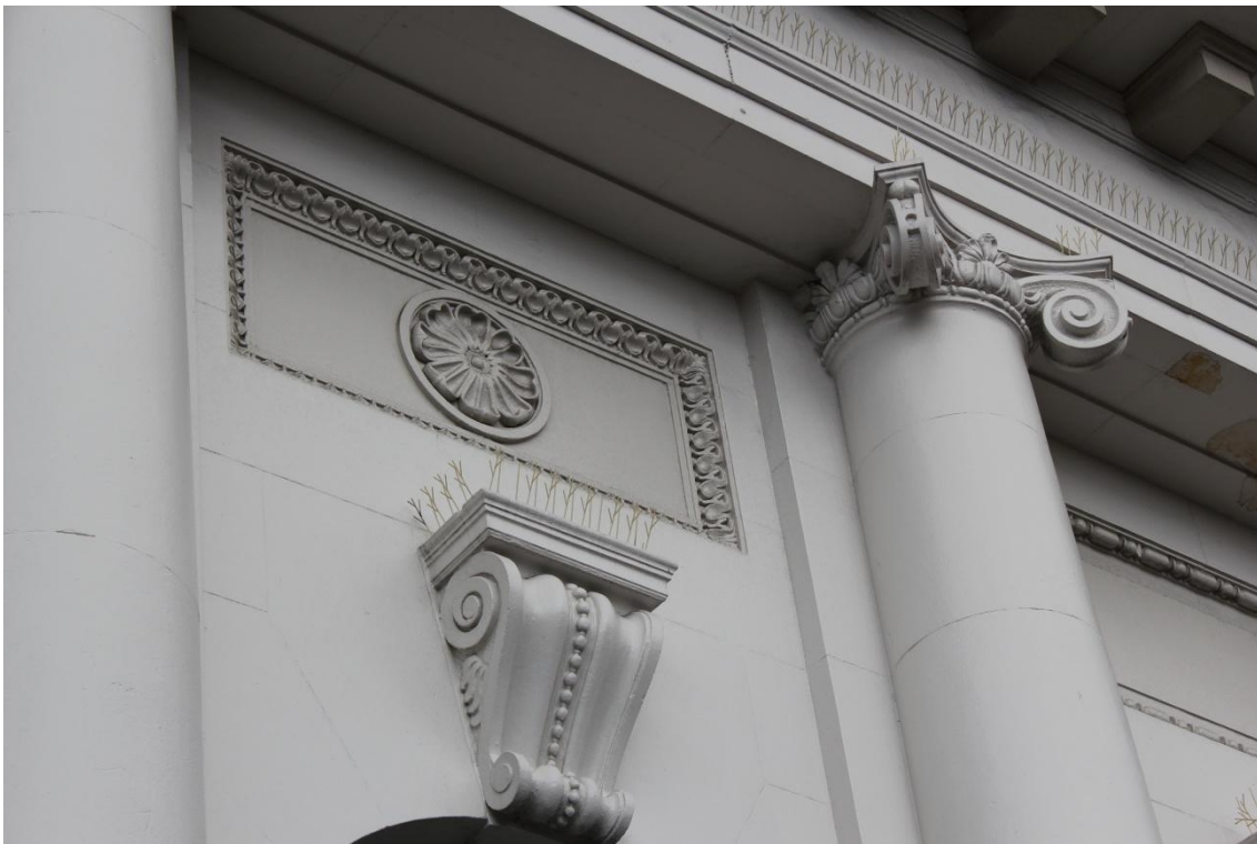
Figure 9: The central panel and its classical rosette, moulded ornamental bracket and Ionic order capital. Most of the potential roosting sites above window height have been fitted with Nixalite bird spikes. 13 May 2014 David Reynolds
