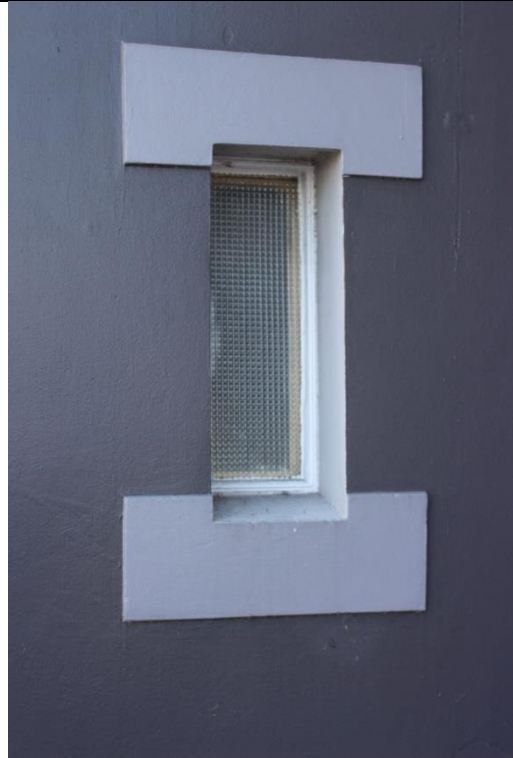
Window detail (Great North Road façade)
