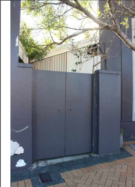
Gates to rear yard and utility area (Great North Road façade)
