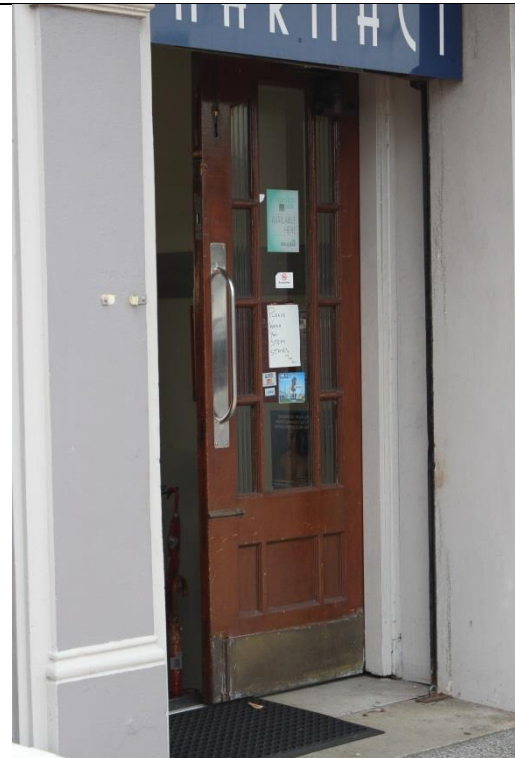
Doorway and door (Rosebank Road façade)
