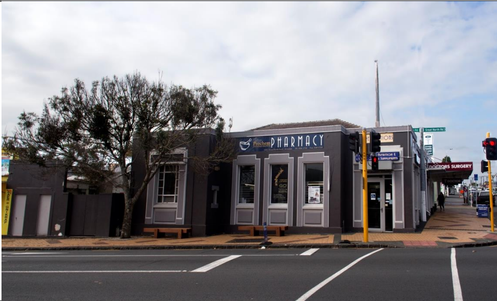
Great North Road façade, showing three bays, gates to the rear yard, and former telephone boxes (at right)
