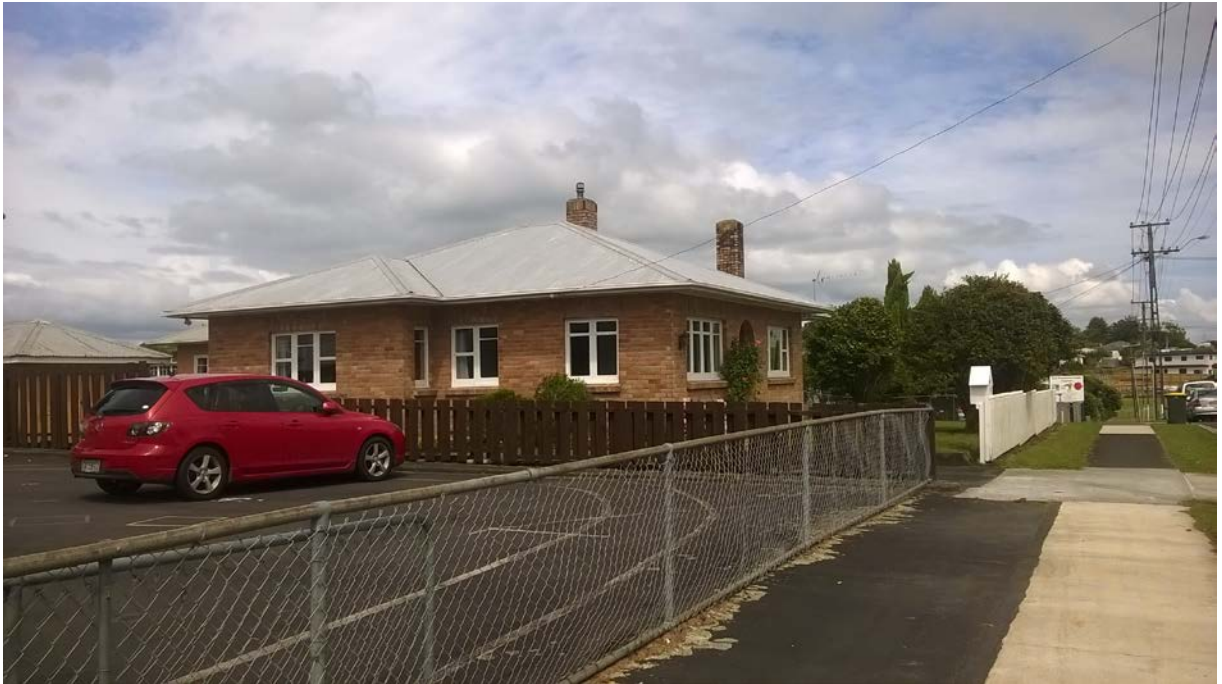
Figure 50. Neighbouring manse – also designed by Johnson Clark, but later in 1940.
