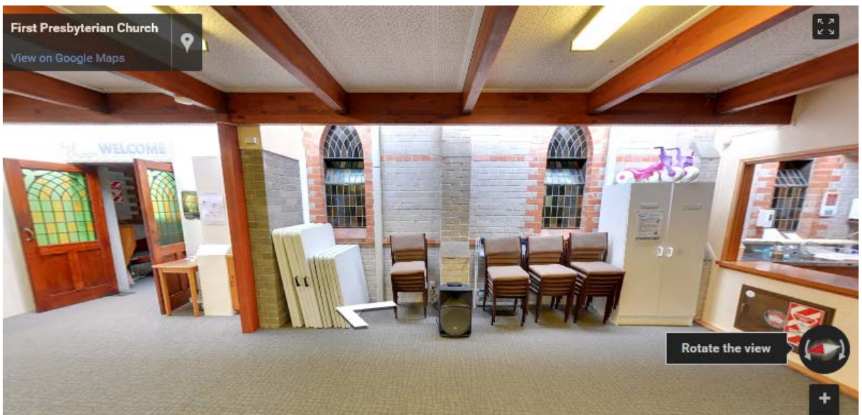
Figure 26. 1970s foyer area built beside the original exterior wall, which remains for the most part, intact. Seeinside, May 2016.
