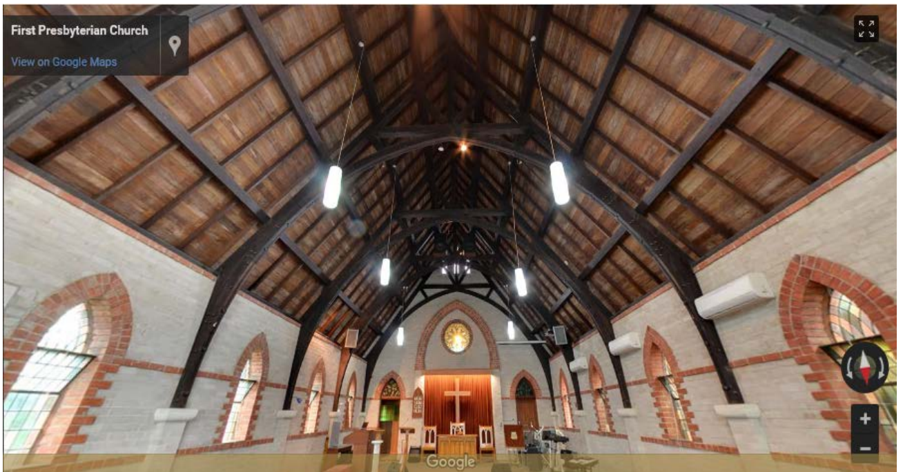
Figure 27. Arched windows and truss ceiling with exposed rafters. Seeinside, May 2016.
