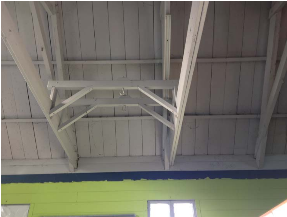
Figure 47. Timber ceiling system (unidentified hooks present).
