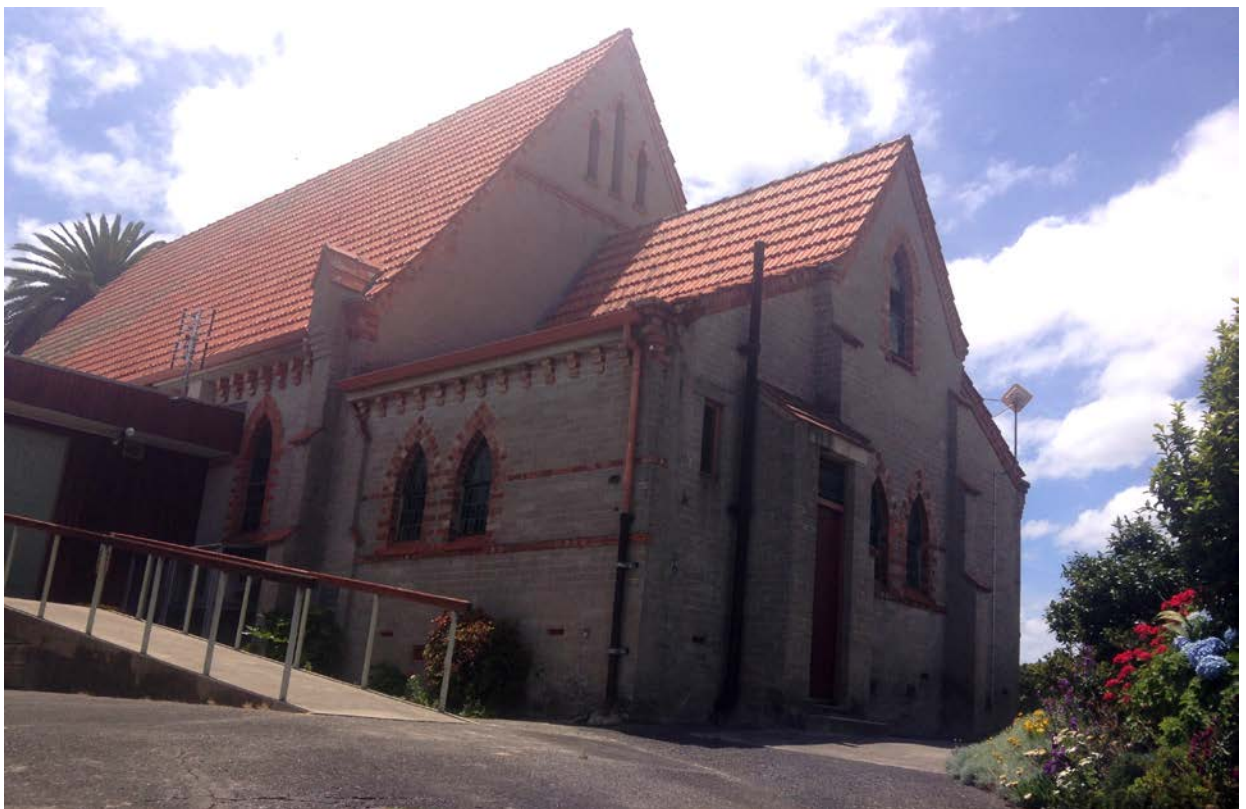
Figure 21. Rear elevation of the 1926 church building.
