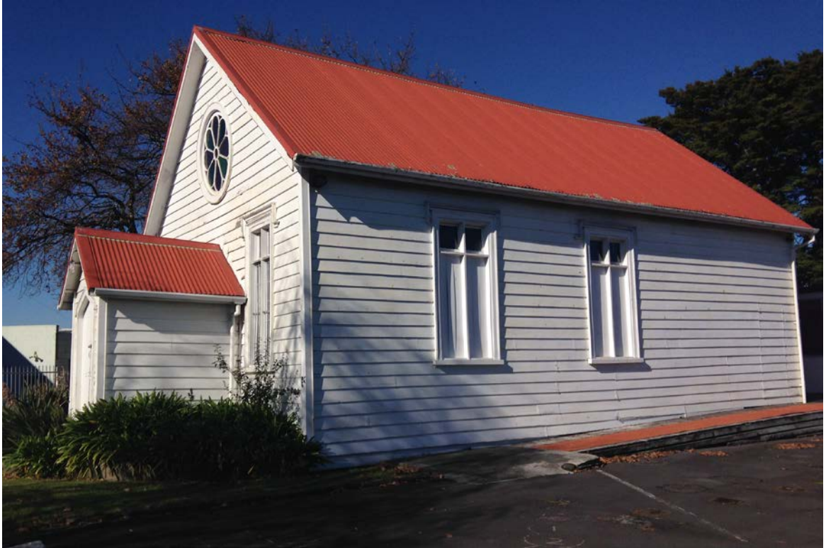
Figure 34. Side elevation – the third window on side elevation has been removed and replaced with weatherboards.
