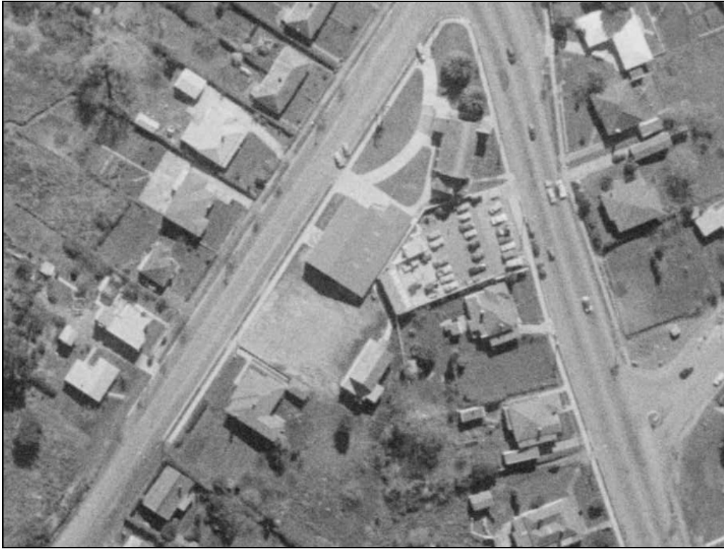
Figure 130. Aerial map of church site in 1960. (CROWN 583_1928_11). Source: Land Information New Zealand.
