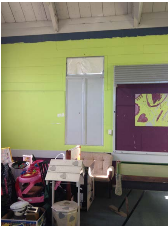
Figures 49. Left: side wall elevation. While cosmetically the current colour palette is not a sympathetic feature the materiality on the upper level of the walls remains sympathetic. Right: Front entrance door, as seen from inside the portico.
