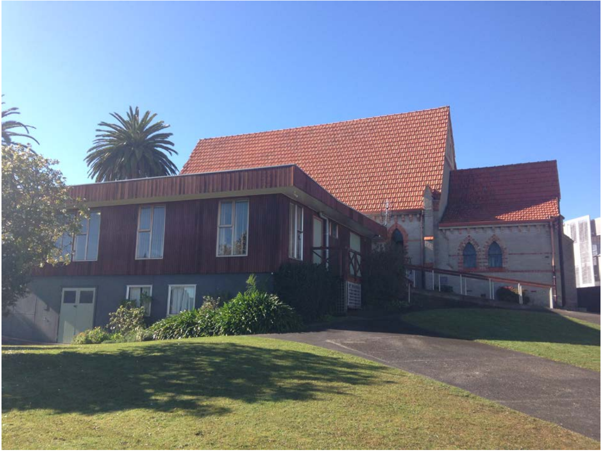
Figure 22. 1970S/1980s addition in relation to the 1926 church building. June 2017.
