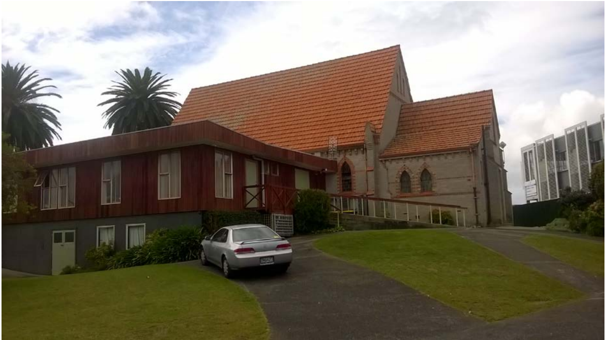
Figure 11. The 1975 ground level and basement addition attached to 1926 church, as seen from the rear of 67 Great South Road.
