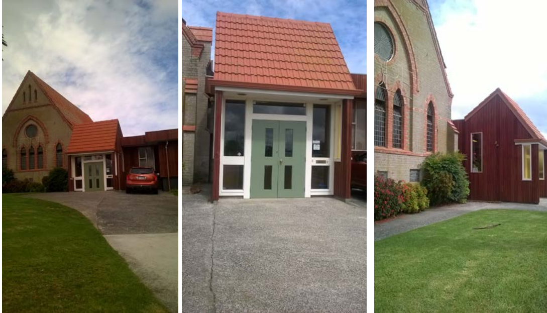
Figure 13. Left: view as seen from corner footpath of Great South Road and Coles Crescent.
