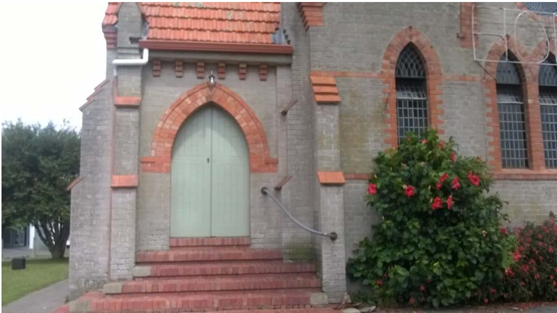
Figure 17. Arched side door entrance with steps.
