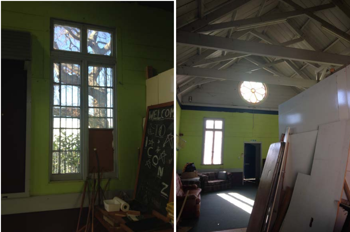
Figure 48. Left: wall and window. Right: Internal view, looking to the front of the building.
