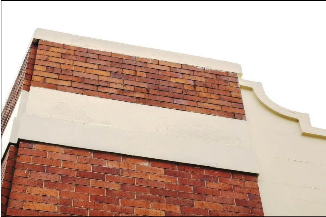
Figure 41: The site May 2016 – The southern elevation – looking at the ‘returned’ brick, the parapet coping and the rendered banding – under which may be the original Lichfield stone. Photograph: Blair Hastings.
