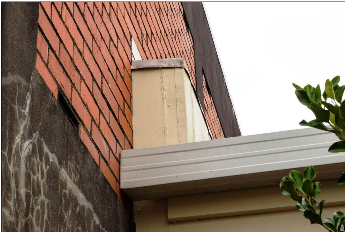
Figure 46: The site May 2016 – The parapet rear wall of the circa 1973 addition – connected to the neighbouring building at 152 Green Lane West. Photograph: Blair Hastings.
