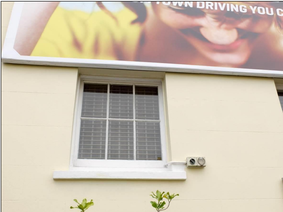
Figure 52: The site May 2016 – The northern elevation – showing the fixed timber window south of the two hung sash windows. Photograph: Blair Hastings.
