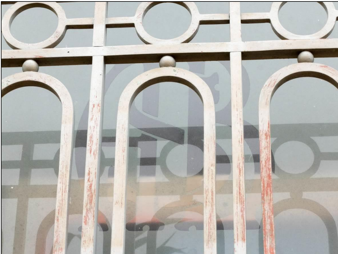
Figure 55: The site May 2016 – 'ASB' reverse frosted into the lower sash glazing of the main / street elevation windows. Photograph: Blair Hastings.
