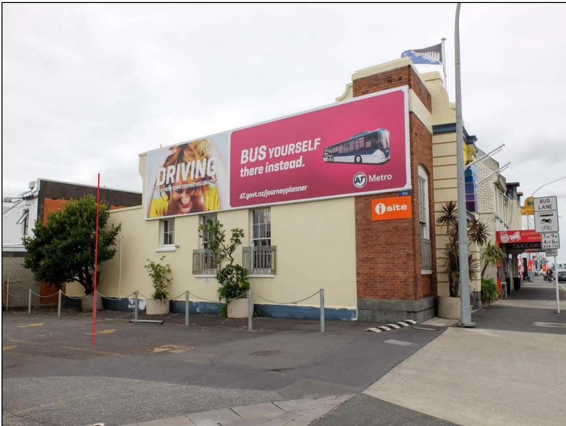
Figure 39: The site May 2016 – Looking at the intact northern elevation. The red line to the left hand side of the photograph shows the approximate line of the 1973 extension. Photograph: Blair Hastings.
