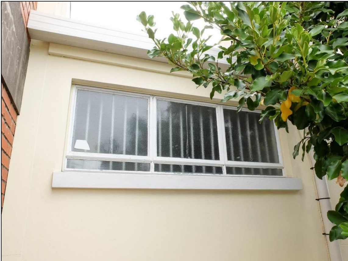
Figure 50: The site May 2016 – The circa 1973 addition to the rear of the original building - showing the use of steel and not timber window joinery. Photograph: Blair Hastings.
