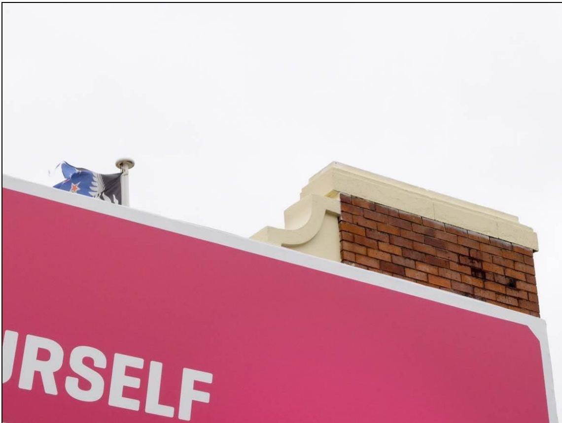
Figure 43: The site May 2016 – The northern elevation – looking at the returned brick, the parapet coping and the advertising billboard. Photograph: Blair Hastings.
