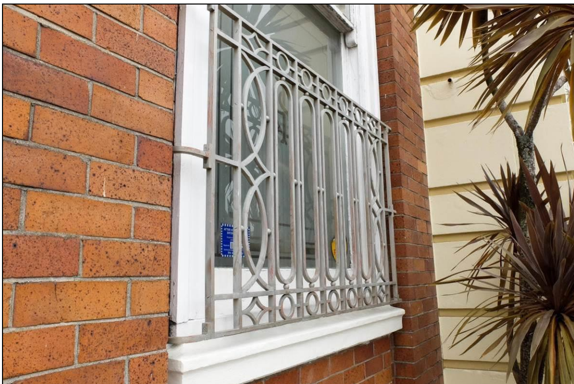
Figure 54: The site May 2016 – One of the two hung sash windows on the main / street elevation. The decorative security screen was originally specified in bronze. Photograph: Blair Hastings.
