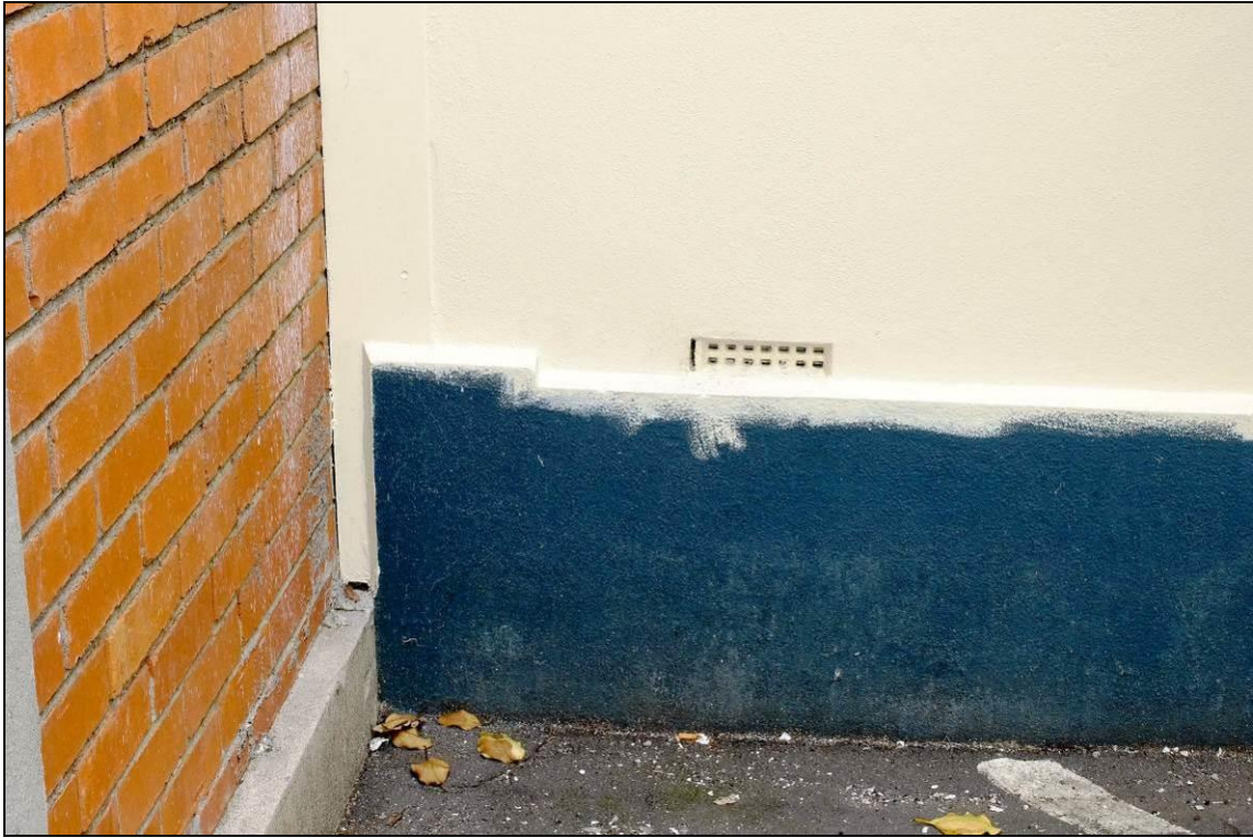
Figure 49: The site May 2016 – The rendered ‘skirting’ of the northern elevation – at the rear of the subject building – connected to the neighbouring building at 152 Green Lane West. Photograph: Blair Hastings.
