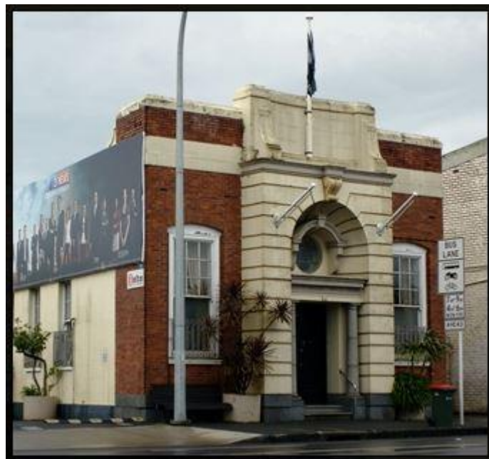
Figure 69: Photographs September 2011 - http://timespanner.blogspot.co.nz/2011/09/bank-re-used.html .
