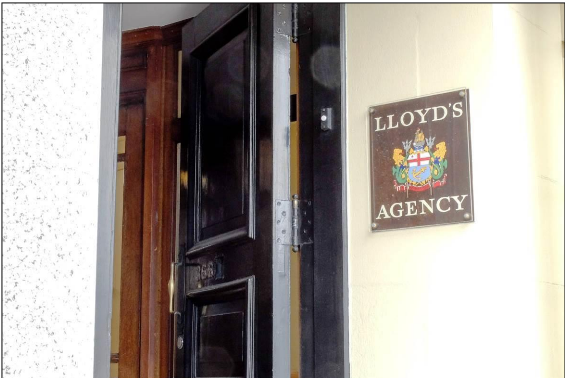
Figure 68: The site May 2016 – The main elevation – showing the current tenant's signage – face fixed through the cement render. Photograph: Blair Hastings.
