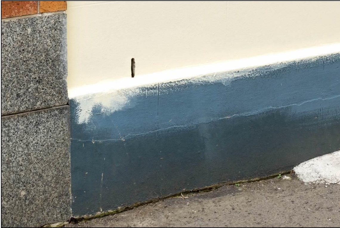
Figure 45: The site May 2016 – The rendered and painted 'skirting' along both long or side elevations. Photograph: Blair Hastings.
