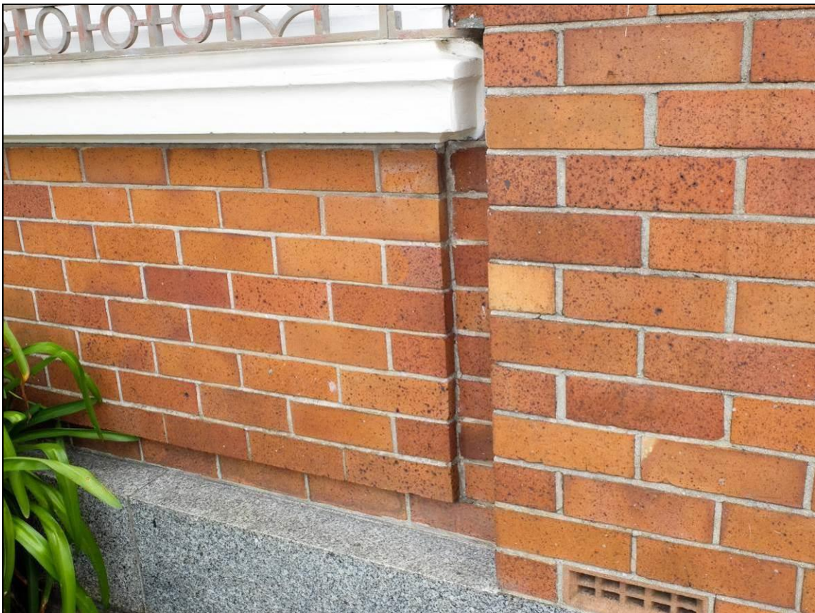
Figure 64: The site May 2016 – The main or street elevation – showing the stretcher bonded brick with subtle stepping to gain some relief and shadowing in the overall form. Photograph: Blair Hastings.
