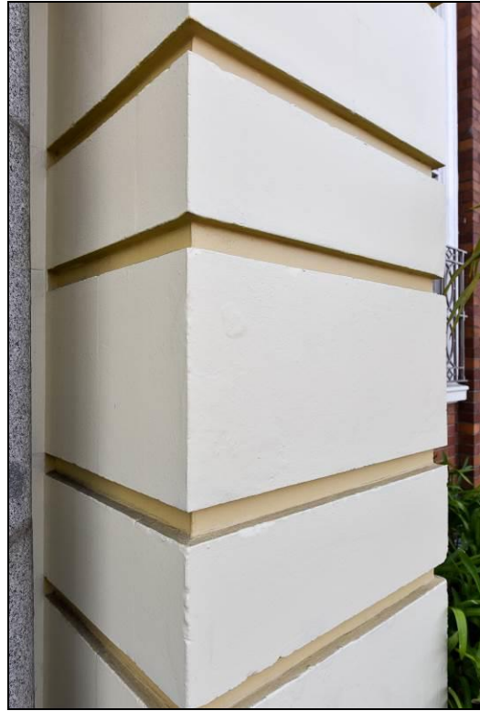
Figure 57: The site May 2016 – Street elevation details: Left: Corner brick-work. Right: Cement rendered quoining. Photographs: Blair Hastings.
