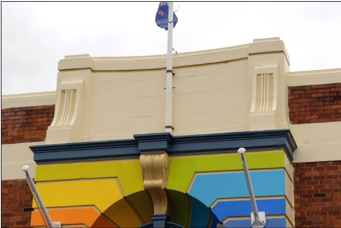
Figure 63: The site May 2016 – The main or street elevation – showing the main pediment which originally had brass bank lettering – cement render has covered any original fixings. Photograph: Blair Hastings.
