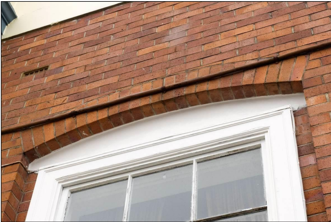
Figure 67: The site May 2016 – The main elevation – showing the subtle recessing of the timber window in the gently arched head. Photograph: Blair Hastings.
