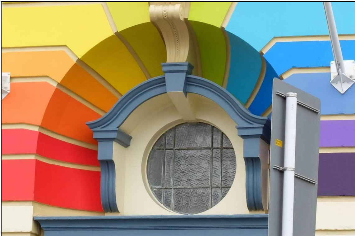
Figure 62: The site May 2016 – The main or street elevation – showing the 'playful' composition of classical elements, the equally 'playful' recent paint scheme and the face-fixed banner-hangers. Photograph: Blair Hastings.
