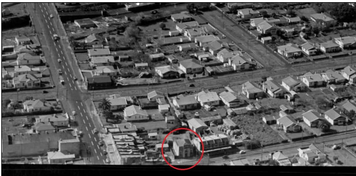
Figure 32: Aerial photograph of Ellerslie Racecourse and Greenlane (looking east), 1 September 1949. Full image top, extract bottom. The 'local' shops were still standing – north of, or to the left of the bank. Ellerslie Racecourse, Auckland. Whites Aviation Ltd :Photographs. Ref: WA-21789-G. Alexander Turnbull Library, Wellington, New Zealand. http://natlib.govt.nz/records/22870975
