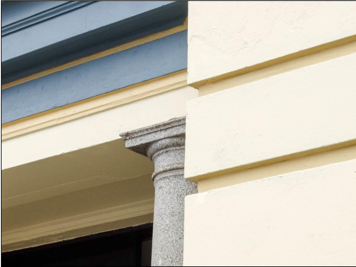
Figure 59: The site May 2016 – Architectural detail of the main elevation – Tuscan column (one of two). Photograph: Blair Hastings.
