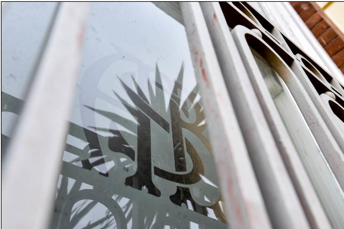
Figure 56: The site May 2016 – 'ASB' reverse frosted into the lower sash glazing of the main / street elevation windows. Photograph: Blair Hastings.
