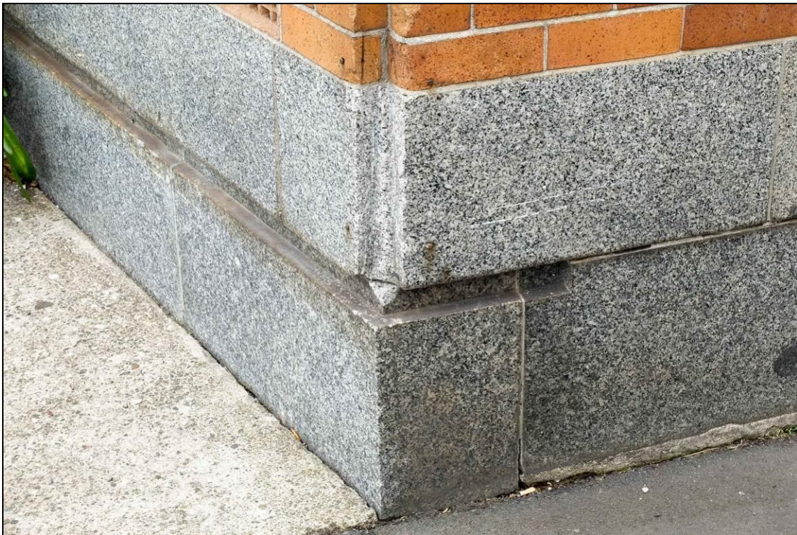
Figure 44: The site May 2016 – The south-west corner – looking at the granite base – note the rebated horizontal corner detail common to all branch buildings in Patterson's series. The vertical corner above the rebate has broken away. Photograph: Blair Hastings.
