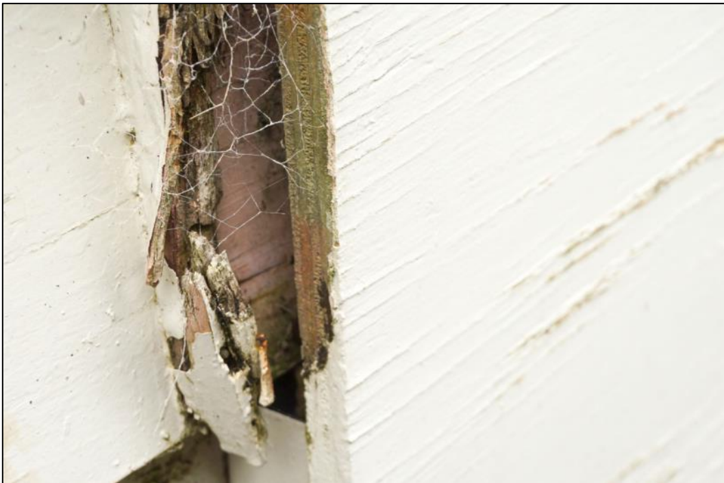
Figure 94: External weatherboard detail – rotten boards have been covered rather than replaced. Ingress is continuing – further fabric failure likely. Some evidence of previous paint colours (possibly undercoat) evident. Photo: Blair Hastings – March 2017.
