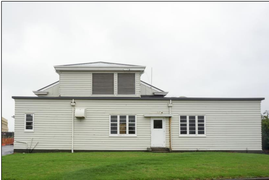
Figure 73: North elevation of the building. Windows appear to be original although when compared to the Wigram Institute Building, some windows may have been removed around the kitchen – perhaps to accommodate larger cooking facilities. Grille to projection room modified. Photo: Blair Hastings – March 2017.
