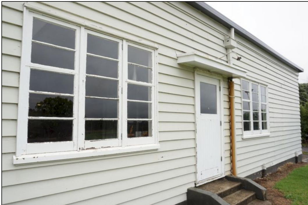
Figure 88: Casement windows similar to those used in state houses at the time. Modern internal fixings. Transoms match the proportioning used in the hung windows seen along the main or east elevation. The porch is quite likely original. A mixture of plumbing fixtures evident. Photo: Blair Hastings – March 2017.
