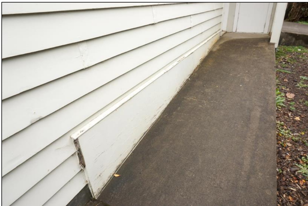
Figure 72: Ramp detail from above. Boarding has been applied to cover rotten weatherboards and floorboards internally. A temporary repair job that will need attention. Photo: Blair Hastings – March 2017.
