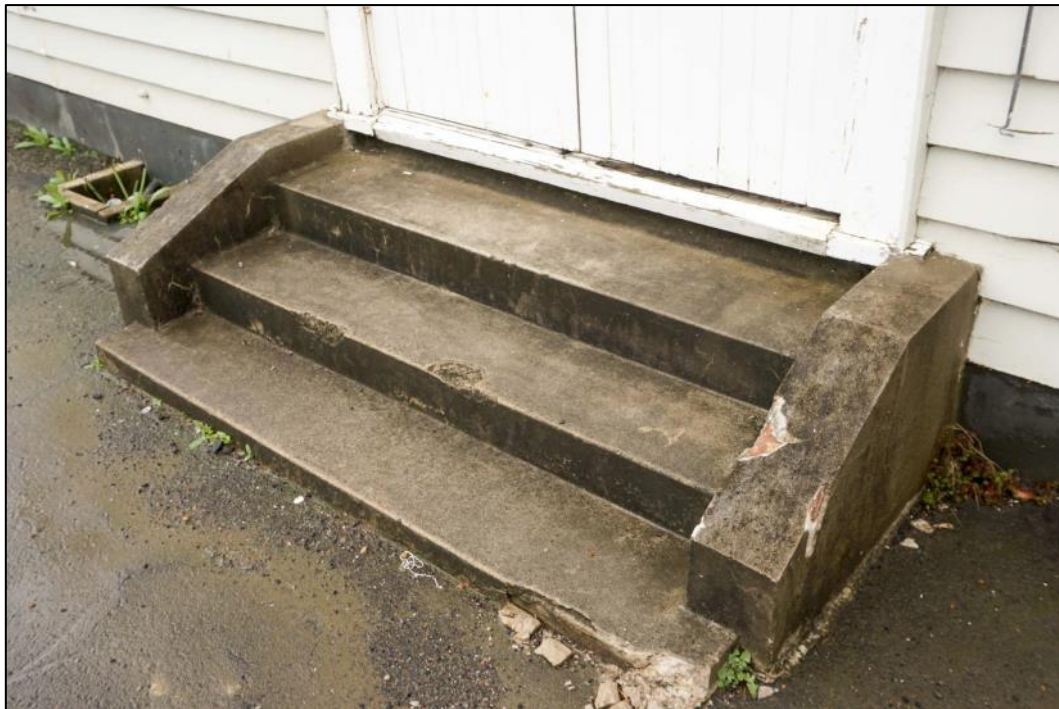
Figure 83: Southern section of the east elevation – original steps into the main hall space show concrete render over brick. The disrepair is common across material and fabric across the exterior shell of the building. Photo: Blair Hastings – March 2017.
