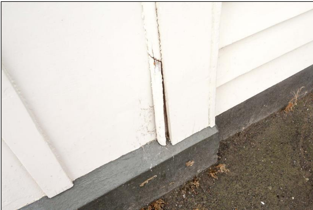
Figure 96: External beading failure - indicative of many similar problems across the exterior shell. Photo: Blair Hastings – March 2017.
