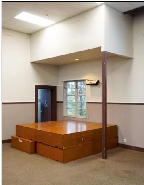
Figure 101: Interior – Southwest corner of the interior – originally part of the dressing room – walled off from the Hall (from where the photo is taken) and the stage, to the left. The column is modern – as is the ceiling. The dressing room was originally accessed from a door to the right of the window – now removed. Photo: Blair Hastings – March 2017.
