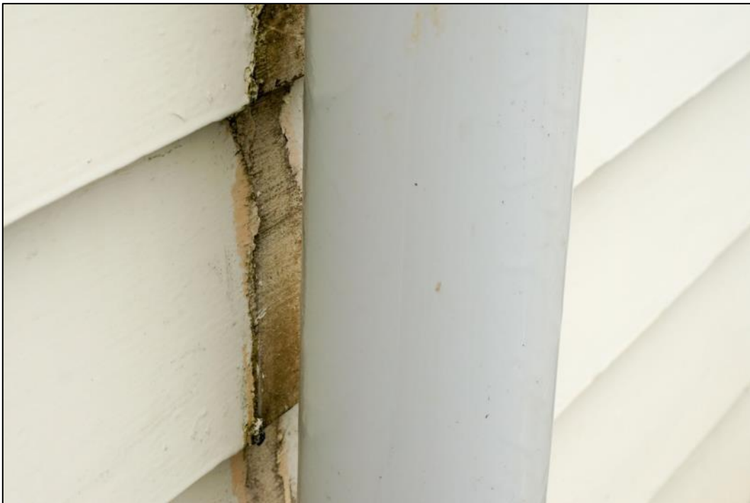
Figure 92: External paint detail – no paint behind downpipe - common across the exterior shell – will cause material and fabric failure. Photo: Blair Hastings – March 2017.
