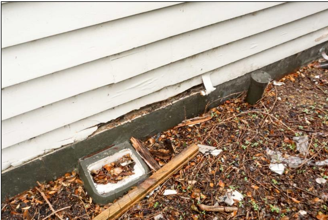
Figure 93: External weatherboard and drainage detail – weatherboards rotten and hard landscaping not calibrated correctly – water falling to the building. Photo: Blair Hastings – March 2017.
