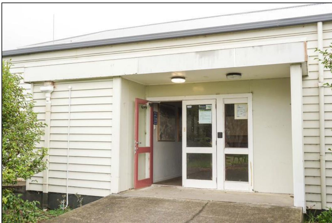
Figure 70: Close-up image of the entrance porch seen above. Not original to the building. Modified doors. Photo: Blair Hastings – March 2017.
