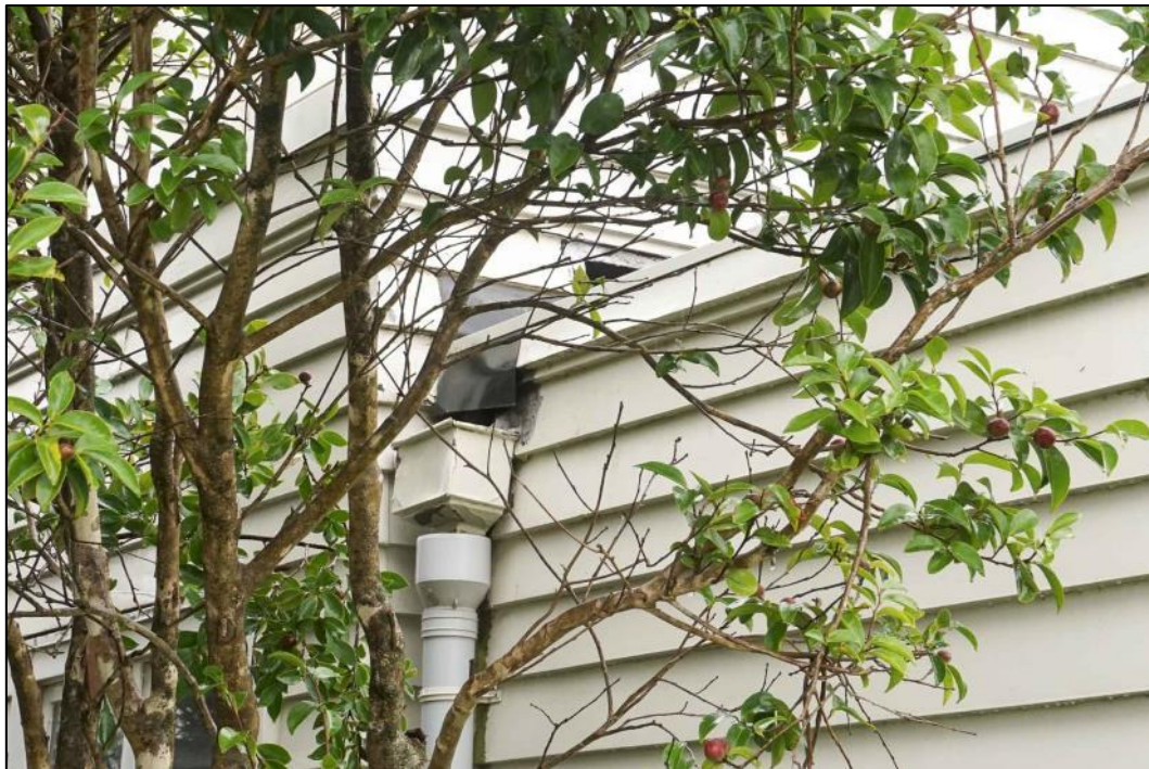
Figure 97: Rainwater head, downpipe and flashing system all incompatible with one another - at this and similar junctions across the building. Roofing does not appear to have been redone in conjunction with re-roofing the main hall and apron space 2014. Photo: Blair Hastings – March 2017.
