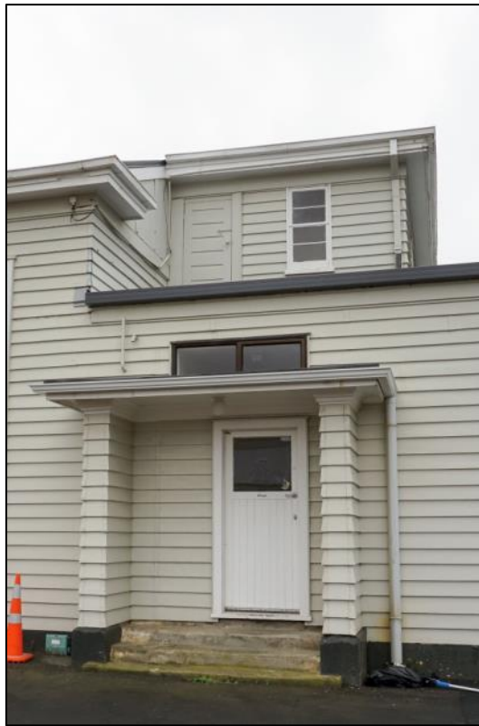
Figure 77: Northern end of east elevation. Porch detail original. Opening modified. Joints clearly show where the original door was. Modern aluminium windows above. projection room above that again. Photo: Blair Hastings – March 2017.
