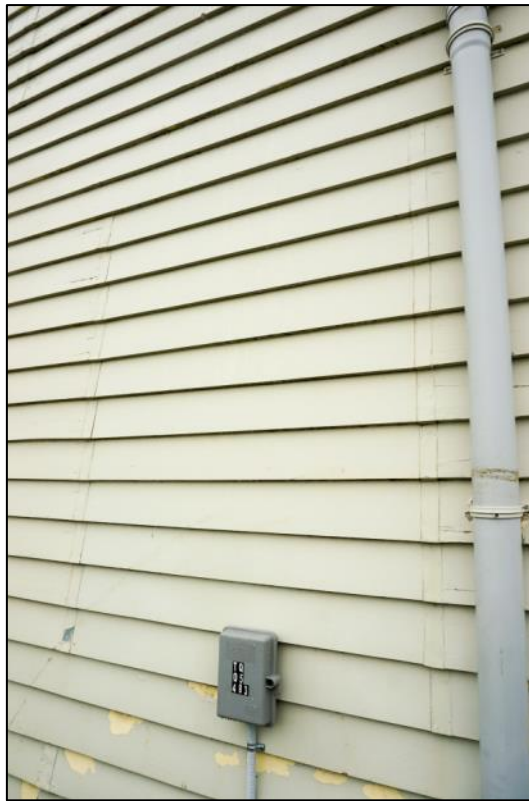
Figure 81: Southern section of the west elevation – the outline of the original door and steps into the dressing room can be seen in the tin weatherboard jointers – refer also below. Photo: Blair Hastings – March 2017.
