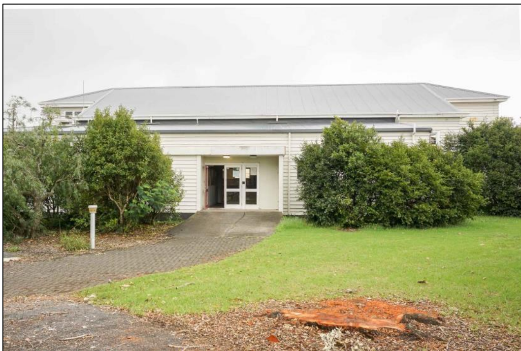
Figure 69: Looking east at the west elevation of the subject building. The porch that provides shelter external to the main door has been added. The roof above the entrance foyer has re-pitched and re-roofed. Photo: Blair Hastings – March 2017.
