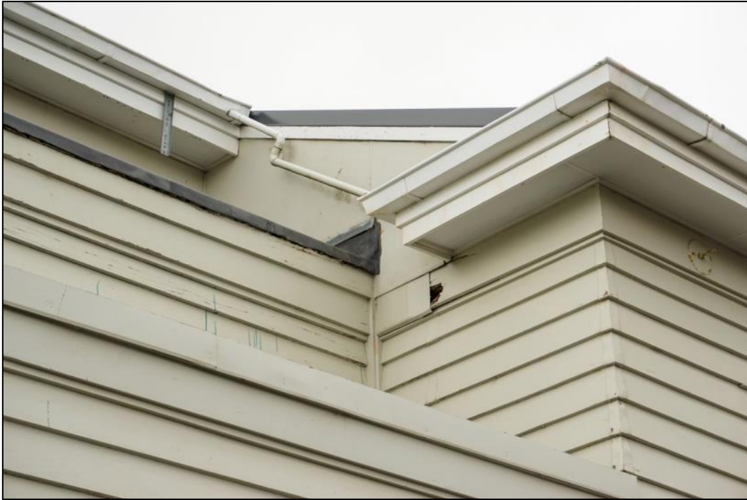
Figure 79: Detail of the wall junctions at the southeast corner of the building. The middle 'tier' (shown also below) was added at some stage. A combination of weatherproofing and roofing systems are evident. Photo: Blair Hastings – March 2017.
