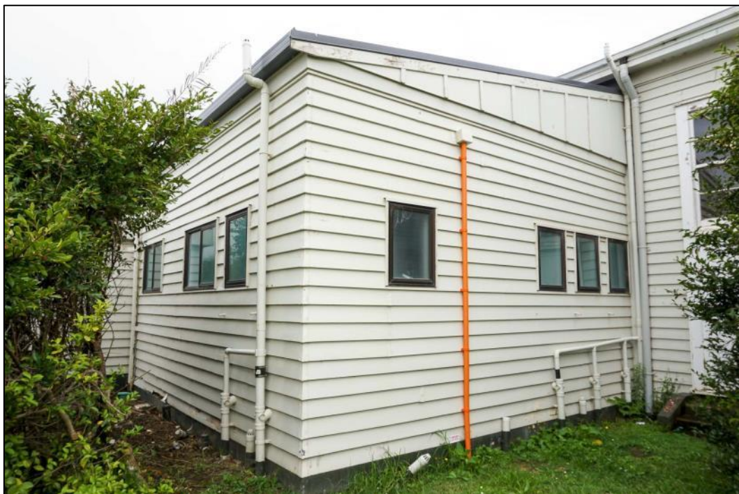
Figure 86: The southwest corner of the originally flat-roofed 'apron' that extends the building to the west and the north. The newly pitched roof is evident, as is also aluminium windows and a mix of modern plumbing fixtures. Photo: Blair Hastings – March 2017.
