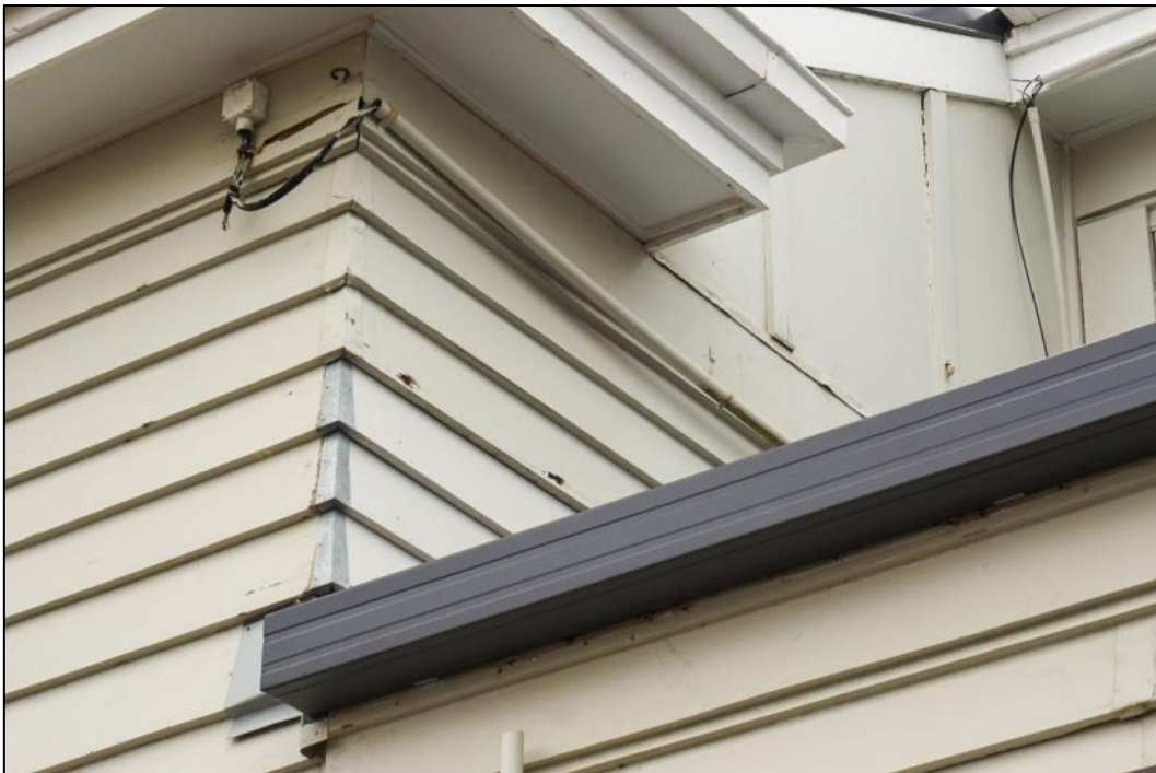
Figure 78: Detail of the wall junction above the porch (referring to the photo above in figure 77). Galvanised soakers have been fitted to address a problem. They remain unpainted. Further timber rot is still evident. Photo: Blair Hastings – March 2017.
