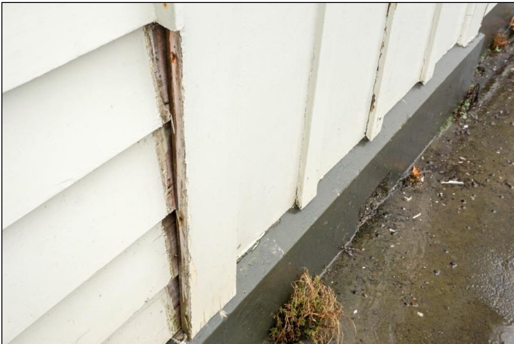
Figure 91: External trim detail – scribe missing – common of other ingress defects across the exterior shell. Photo: Blair Hastings – March 2017.
