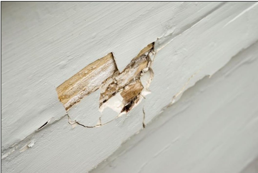
Figure 95: Paint failure – perhaps due to water ingress – indicative of many similar problems across the exterior shell. Photo: Blair Hastings – March 2017.
