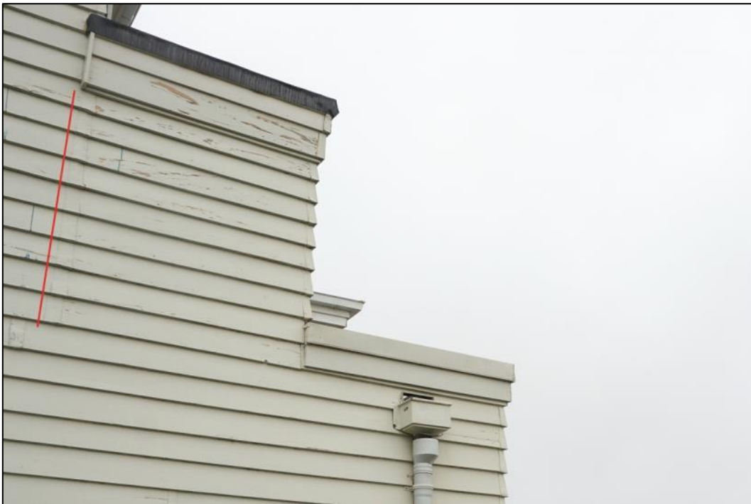
Figure 80: Detail of the southeast corner of the south elevation of the building. The red line shows tin jointers where the second 'tier' was added. Photo: Blair Hastings – March 2017.
