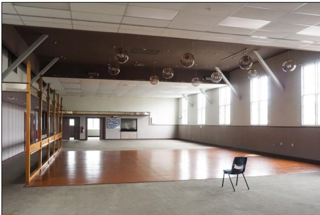
Figure 100: Interior – highly modified and compromised. Almost no original fabric evident other than most of the window and door joinery and the ceiling buttressing, encased in timber. Photo: Blair Hastings – March 2017.
