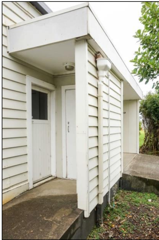
Figure 71: Non-original entrance porch to the west elevation. Both ramps have been added at some stage. Photo: Blair Hastings – March 2017.
