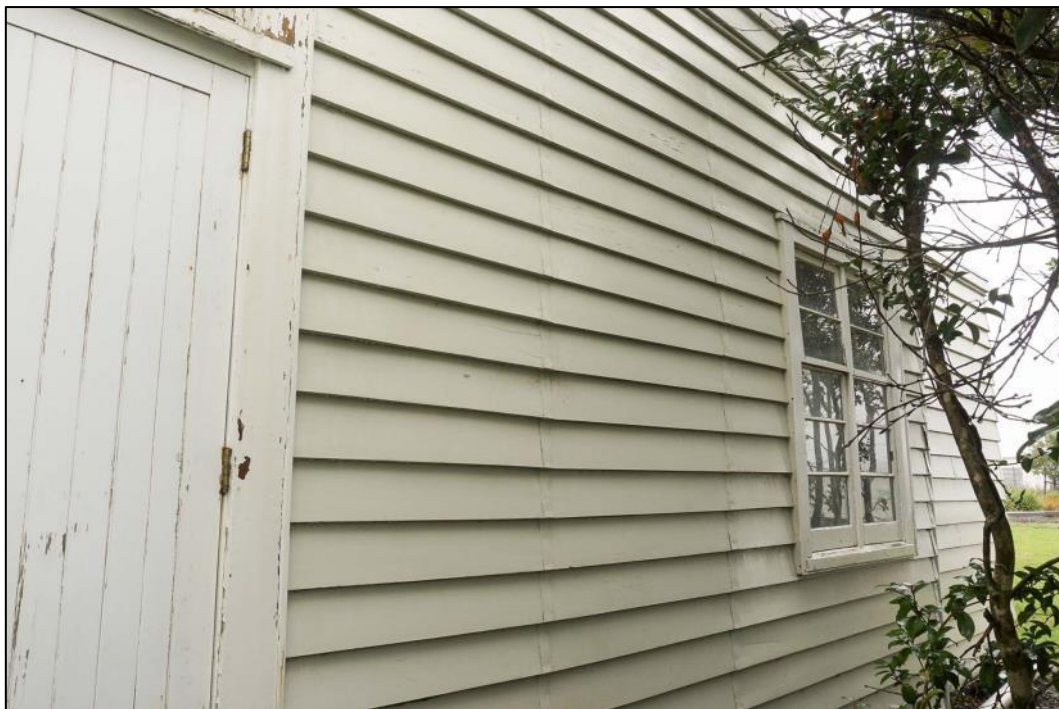
Figure 85: Southern section of the west elevation and to the right of the window the toilet block, built circa 1940. The filled in door into the former dressing room is evident (to the left of the window). The photograph shows the general disrepair of the building fabric. Photo: Blair Hastings – March 2017.
