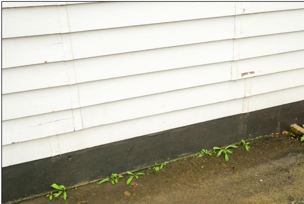
Figure 75: Southern section of the east elevation – the outline of the original door and steps into the Barber's Shop can be seen in the tin weatherboard jointers – refer also below. Photo: Blair Hastings – March 2017.
