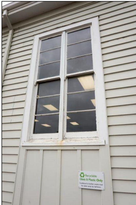
Figure 87: Hung windows with horned sashes. Transoms match the style of the both the era, and of the casement windows used within the apron annex of the building – as seen in figure 88 below. Photo: Blair Hastings – March 2017.
