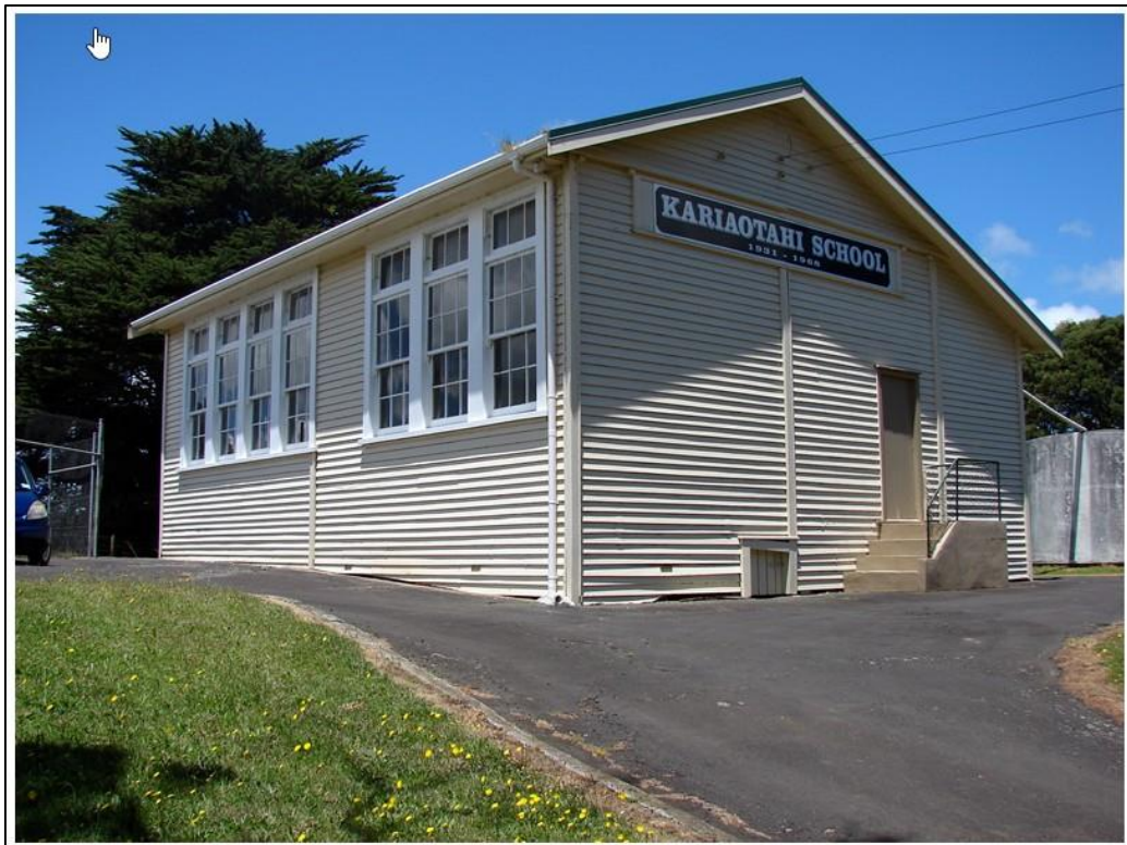
Figure 8: The Kariaotahi School Hall - built 1931 in a generic rectangular gable ended style. Timber framed, timber weatherboards, hung windows and an iron roof. The building exhibits a robust simplicity to the form – much of which is similar to the Institute building. https://www.waikatodistrict.govt.nz/recreation/community-halls .
