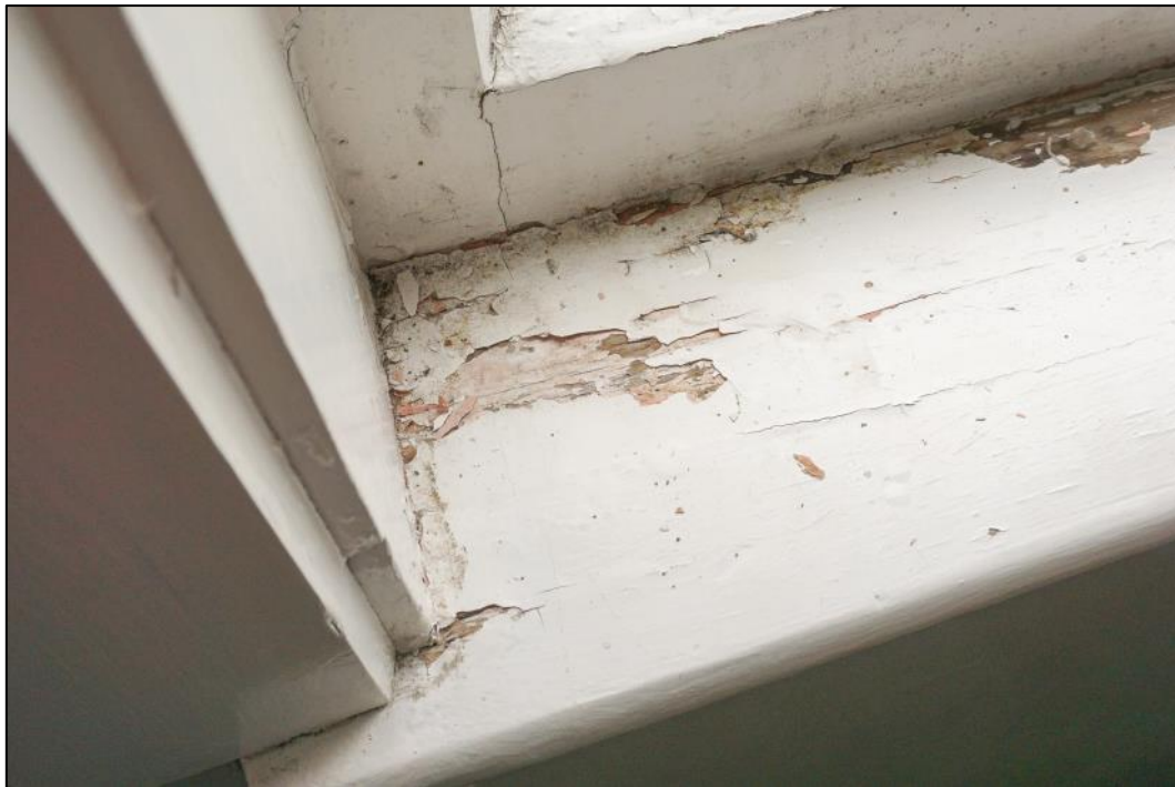
Figure 89: Internal window sill detail – showing signs of wear and possible water ingress. Photo: Blair Hastings – March 2017.
