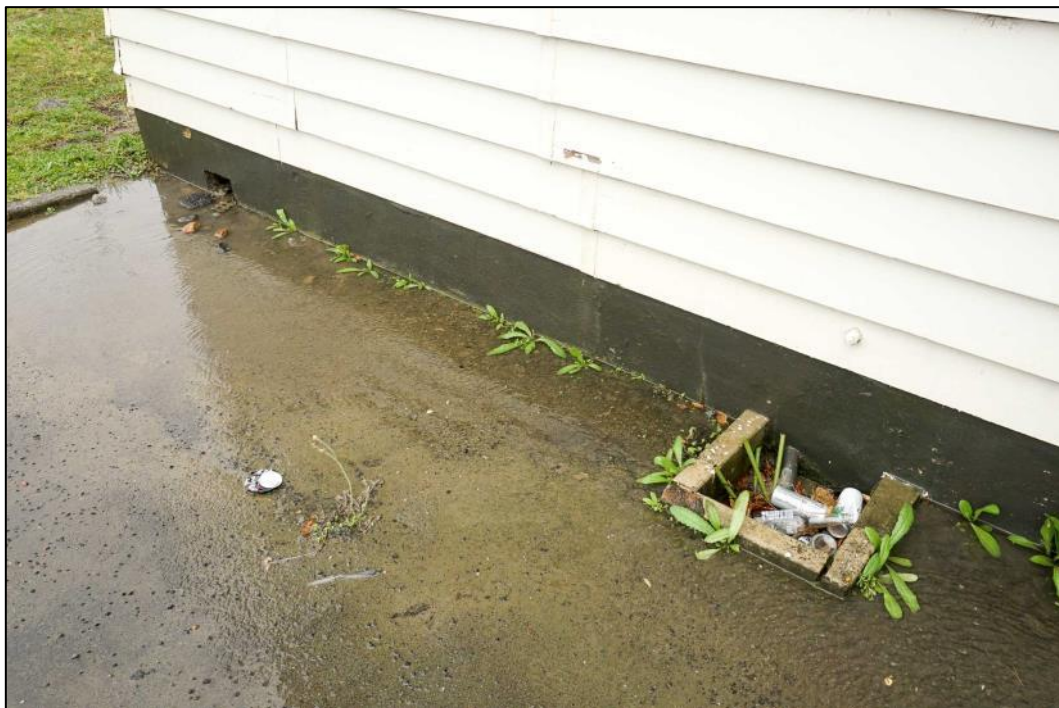
Figure 90: Southern end of the east elevation – rain water ponding against the building. Photo: Blair Hastings – March 2017.
