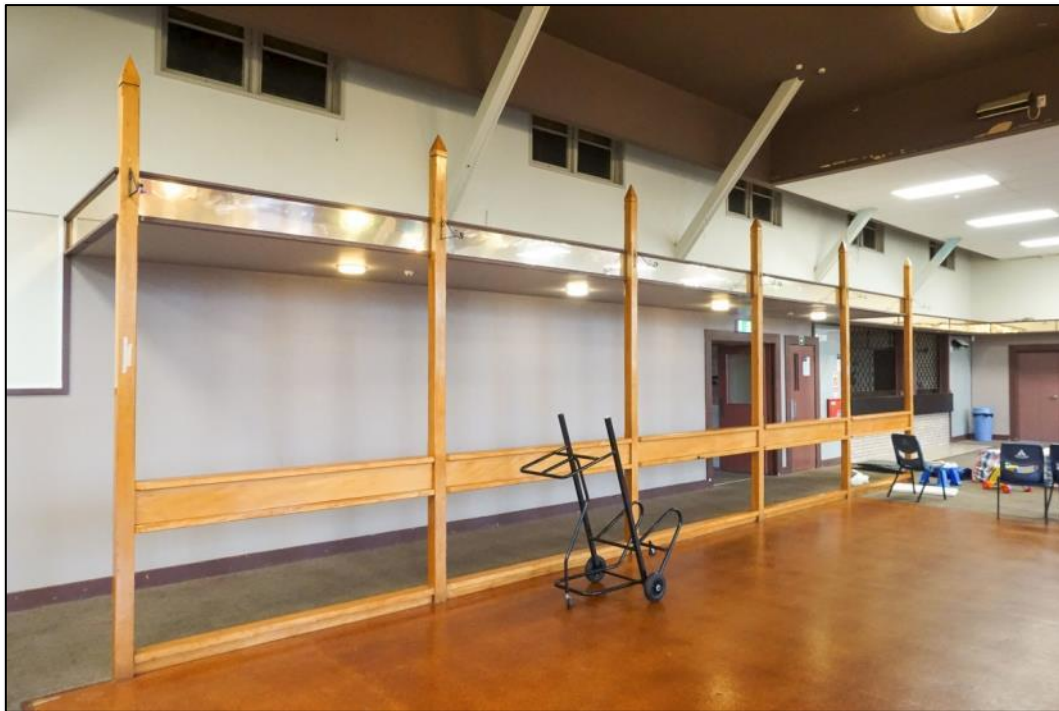
Figure 99: Interior – highly modified and compromised. High level windows mirror hung windows on the opposite (east) elevation but are now wholly internal facing as the re-pitched apron roof springs from above the window heads. Photo: Blair Hastings – March 2017.
