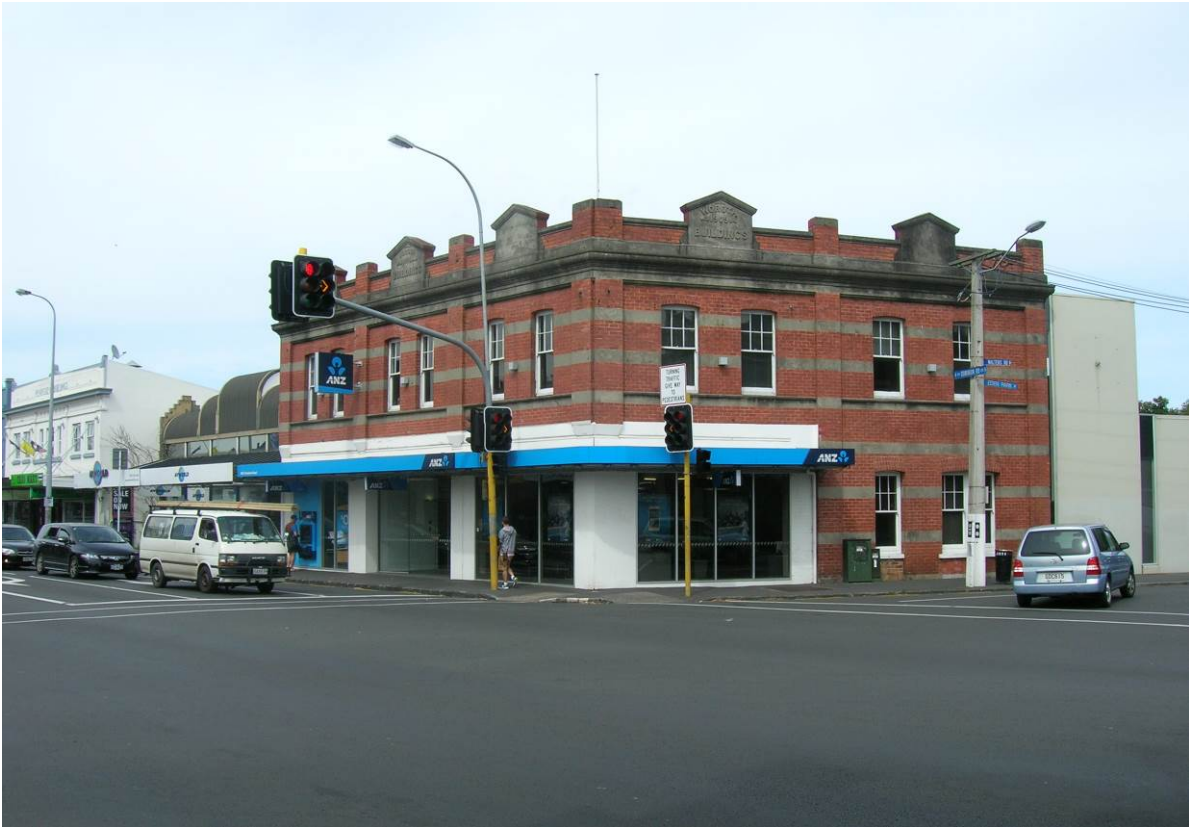
▲ Worota Building, 227-231 Dominion Road / cnr. Walters Road Mt Eden, 1907
