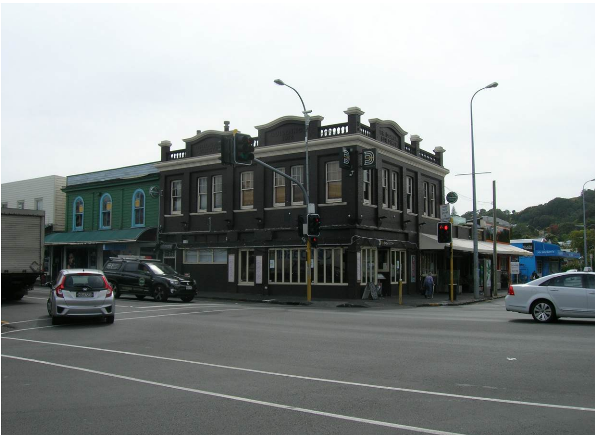
▲ Bridgeman Building, 234 Dominion Road / cnr. Valley Road Mt Eden, 1912
