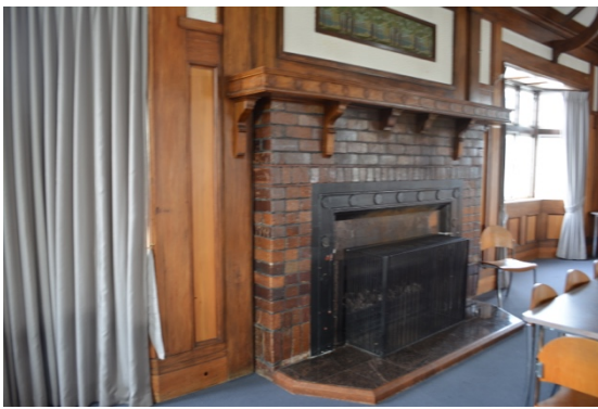
Figure 30: The distinctive glazed brick fireplace with decorative timber mantle (THS, 2016).
