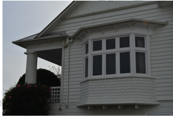
Figure 27: One of the bow windows on the south elevation with shingle base and timber modillions (THS, 2016).
