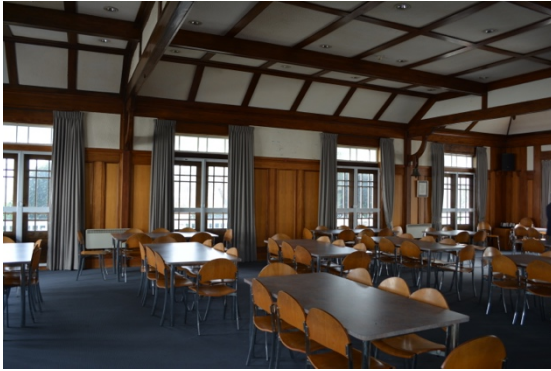
Figure 28: The dining hall, looking towards the west wall, showing the decorative timber panelled walls and beam and batten ceiling. Note the secondary glazing units fitted to the French doors (THS, 2016).
