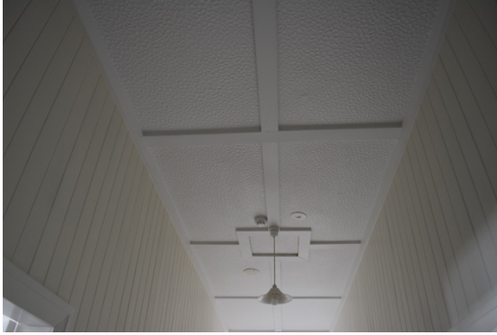
Figure 21: Board and wide batten ceilings, arranged in a crisscross pattern, and timber tongue and groove wall panelling (THS, 2016).
