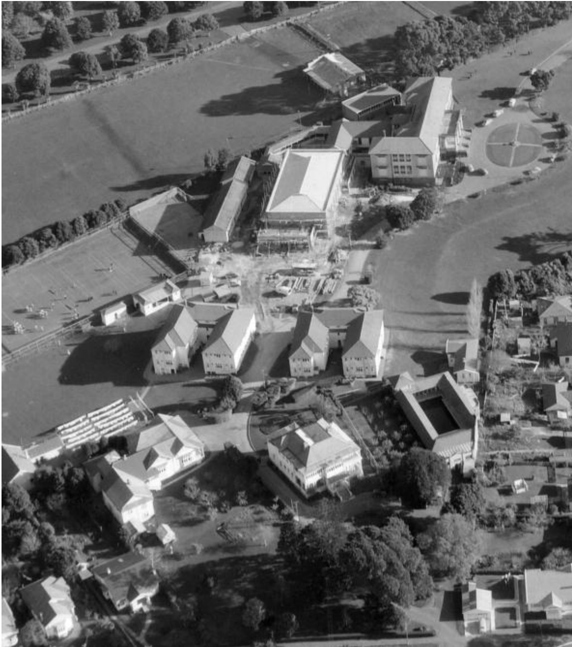
Figure 56: A close-up aerial image (Figure 46) of St Cuthbert's College in 1955, the construction of Clouston Hall. The rear elevations of Dunblane House, Elgin House and the Refectory are visible.
