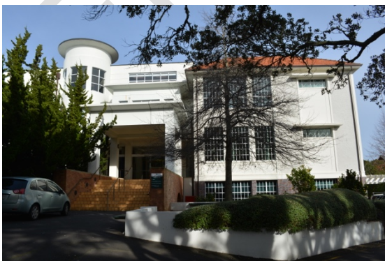
Figure 5: East elevation of the Robertson Building showing the Information Centre extending to the rear (THS, 2016).
