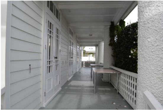
Figure 26: Looking along the porch on the west (front) elevation, showing a series of French doors and structural columns (THS, 2016).
