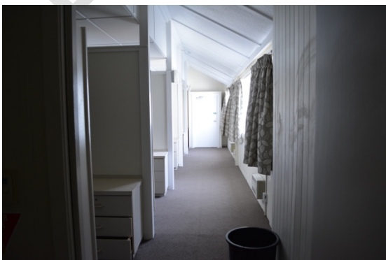
Figure 19: Interior view of the wings showing dormitory cubicles leading off a corridor that was originally built as an open-air verandah/balcony (THS, 2016).
