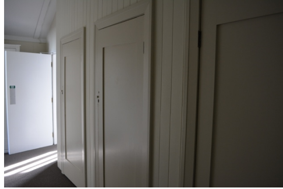
Figure 22: Traditional timber panelled doors with bevelled architraves. Modern fire-proofing doors (left) have been added in both houses (THS, 2016).
