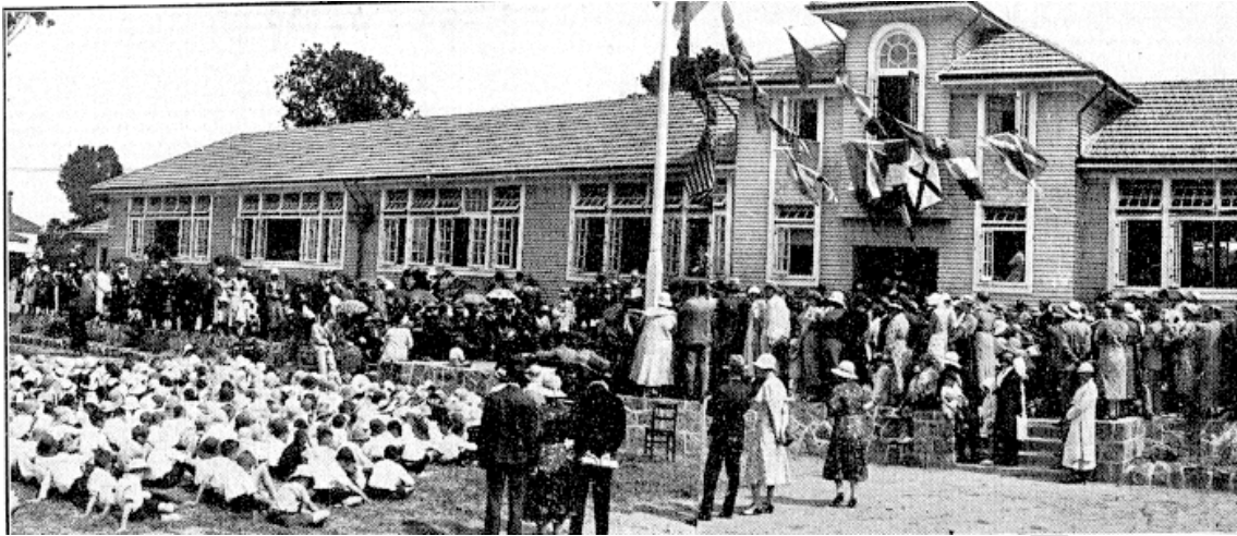
Figure 92: The Parnell Infant School, designed by A. B. Miller, following its completion in 1933. Note the expanses of windows along the principal façade, similar to the Robertson Building ( Papers Past ).
