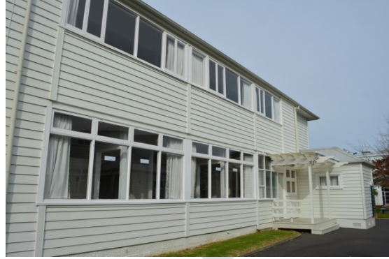
Figure 18: North elevation of Elgin House showing the infilled balconies, originally designed to provide open-air sleeping (THS, 2016).
