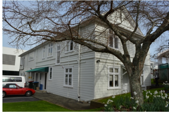
Figure 25: East (rear) and part north elevations. This portion of the building is utilised as residential accommodation (THS, 2016).
