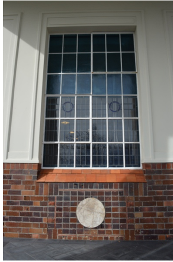
Figure 8: An original window featuring leaded and stained glass with tile sill (THS, 2016).
