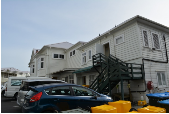
Figure 24: South elevation, viewed from the east (THS, 2016).
