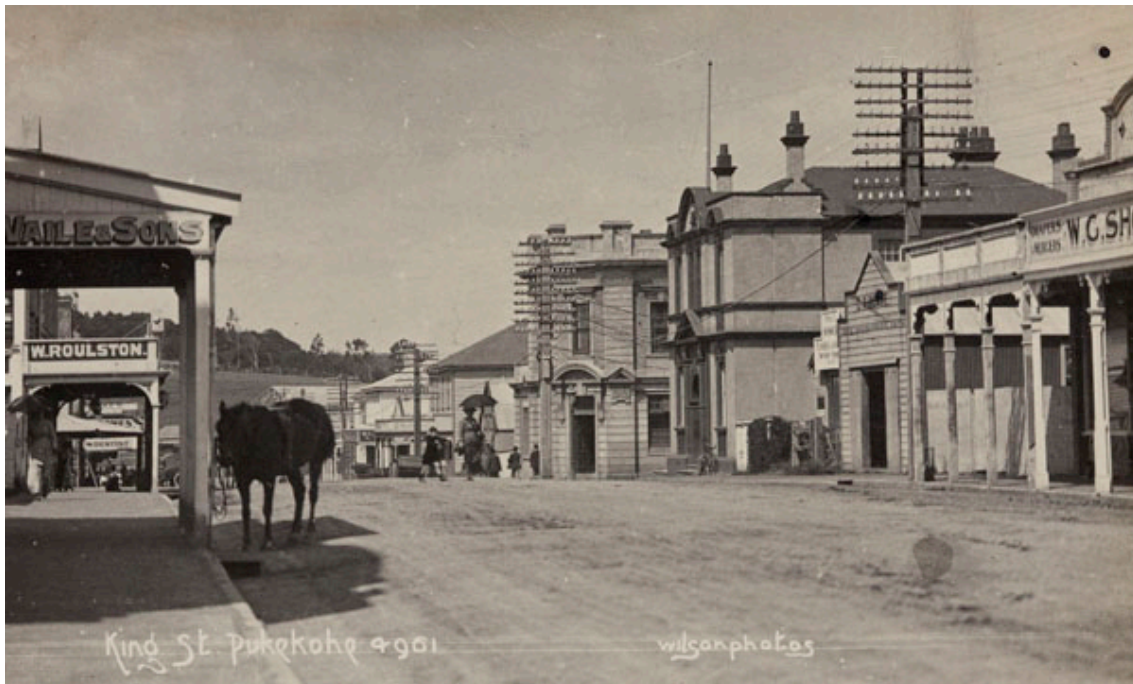
Figure 22: Looking east along King Street, Pukekohe, c.1915. Note the larger masonry Post Office and Bank of New Zealand buildings set amongst smaller timber structures (South Auckland Research Centre, FRA: I, 5 / Footprints 04843, reproduced by courtesy of Pukekohe Library).
