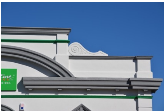
Figure 10: Stepped parapet and deeply profiled open segmental pediment with decorative plastered scrolls and corbels.
