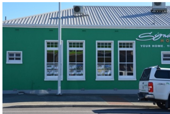
Figure 11: A series of double-hung sash windows with multi-glazed top lights, and smaller aluminium units on the south elevation.
