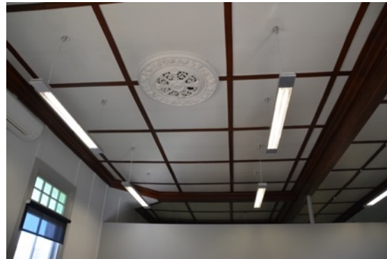
Figure 13: Timber beam and batten ceiling with decorative ceiling "rose".
