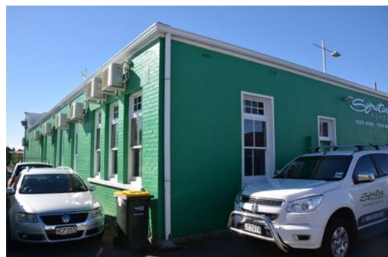
Figure 7: Part west (rear) and north elevations.
