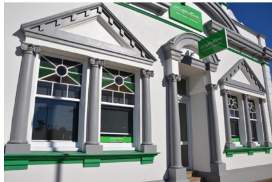
Figure 9: Central entry and decorative timber sash windows, Ionic columns and profiled pediments.
