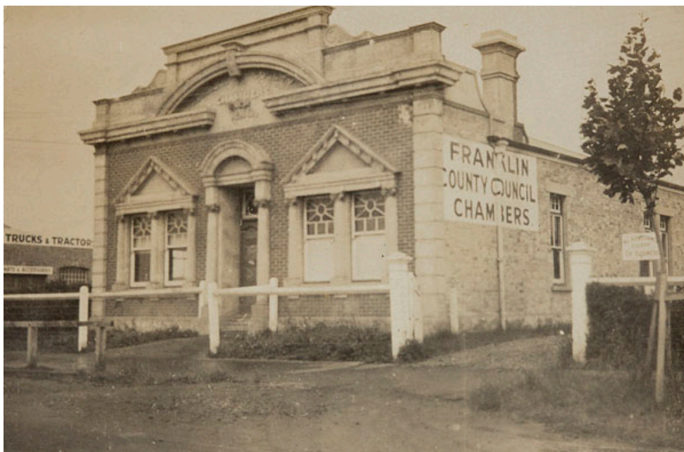
Figure 21: Exterior view of the Franklin County Council Chambers, 1924 (South Auckland Research Centre, Footprints 03223).
