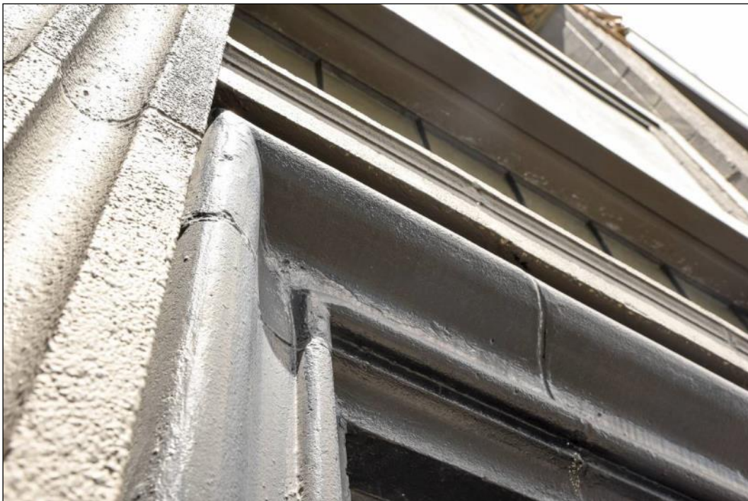
Figure 77: Close-up of the entrance way / door frame on New North Road. The photograph evidences the generally good condition of the entire façade - October 2016. Photograph: Blair Hastings.
