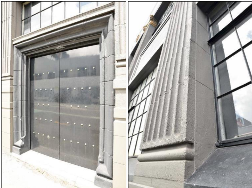
Figure 75: Close-up of the original entrance way / door frame (left) – the door has most likely been changed. Close-up of the base of one the square fluted columns on the main street elevation showing the 'restraint' or stripped back classical detailing (right) - October 2016. Photograph: Blair Hastings.
