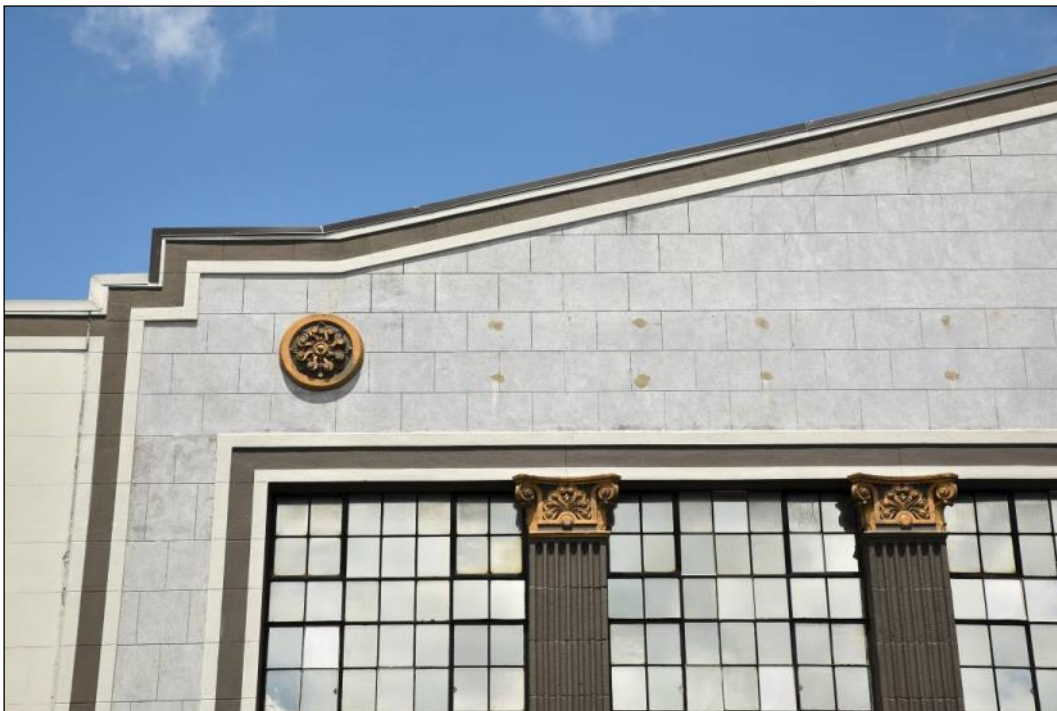
Figure 70: Close-up photograph of the both the junction formed by the 1947 extension to the original street façade and part of the gable end of the original factory building. The restrained but high contrast paint scheme is well specified to highlight the strong geometric forms of the stripped back classical façade. Patching in the rendered façade is clearly evident where the lettering was removed between the decorative rosettes - Photograph: Blair Hastings.
