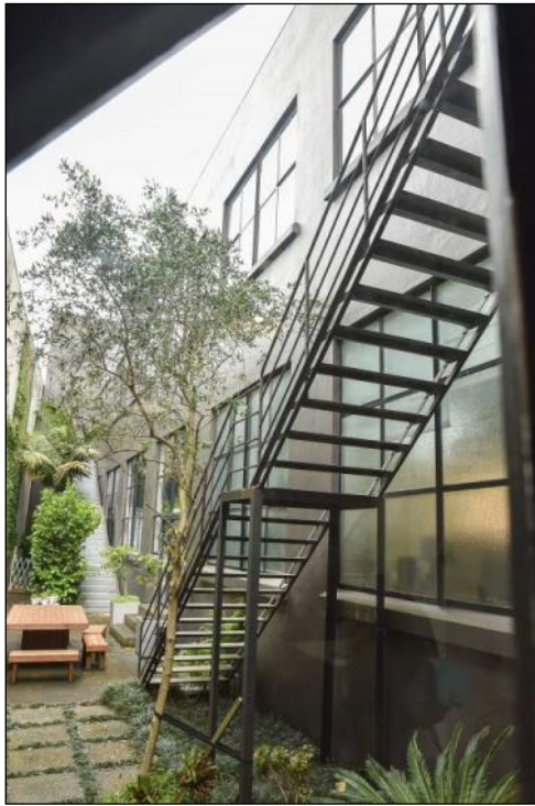
Figure 85: The 'courtyard' to the rear of the 1947 extension showing the west façade of the original 1929 factory building. The escape stairs were part of the aforementioned extension built in the 1940s. The steel windows replaced the original windows sometime between 1957 and 1963 – October 2016. Photograph: Blair Hastings.
