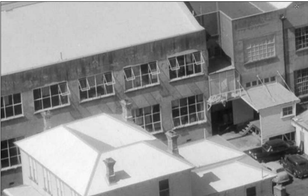
Figure 59: March 1963. Bridgens and Company Ltd, New North Road, Auckland. Whites Aviation Ltd :Photographs. Ref: WA-59525-F. Alexander Turnbull Library, Wellington, New Zealand. http://natlib.govt.nz/records/22325512 . Note the 1957 photograph above – the windows along the west elevation have been changed. Full image previous - Extract above.
