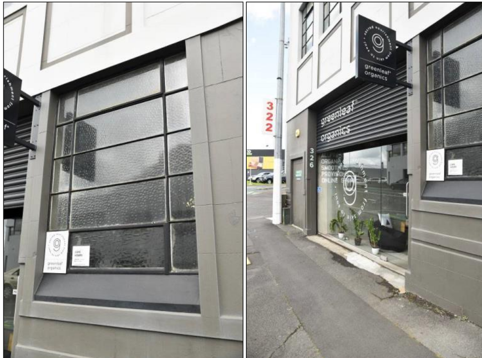
Figure 76: Close-up of the original steel window with opening top sash in the 1947 section of the main building façade (left) The entrance to Greenleaf Organics Café showing the new glazed 'shop-front' and street signage but generally otherwise intact original façade (right) - October 2016. Photograph: Blair Hastings.
