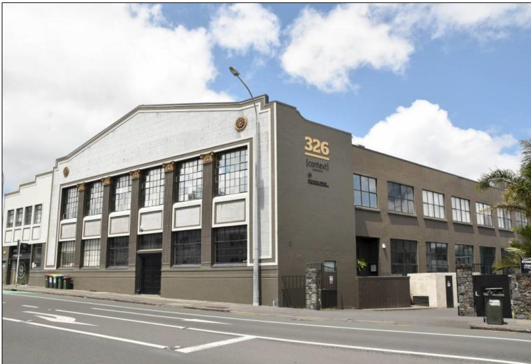
Figure 68: The building's street and western façades October 2016 – Taken from the northern footpath on New North Road – looking southeast. The street façade is largely intact. Western façade contains steel window changes sometime between 1957 and 1963. The northern most window bay on the ground floor has been removed to accommodate the principal entrance into the shared office space. Photograph: Blair Hastings.
