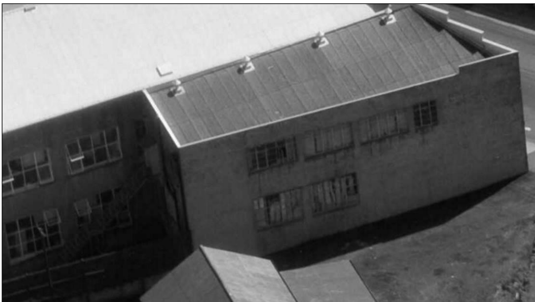
Figure 61: March 1963 . Kiwi Bacon Company Ltd industrial premises, Auckland. Whites Aviation Ltd :Photographs. Ref: WA-59540-F. Alexander Turnbull Library, Wellington, New Zealand. http://natlib.govt.nz/records/22860837 . Extract. Full image above.
