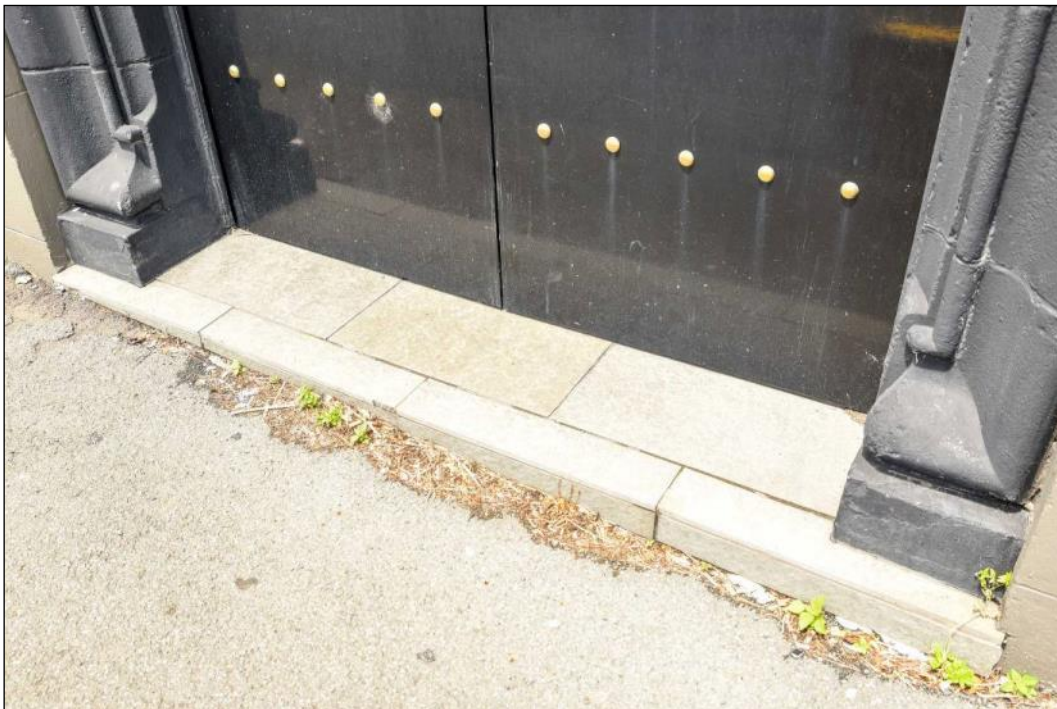
Figure 82: Close-up of the original entranceway – the door sill tiling appears to have been modified and the door is new – or it is possible that the original has been over-clad - October 2016. Photograph: Blair Hastings.
