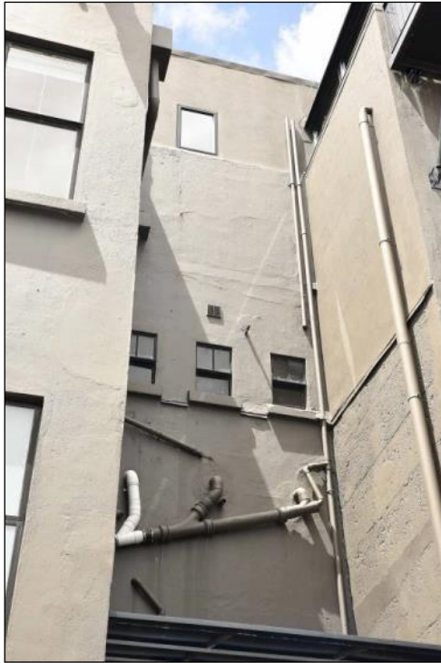
Figure 83: Close-up of the toilet bay at the rear of the original factory building. The three first floor windows in the centre of the photograph may be original – there is a faint plaster line above them which may indicate the roofline of the original block. The window above is within the extension to the rear, subdivided and strata titled as a separate and independent property. The subject site / building ends at the underside of the structural ceiling to the first floor toilet. October 2016. Photograph: Blair Hastings.
