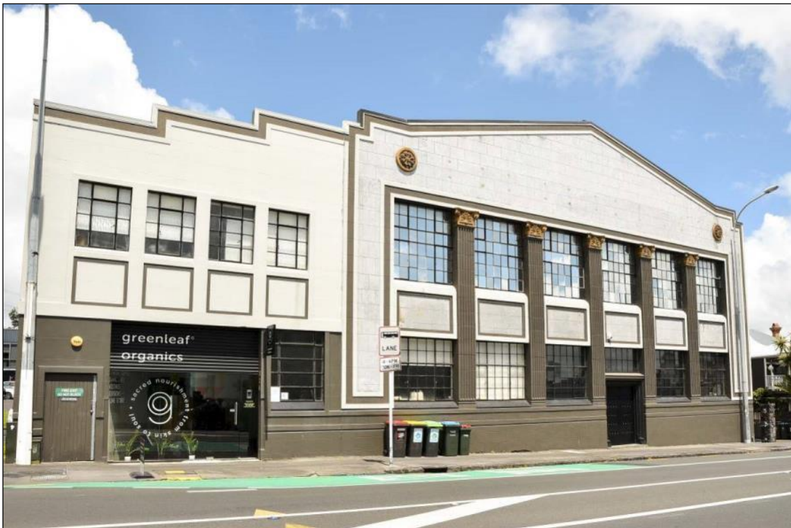
Front elevation of the former factory building as seen from the northern footpath on New North Road
