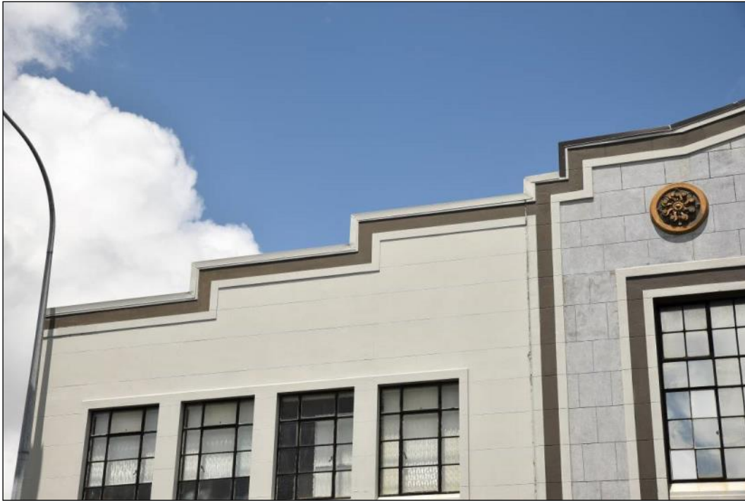
Figure 69: Close-up photograph of the junction formed by the 1947 extension to the original street façade. The stripped back classical detailing is in evidence either side of the junction – the later addition subtly in scale and form - Photograph: Blair Hastings.
