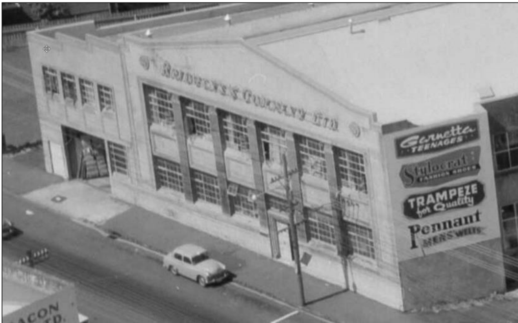
Figure 58: March 1963. Bridgens and Company Ltd, New North Road, Auckland. Whites Aviation Ltd :Photographs. Ref: WA-59525-F. Alexander Turnbull Library, Wellington, New Zealand. http://natlib.govt.nz/records/22325512 . Full image previous - Extract above.
