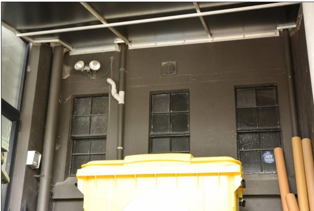
Figure 84: Close-up of the ground floor of the recessed toilet bay at the rear of the original factory building, in the west elevation. The three windows are likely original – October 2016. Photograph: Blair Hastings.
