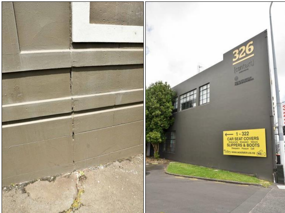
Figure 79: Close-up minor cosmetic deterioration in the main street façade – such ‘damage’ is relatively isolated and minor (left). East façade showing original steel window bays as seen on the 1947 plans (right) - October 2016. Photograph: Blair Hastings.
