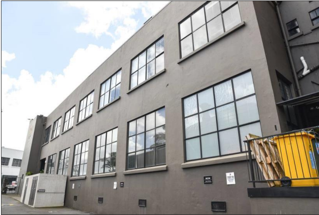
Figure 71: The west elevation October 2016 –The current steel windows were changed from the original smaller sashes sometime between 1957 and 1963. The rough openings are assumed to be original in size. The recess to the right of the photograph is to the original two storey toilet block – the windows top-right may be original. The window in the rear or south facing ‘return’ into the recess does not appear on original plans. Photograph: Blair Hastings.
