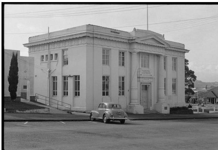
Figure 11: Borough Council offices, Dargaville, 1923 – Wade and Bartley. 63
