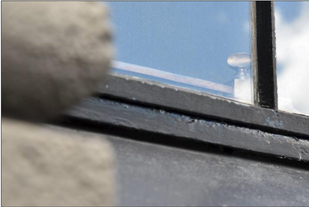
Figure 81: Close-up of the steel windows in the main street façade – showing early or original internal brass window fittings and stays - October 2016. Photograph: Blair Hastings.
