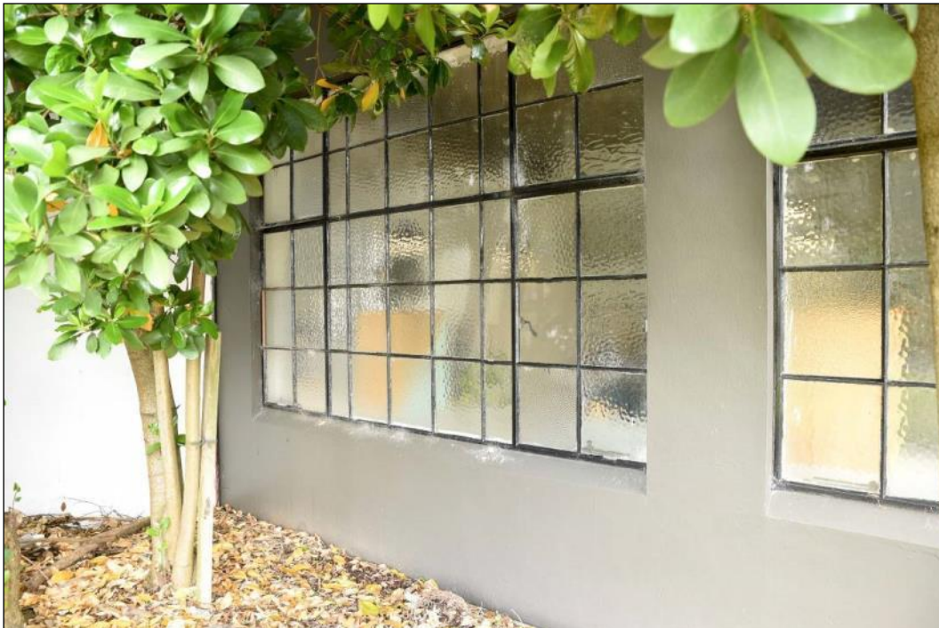
Figure 80: Close-up of the steel windows in the eastern façade of the 1947 extension (now Greenleaf Organics Café). Note the ‘simplified’ detailing to exclude proud sills when compared to the original 1929 building - October 2016. Photograph: Blair Hastings.
