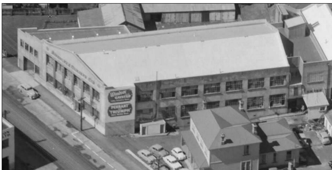
Figure 56: April 1957 . Factories on the New North Road, Auckland, New Zealand. Whites Aviation Ltd :Photographs. Ref: WA-43959-F. Alexander Turnbull Library, Wellington, New Zealand. Shows original windows along west façade and an early generator building close to the street boundary – superseded in 1984 by the AEPB transformer. http://natlib.govt.nz/records/23107313 . Extract. Full image above.
