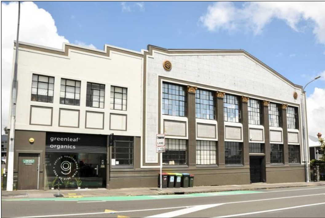
Figure 67: The building façade October 2016 – Taken from the northern footpath on New North Road – looking due south. The façade is largely intact save for the original 'Bridgens & Company Ltd' 3-dimensional lettering. Note the façade of the 1947 addition – to the left (east) of the original factory building does not align with original plans – but does align with photos (above) from 1957 – the assumption is that the plans were modified prior to construction. Photograph: Blair Hastings.
