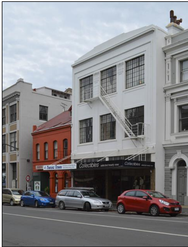
Figure 6: The Hewitt's Building, Dunedin - remodelled 1929 by architect Leslie D. Coombs. 59
