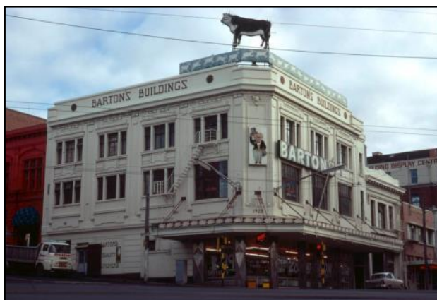
Figure 7: Barton's Building, Dunedin - 1928 by architect William Henry Dunning. 60
