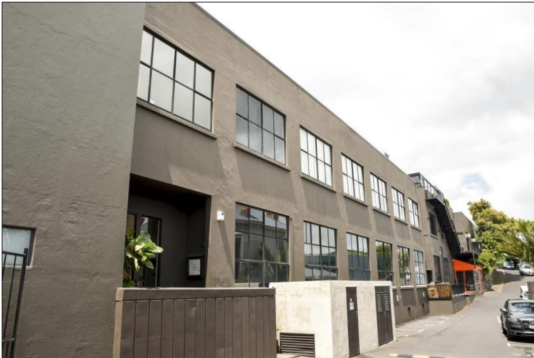
Figure 72: The west elevation October 2016. Shows the steel windows changed sometime between 1957 and 1963. The northern most window bay on the ground floor has been removed to accommodate the principal entrance into the shared office space – for which the building is now used. Photograph: Blair Hastings.
