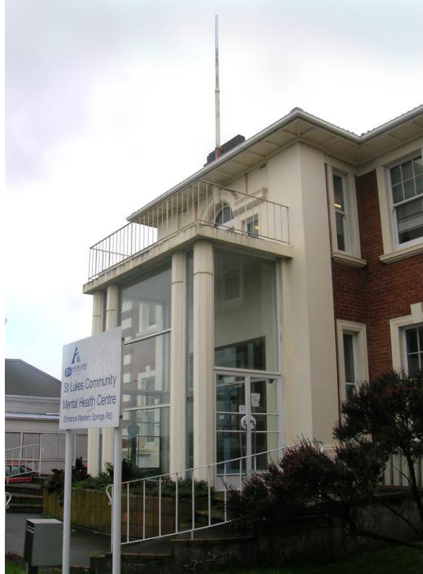
Close-up view of portico
