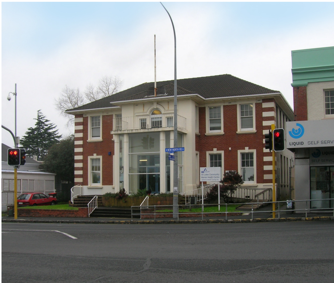
Current view, May 2016 – Salmond Reed Architects
