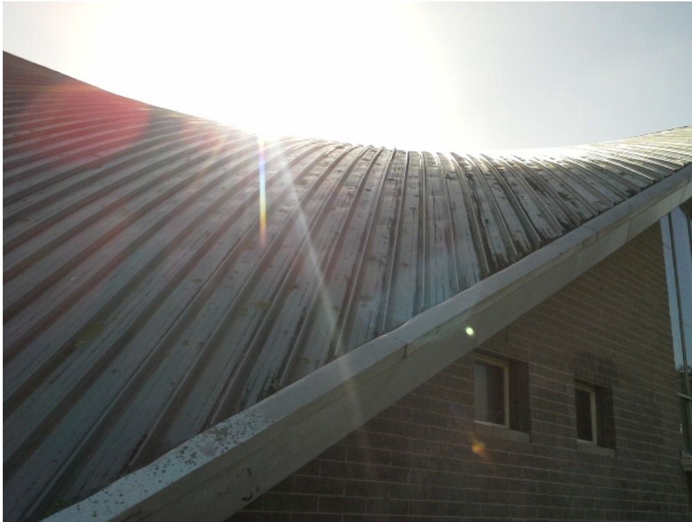
Figure 24: The detail of the hyperbolic roof. Auckland Council, July 2016.
