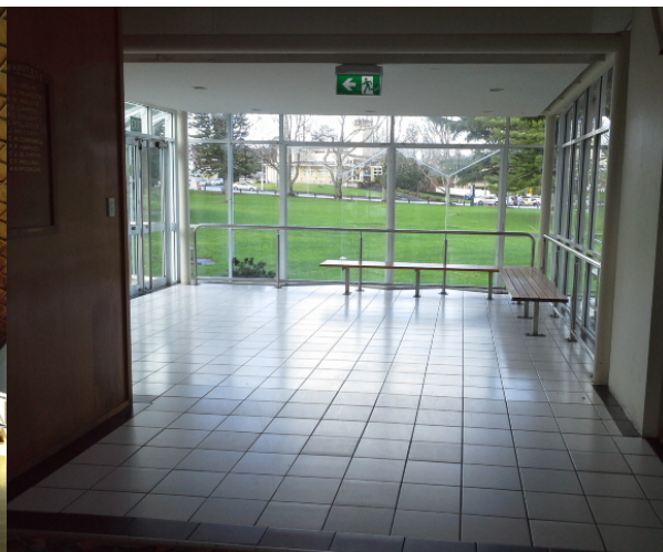
Figure 5: A later addition of the entrance lobby constructed in 1970. Auckland Council, 2016.
