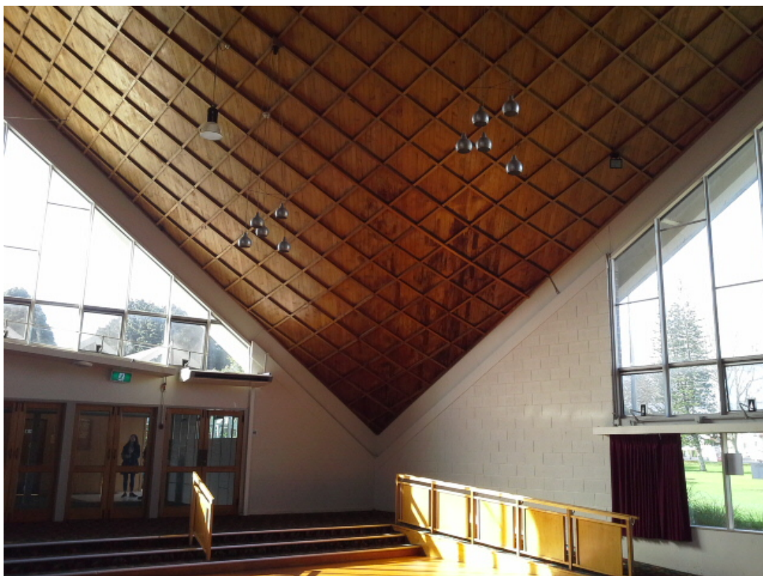
Figure 29: The timber lattice framework of ceiling of the main hall. Auckland Council, July 2016.
