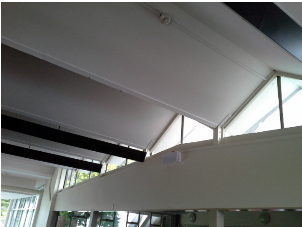
Figure 33: The zig zag ceiling of the rear building. Auckland Council, July 2016.
