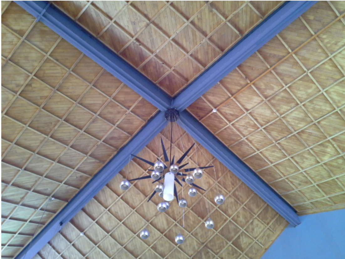
Figure 30: The timber lattice framework of the ceiling of the main hall, with the support of four steel ridge beams. Auckland Council, July 2016.
