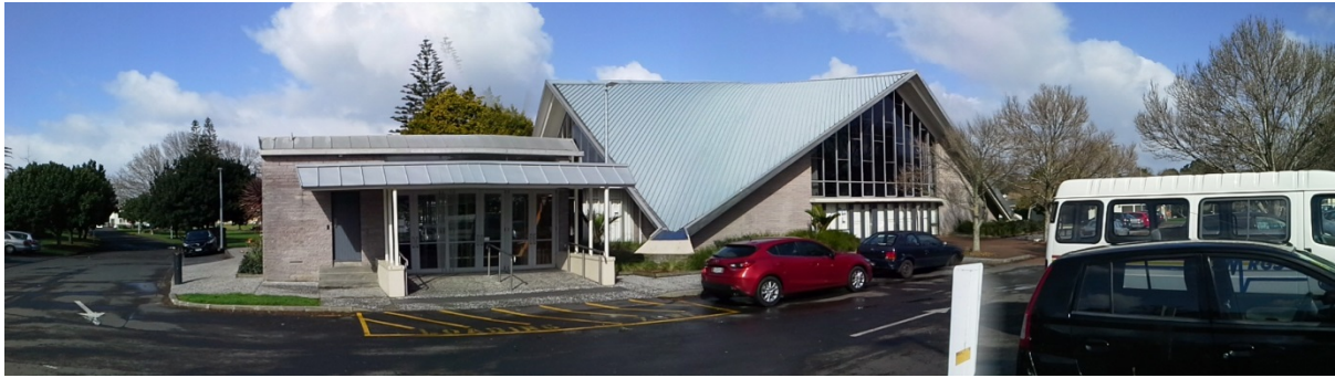
Figure 20: North elevation of Mt. Albert War Memorial Hall. Auckland Council, July 2016.
