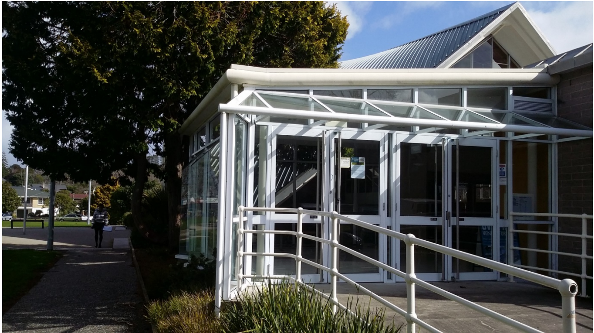
Figure 22: Later addition of the entrance hall. Auckland Council, July 2016.
