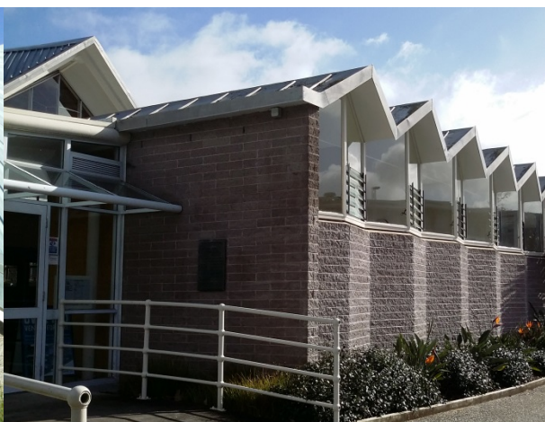
Figure 3: East annex constructed in concrete blocks and Roskill Stone, with a saw tooth roof. Auckland Council, 2016.
