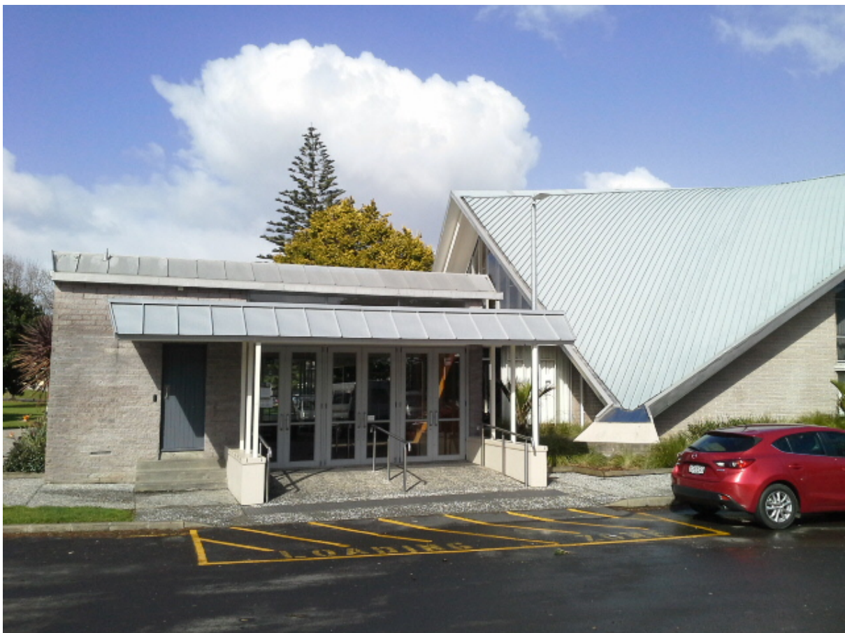
Figure 23: The addition in 2006 of standing seam zinc canopy rood in north elevation. Auckland Council, July 2016.
