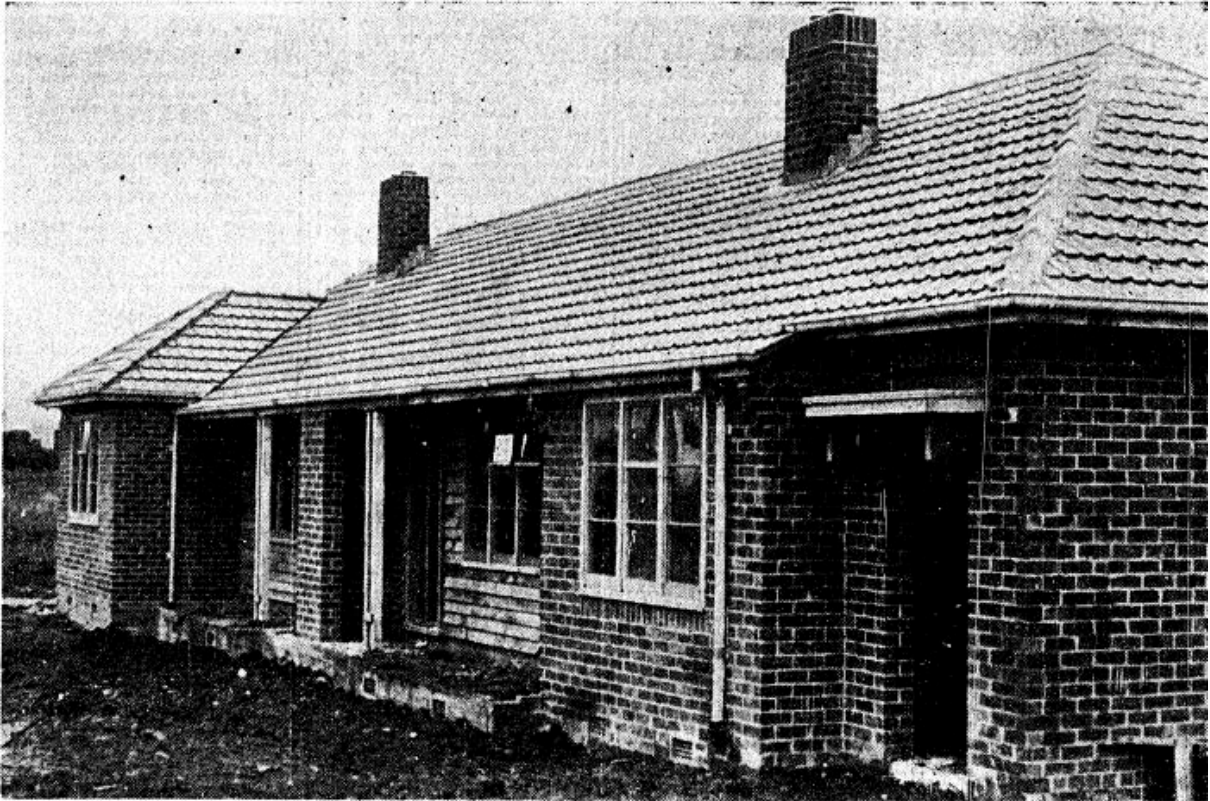
Figure 1. The pensioner flats at Pelham Avenue nearing completion in July 1938. 41
