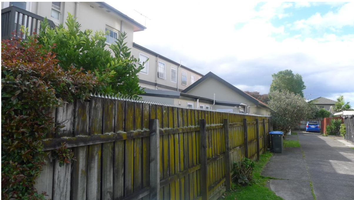
Figure 8. View down the southeastern side of the property, showing the shed, that may be the original reel shed.
