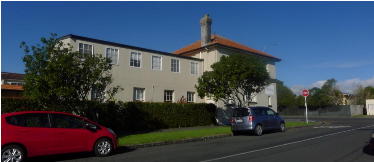
Figure 5. The rear wing as seen from Tui Street. The ground floor was part of the original construction, while the first floor was added in 1992. (David Bade, Auckland Council, 13 May 2014).
