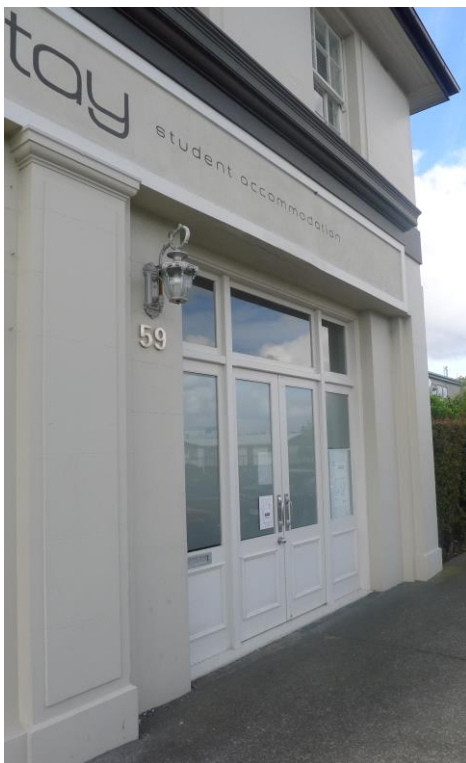
Figure 6. The former fire truck entrance is now a front doorway (David Bade, Auckland Council, 13 May 2014).
