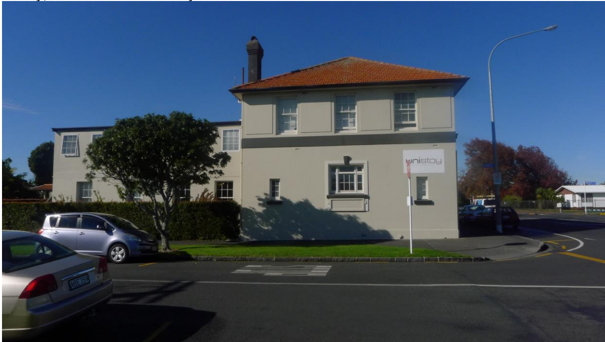
Figure 9. The Tui Street façade (David Bade, Auckland Council, 13 May 2014).
