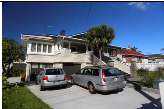
Figure 16: Front elevation, showing garage doors (Rachel Ford, May 2014)
