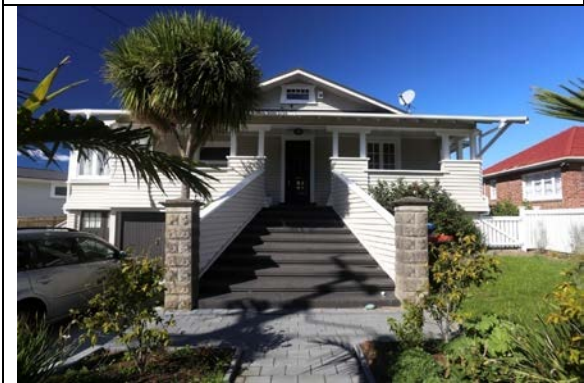
Figure 15: Front elevation, showing tapered steps and wide front verandah (Rachel Ford, May 2014)
