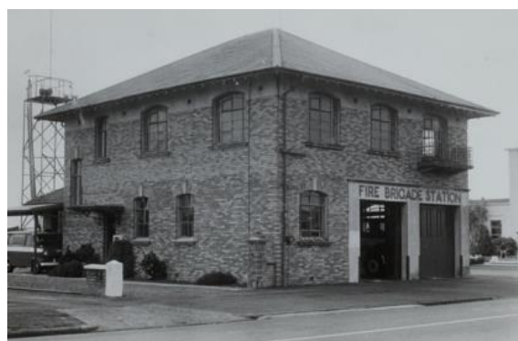
Figure 68: Pukekohe Fire Brigade Station, 1930, photograph 1987 (Auckland Libraries, Manukau Research Library, Courier collection, box 17/4, Footprints 00493).
