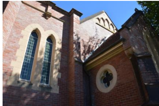
Figure 11: Showing part of the tower and sanctuary, decorated with quatrefoil and lancet windows.
