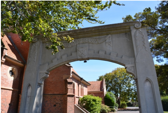
Figure 31: Showing the east side of the arch, showing its decoration.
