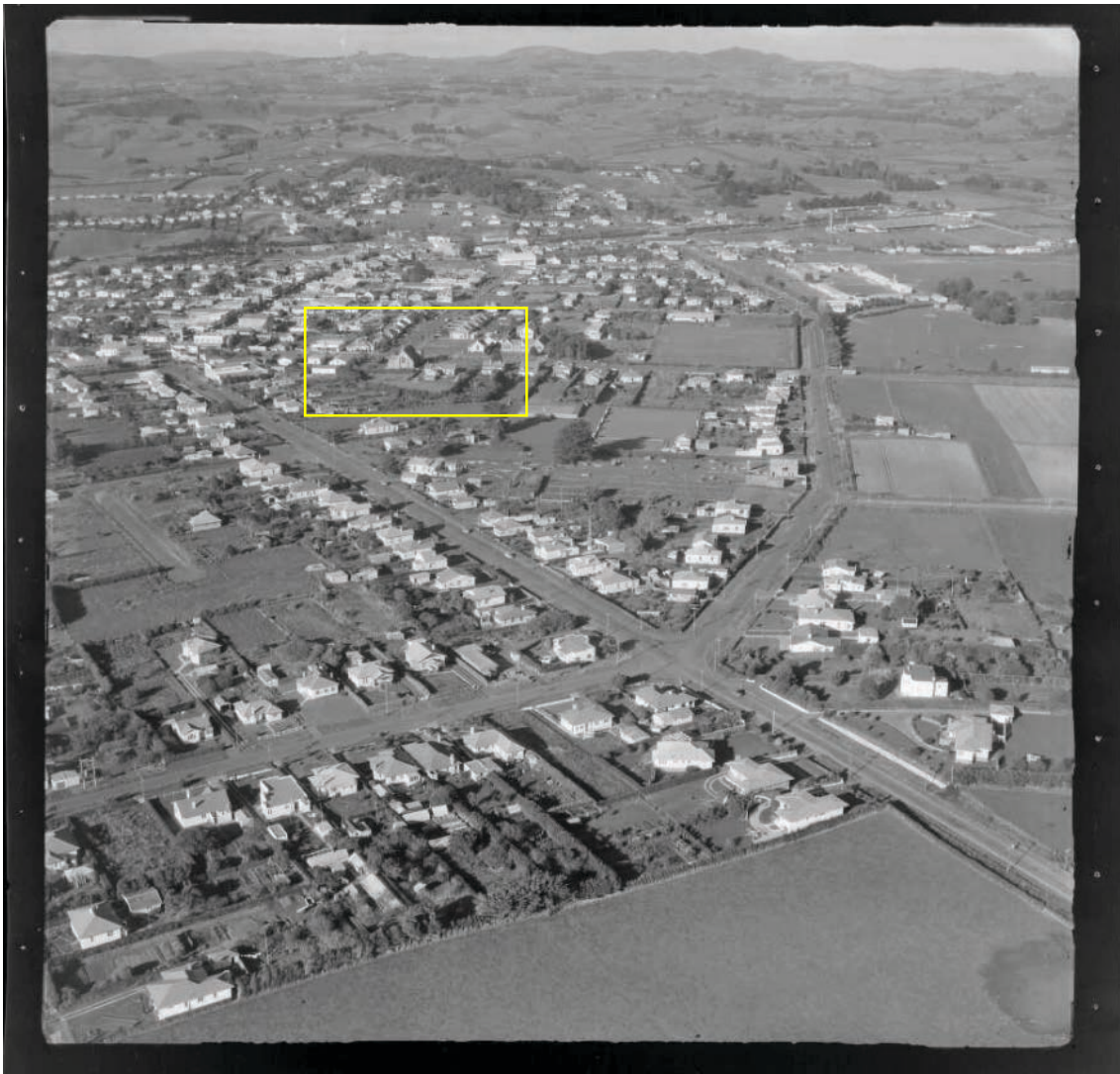
Figure 55: Aerial view of Pukekohe from the west, 22 April 1954, highlighting the church complex (WA-35464-F, Whites Aviation Collection, Alexander Turnbull Library).
