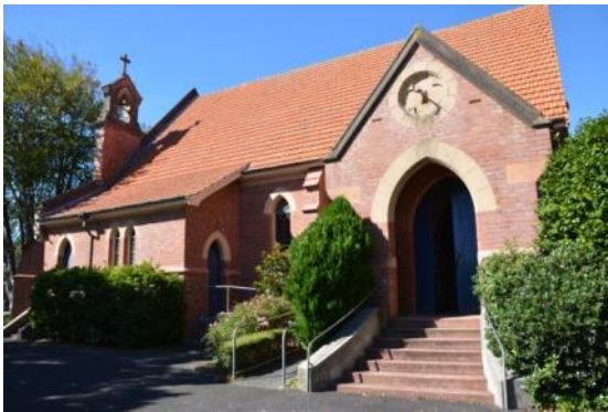
Figure 8: North elevation showing the entrance porch and belfry.
