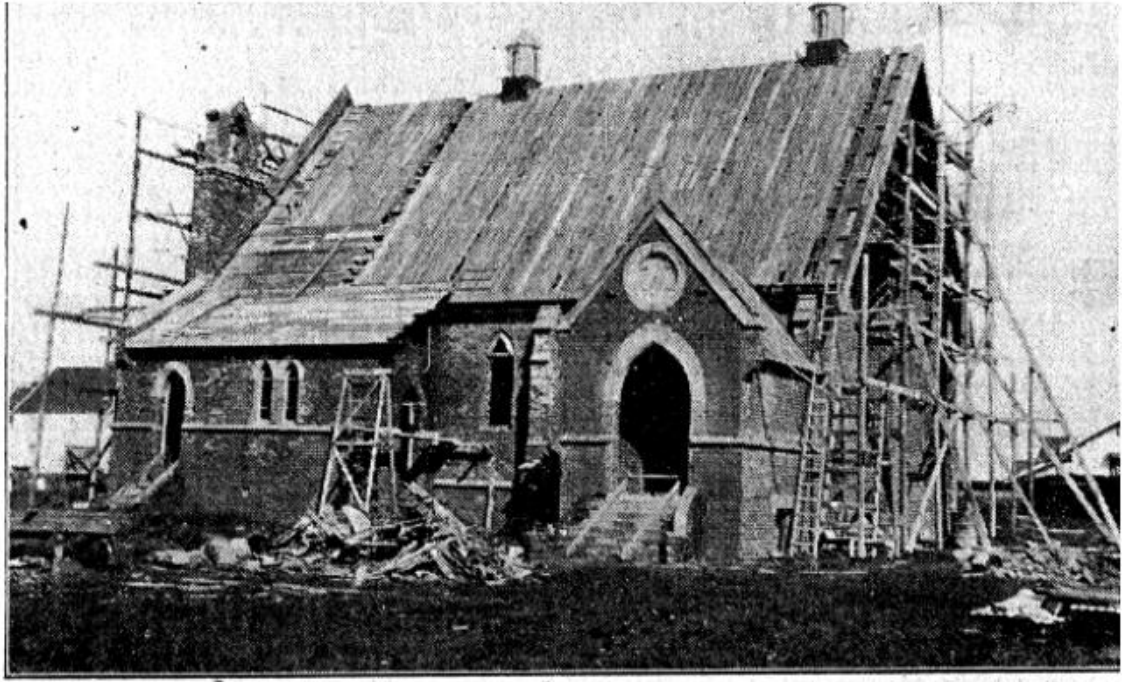
— NEW ANGLICAN CHURCH BEING ERECTED AT PUKEKOHE A photograph taken this week of the new Pukekohe Anglican Church, which is being erected at a cost of £3000. The church will have seating accommodation for 200 people.
