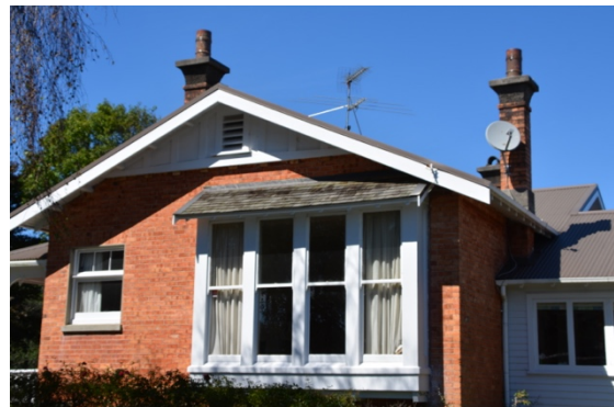
Figure 29: Sash, fixed and casement windows on north elevation.
