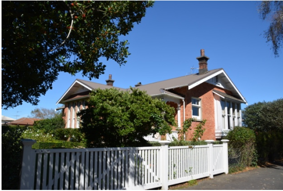
Figure 24: View of the vicarage from the driveway that divides it from the church, showing part of the east and north elevations.
