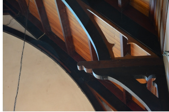
Figure 22: Decorative detailing of the single hammer-beam trusses and the colour variation of the roof timbers.
