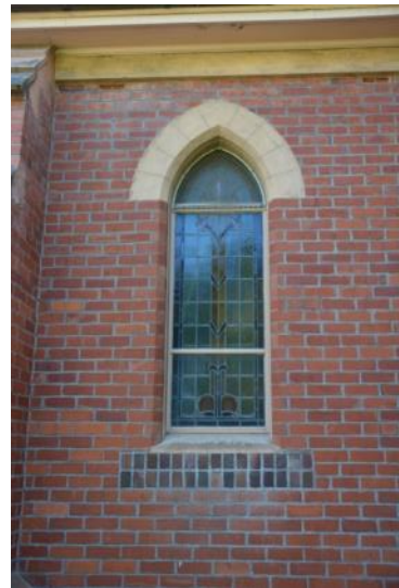
Figure 16: One of a series of smaller windows that light the nave.
