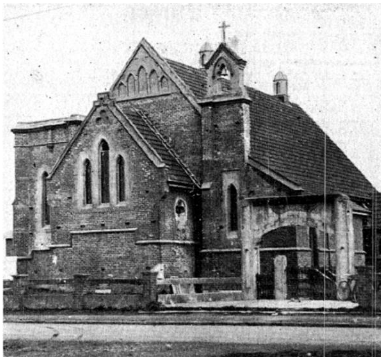
FINE NEW ANGLICAN CHURCH AT PUKEKOHE. The new Anglican Church at Pukekohe, which is now nearing completion and is expected to be ready for use in July. The church will provide seating accommodation for 200 people.
