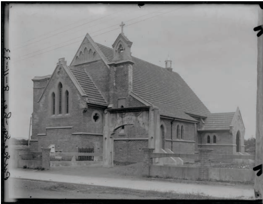
Figure 40: Showing the newly completed second St Andrew's Anglican Church with memorial arch viewed from the northeast, 8 November 1933 (Sir George Grey Special Collections, Auckland Libraries, 4-6312).
