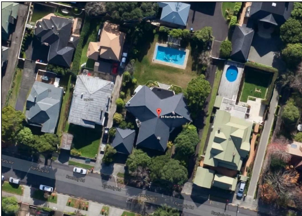
Figure 66: Current aerial photograph of the site – Imagery Copyright Google, Map data 2016.
