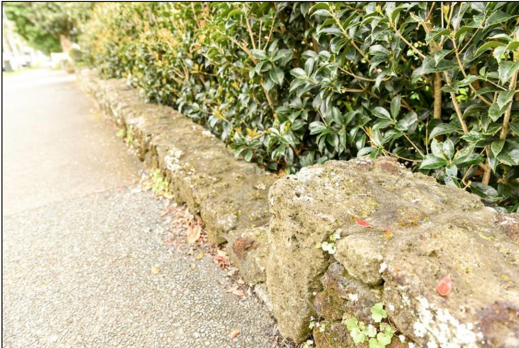
Figure 65: The site October 2016 – Looking at the front nib wall. Photographs below from 2008 show a taller, not-stepped (and probably dry-stone) volcanic stone wall. The 'remainder' may or may not early or original. Photograph: Blair Hastings.
