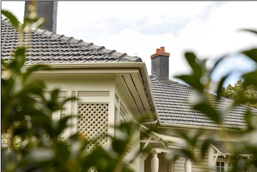
Figure 56: The site October 2016 – Looking north – at the two remaining chimneys, the Marseille styled tiles, the corner privacy and shade screens, and the ventilated timber eaves . Photograph: Blair Hastings.
