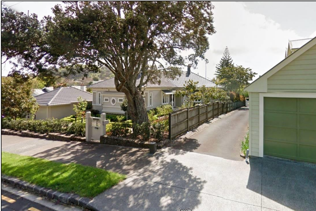
Figure 45: Site context – Looking north at the subject site – the garage in the foreground is at 83 Ranfurly Road. Photo: Google Maps October 2015.
