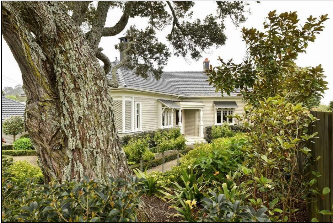
Figure 49: The site October 2016 – Looking north - at the front and east elevations of the house. Photograph: Blair Hastings.
