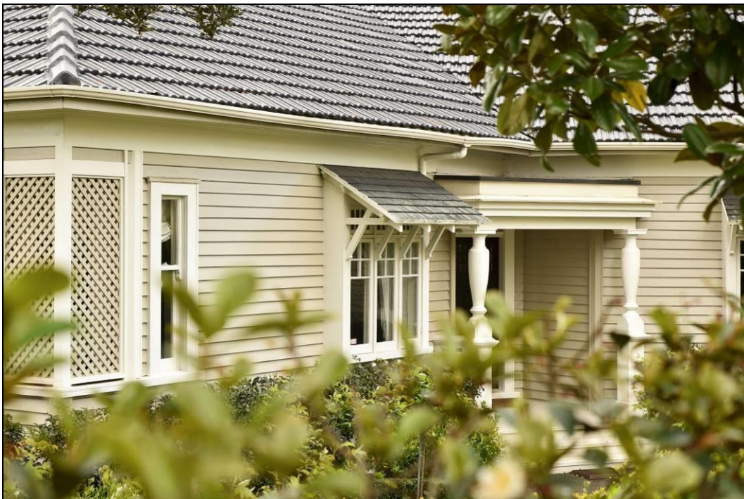
Figure 58: The site October 2016 – Looking north – at the east elevation of the house, showing the flat-roofed porch with the turned timber columns, the timber window awning and both cottage style casement and villa hung windows. Photograph: Blair Hastings.
