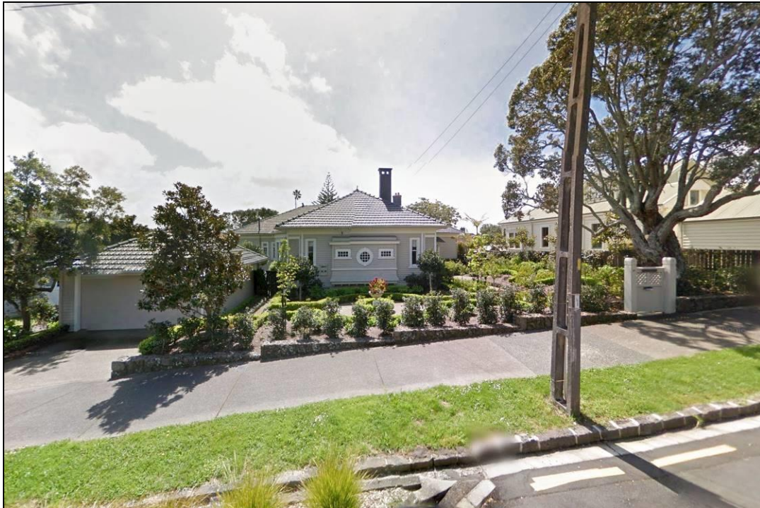
Figure 46: Site context – Looking north north-east at the subject site. Photo: Google Maps October 2015.
