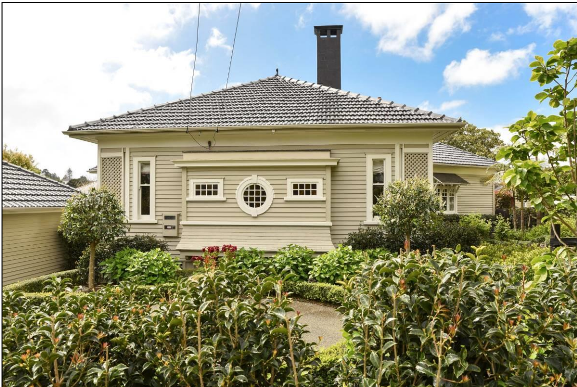
Front elevation of the residence as seen from the northern footpath on Ranfurly Road
