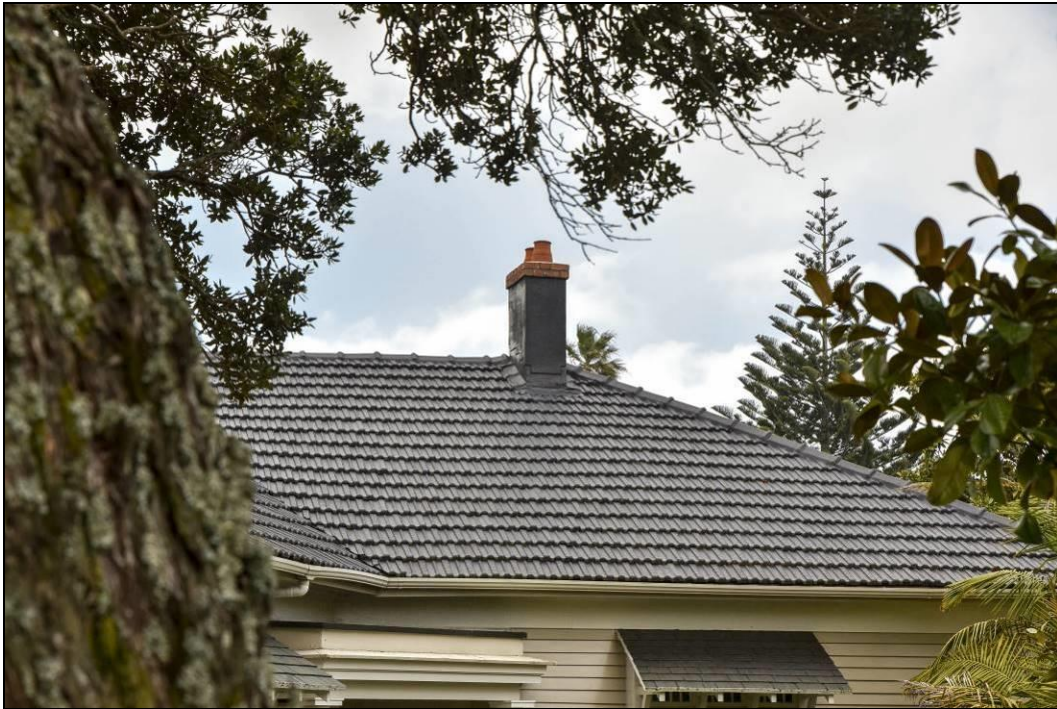
Figure 53: The site October 2016 – Looking north – at the Roof of the north west wing of the house, also one of the two original chimneys that remain. Photograph: Blair Hastings.
