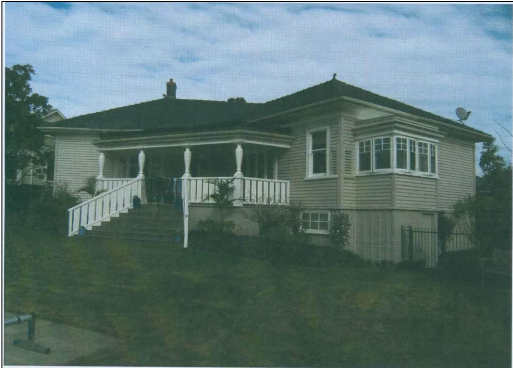
Figure 75: Auckland City Council Images – 2009. Presumably taken to check completion of 1997 works. Auckland Council files.
