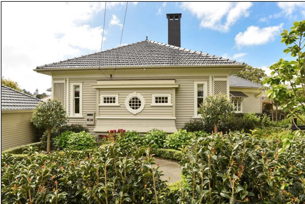
Figure 48: The site October 2016 – Looking north - at the front elevation of the house. Photograph: Blair Hastings.
