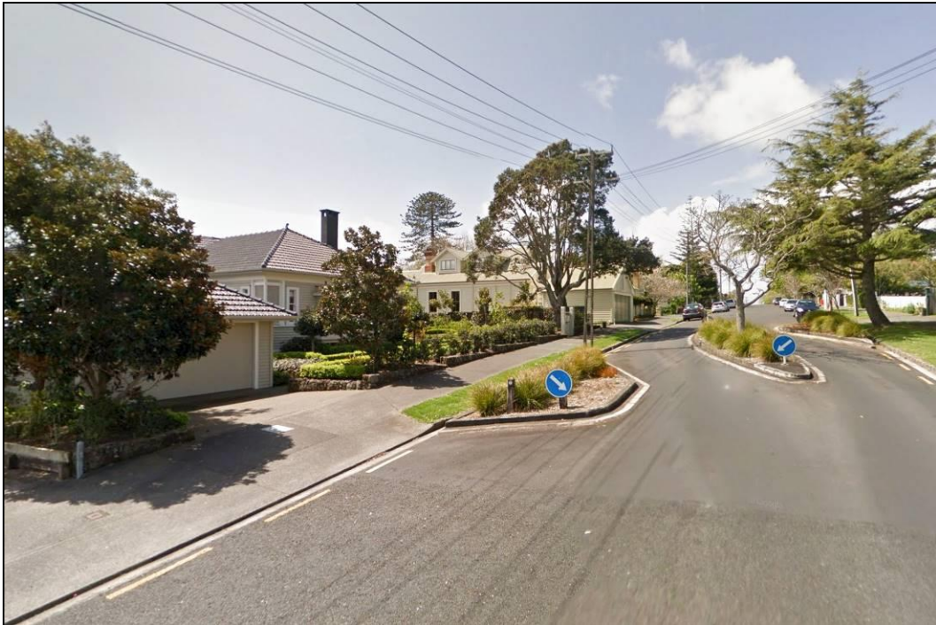
Figure 43: Site context – Looking west along Ranfurly Road (towards Manukau Road). The subject site is on the left – with the garage in the foreground. Photo: Google Maps October 2015.
