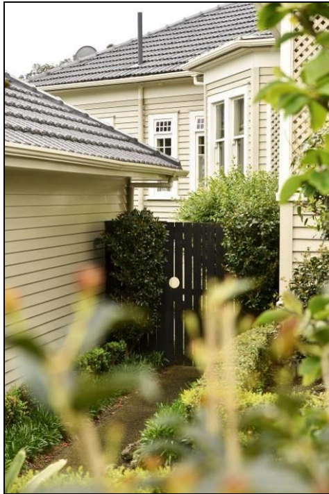
Figure 61: The site October 2016 – Looking north – at part of the west elevation of the house, seen between the vegetation and the modern garage. The chamfered rectangular library (as recorded on the 1997 plans) protrudes at the corner juncture of the southern (front) and northern wings. Both cottage style casement and villa hung windows are evident. Photograph: Blair Hastings.
